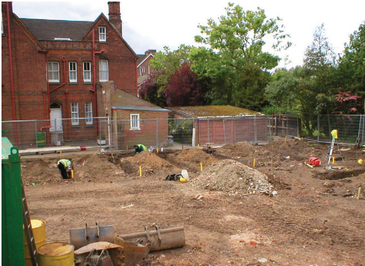
Plate 3: the site during excavation, view west, looking towards 21 West Lodge Road.
