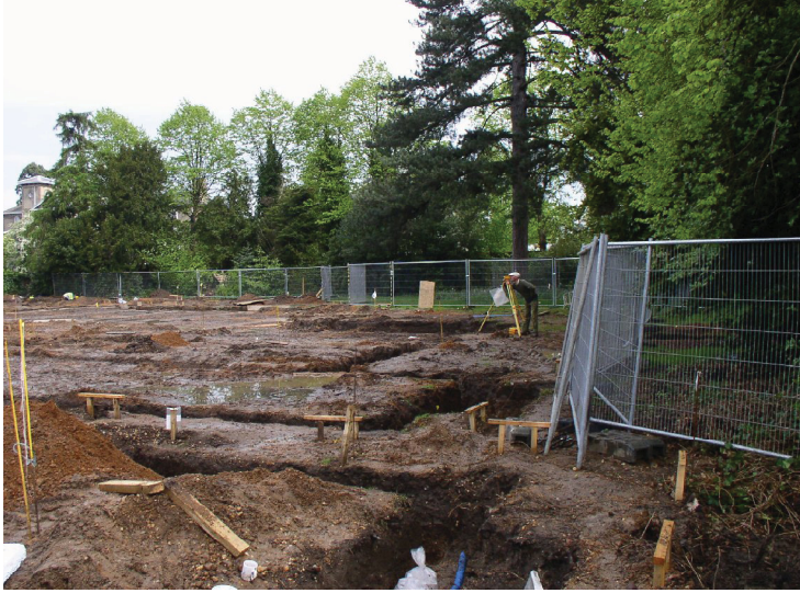
Plate 2: the site during excavation, view north-east.
