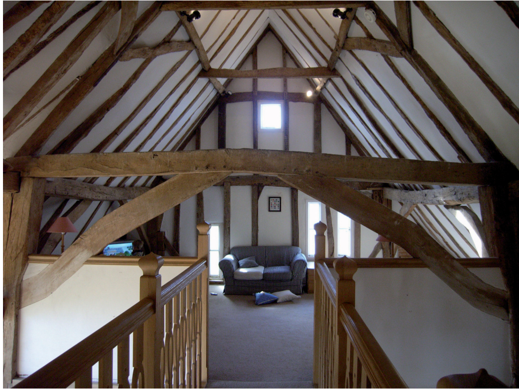
A1.13 Wiggons Barn: original clasped-purlin roof (included for comparison).
