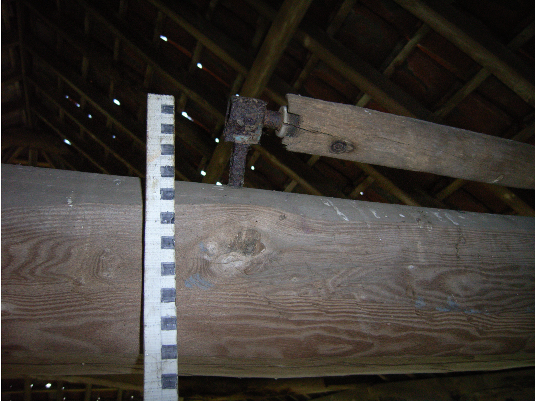
A2.9 Cart Lodge (1). Detail of wooden roller attachment seen from north
