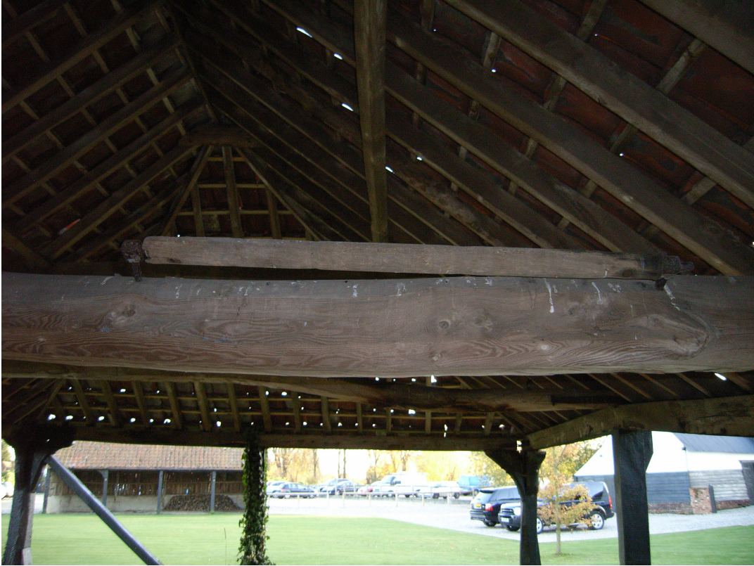
A2.7 Cart Lodge (1). Wooden roller on central tie-beam seen from north.
