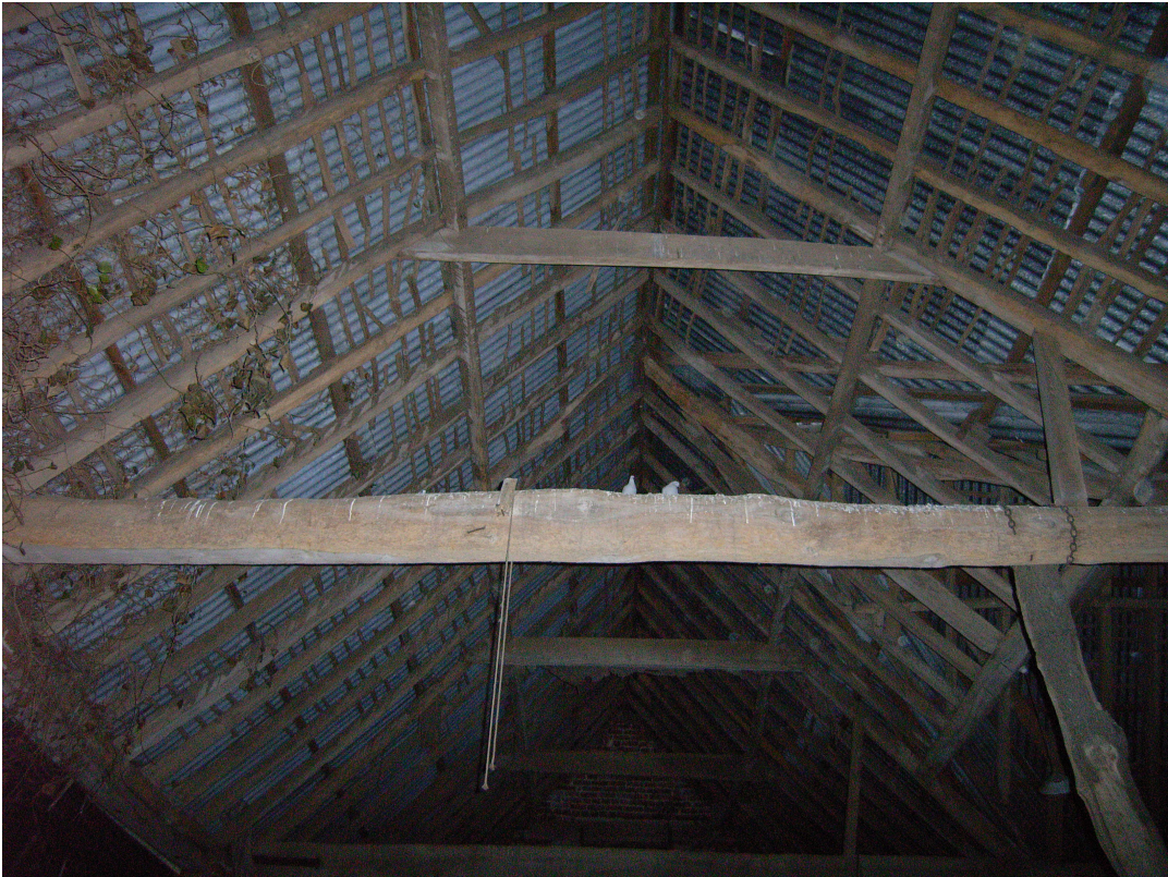
A2.11 Barn (2). Interior of clasped-purlin roof structure from west
