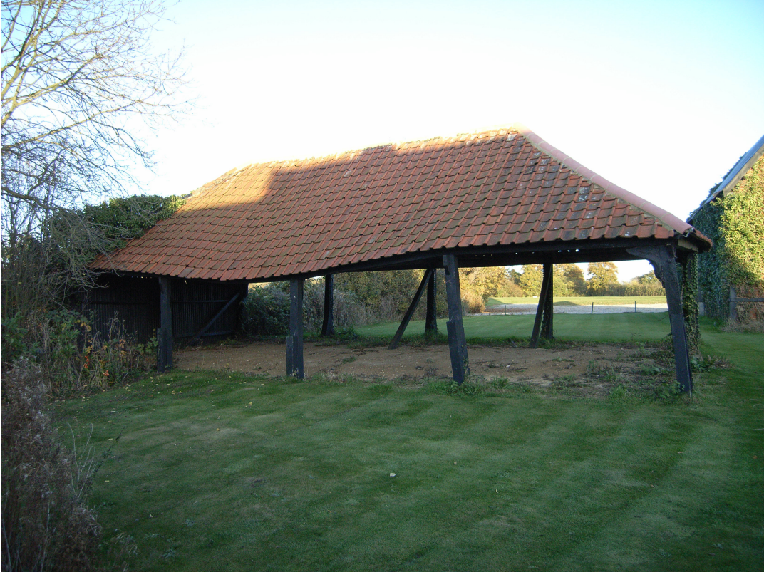
A2.5 Cart Lodge (1). External elevation from west.
