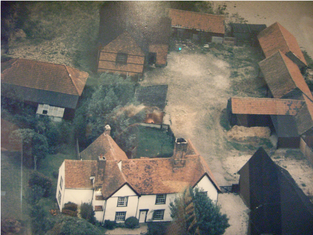
A2.1 Aerial view of site from west taken circa 1975 showing the farmhouse prior to restoration (with its original chimney, lacking any obvious initials or date) and several additional farm buildings now demolished. Buildings 1, 2 and 3 are visible from left to right. (photo in possession of current owner)
