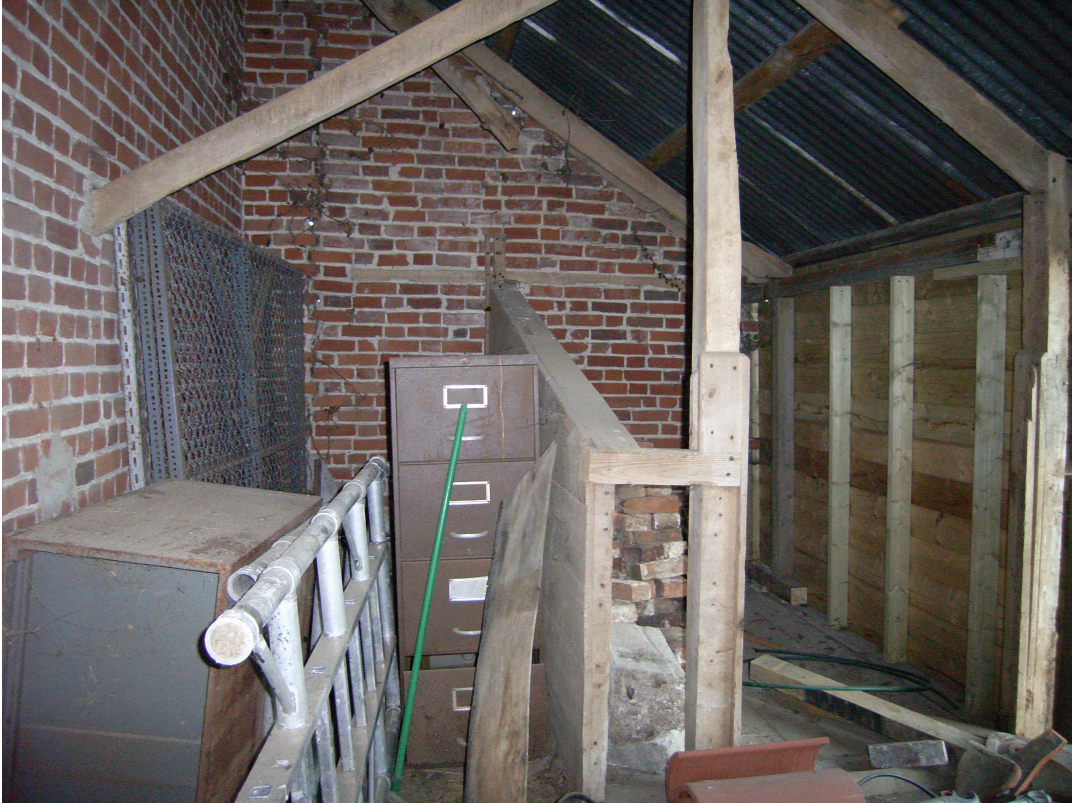
A2.11 Barn (2). Interior of granary from west with remains of two grain bins. The timber wall K-J to right is recent, apparently replacing original brickwork.
