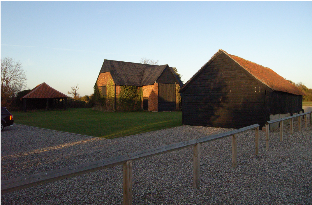
A2.2 General view of site from golf club car park to south-east showing buildings 1, 2 & 3 from left to right.
