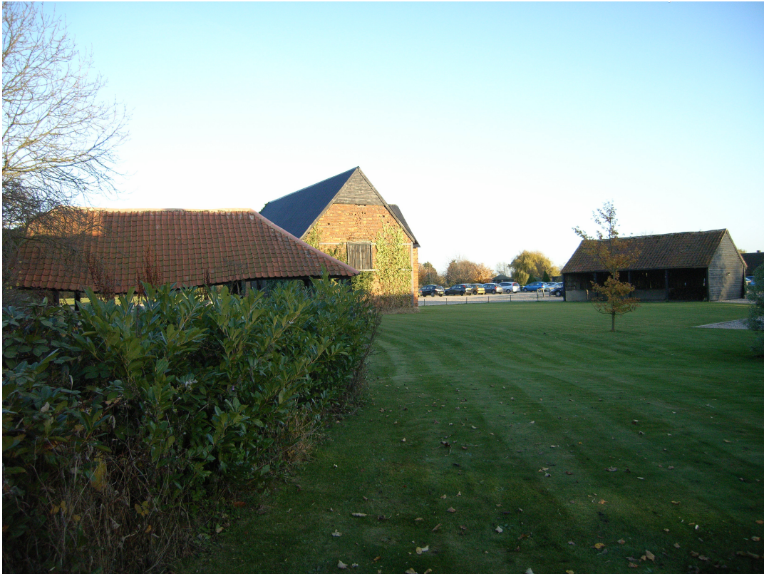
A2.3 General view from north-west showing buildings 1, 2 & 3 from left-to right. The farmyard shown in photo A2.1 is now a lawn with a car park beyond.
