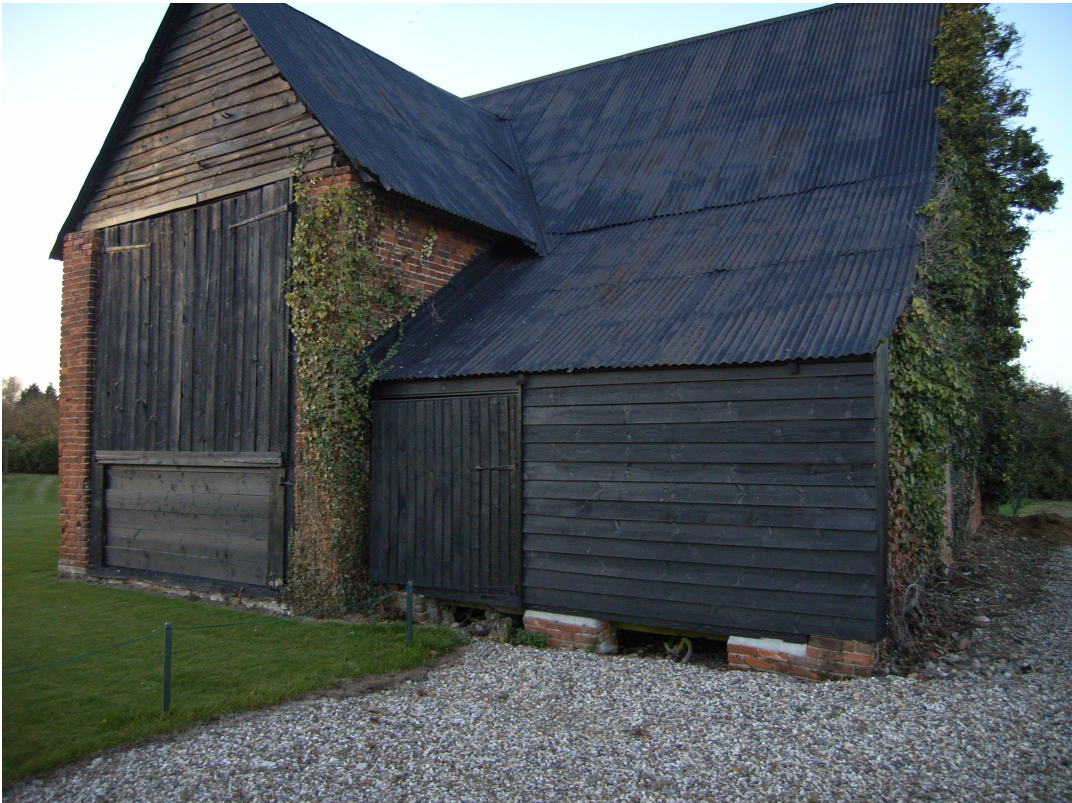
A2.10 Barn (2). Exterior of brick barn with lean-to granary on brick piers in south-eastern corner
