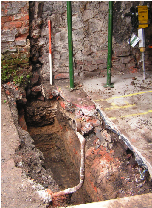
Plate 1 Footings trench at the rear of the building, view south-east.
