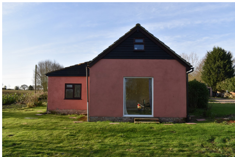
Photograph 2 North-east elevation of the building, showing modern extensions. Photograph taken facing south-west.
