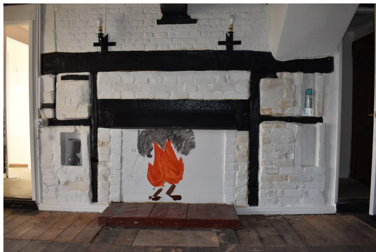
Photograph 16 Fireplace in room 8. Projection for staircase visible in top right. Photograph taken facing south-west.
