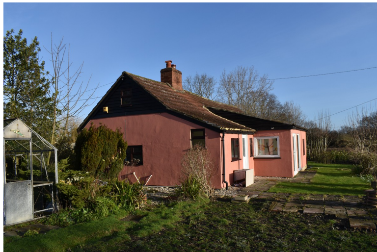
Photograph 4 South-west elevation of building. Photograph taken facing north.
