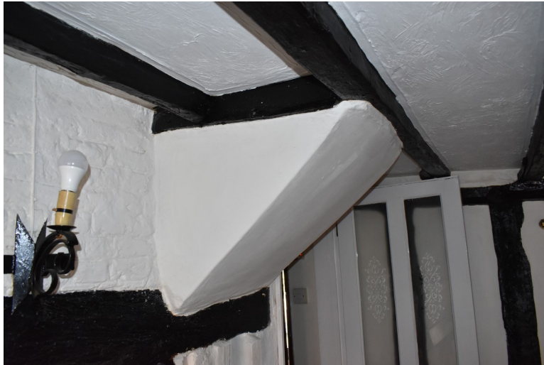
Photograph 17 Detail of underside of staircase projecting into room 8 above fireplace. Photograph taken facing north-west.
