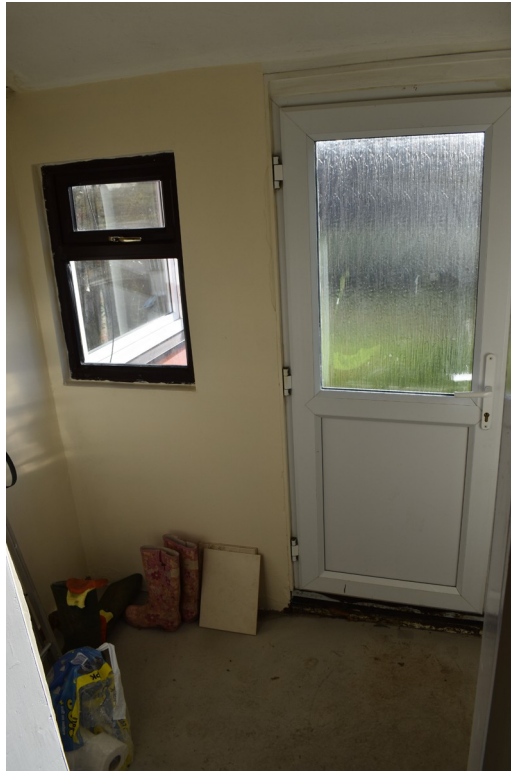
Photograph 7 Interior of room 3. Photograph taken facing north-east.
