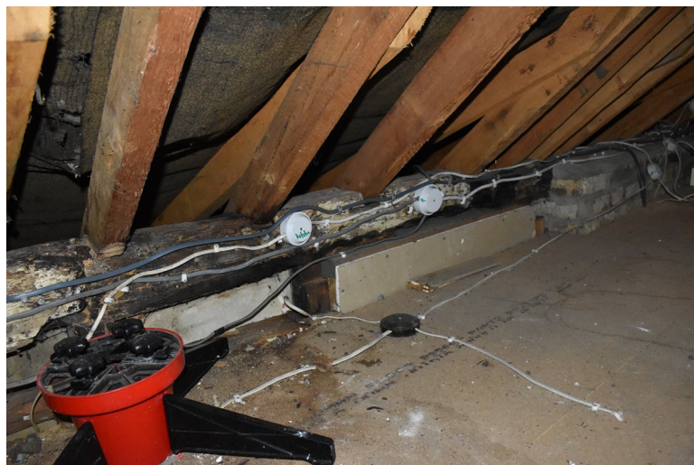
Photograph 26 Showing the end of the eastern wall-plate in the attic, abutting against modern brickwork. Photograph taken facing south.
