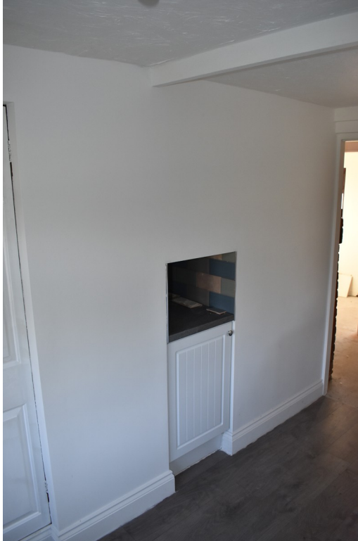
Photograph 21 Interior of room 11, showing obscured south-side of fireplace. Counter-top and cupboard in centre might indicate location of fireplace. Photograph taken facing east.
