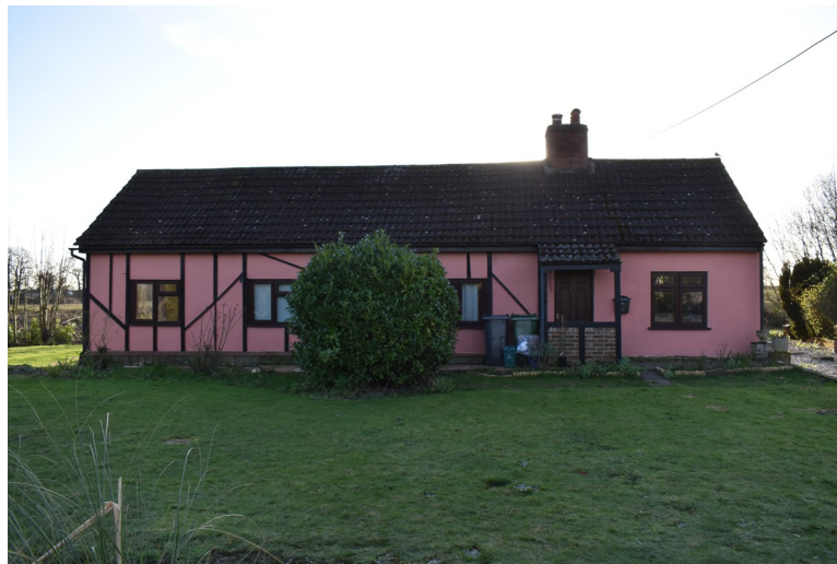
Photograph 1 The north-west elevation of the building, showing imitation timber-framing. Photograph taken facing south-east.
