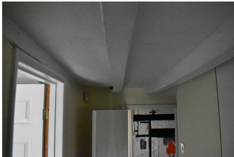
Photograph 10 Interior of room 6, showing joists in ceiling. Photograph taken facing south-west.
