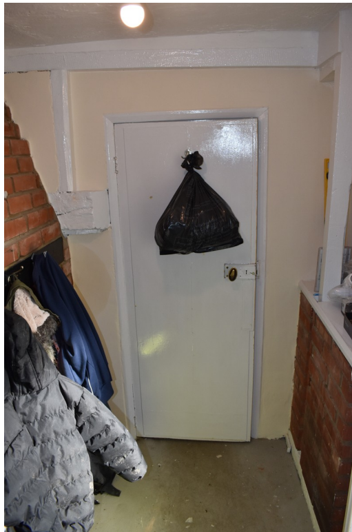
Photograph 20 Interior of room 9, showing door between room 8 and 9 and the mantel-beam of the fireplace in room 8 projecting into this room. Photograph taken facing north-east.
