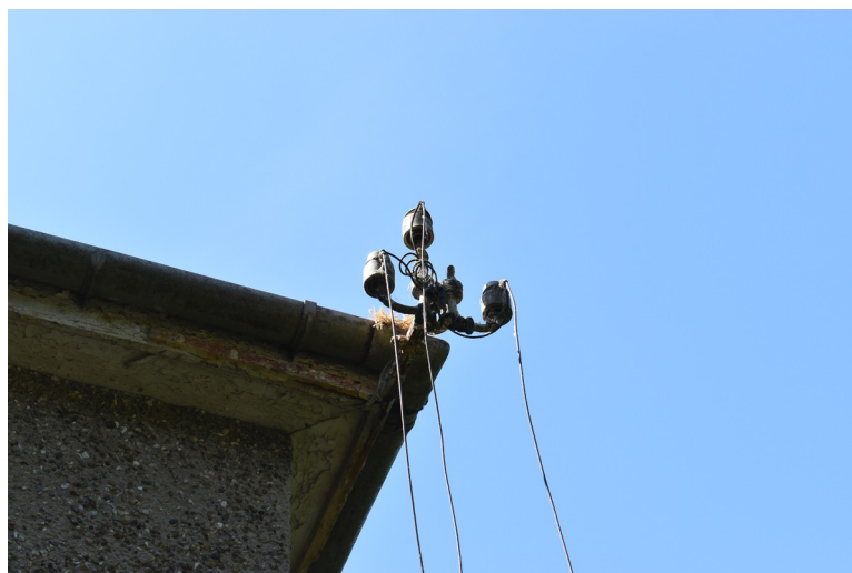
Photograph 6 Detail of ceramic terminals on the corners of the building. Photograph taken facing west.
