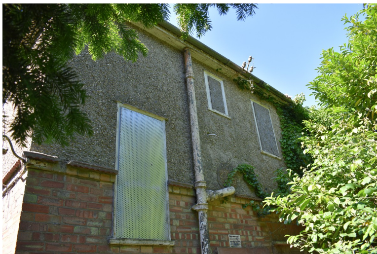
Photograph 7 North-east elevation of building (eastern side). Photograph taken facing south-west.
