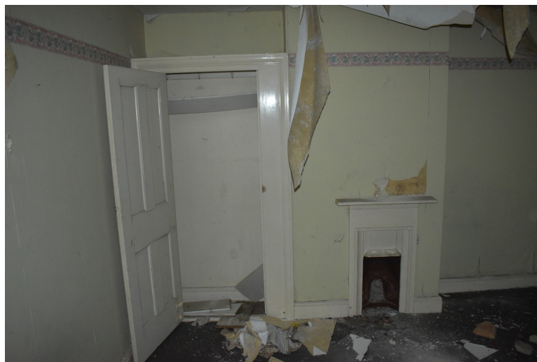
Photograph 19 Room 7a, showing original fireplace and cupboard. Photograph taken facing south-east.
