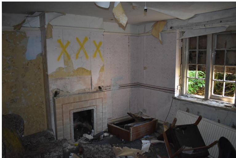
Photograph 12 Interior of room 2a. Photograph taken facing south.
