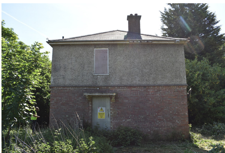
Photograph 8 North-west elevation of building. Photograph taken facing south-east.
