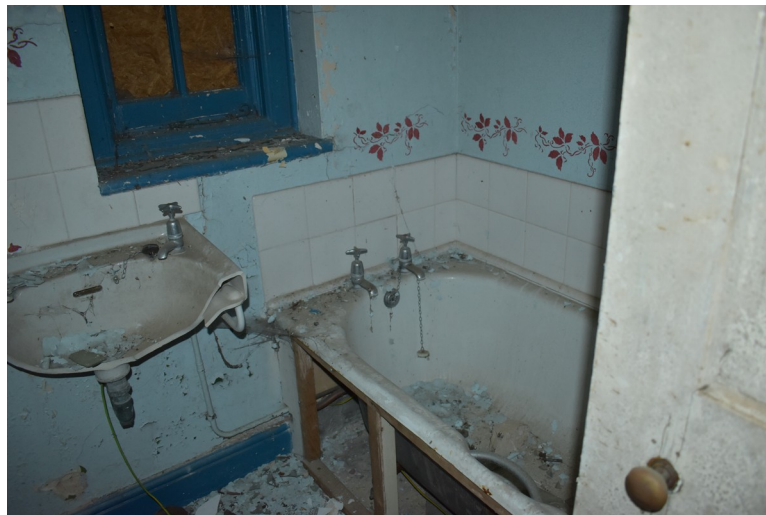
Photograph 24 Room 10a, showing bath and basin. Photograph taken facing east.
