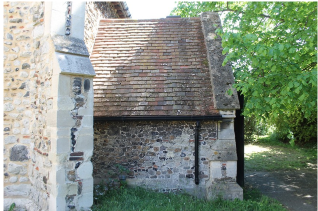
Photograph 2 Western elevation of porch. Photograph taken facing east.
