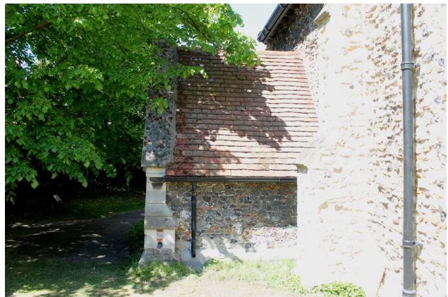
Photograph 3 Eastern elevation of porch. Photograph taken facing west.
