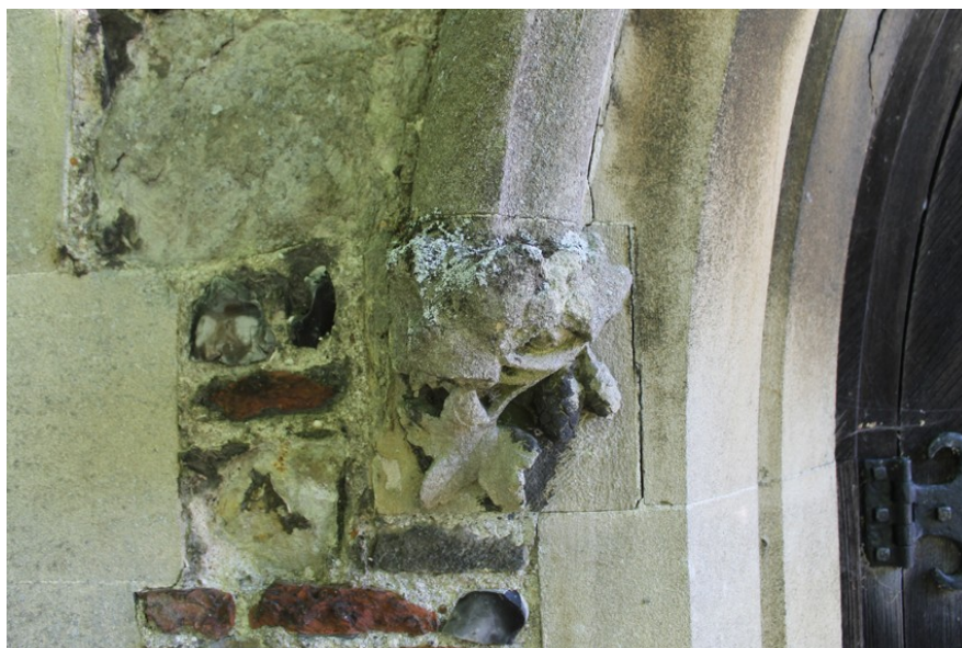
Photograph 5 Detail of decorated label-stop on west side of arch on southern elevation of porch. Photograph taken facing north.
