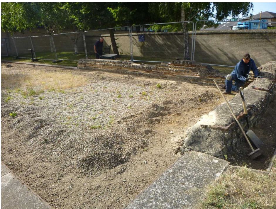
Photograph 1 Working shot during renovation works – looking south-east
