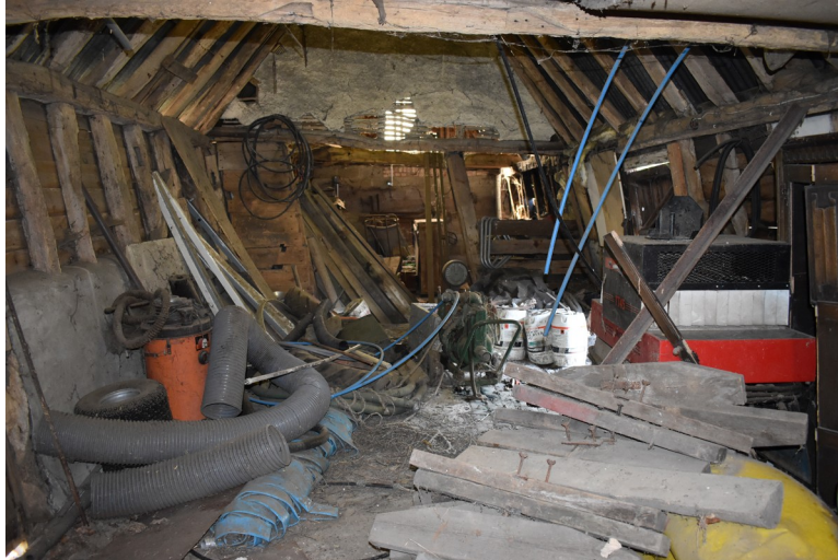
Photograph 12 Interior of bay 2. Photograph taken facing south-east.
