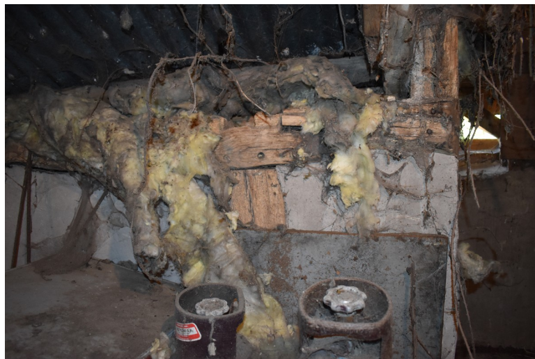
Photograph 7 Detail of small section of exposed ?hand-sawn timber in bay 1. Photograph taken facing north-east.
