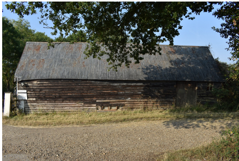
Photograph 5 North-east elevation of the outbuilding. Photograph taken facing west.
