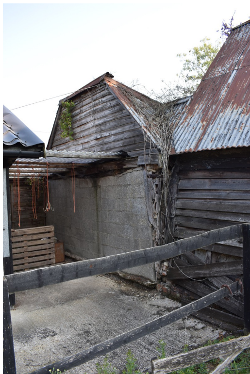
Photograph 2 South-west elevation of outbuilding, bay 1, showing concrete block infilling. Photograph taken facing north.
