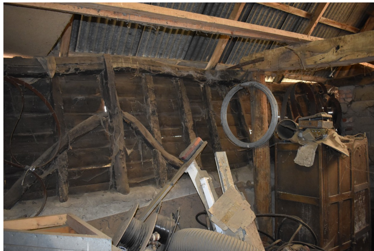
Photograph 16 Interior of bay 3 showing timber-framing. Photograph taken facing east.
