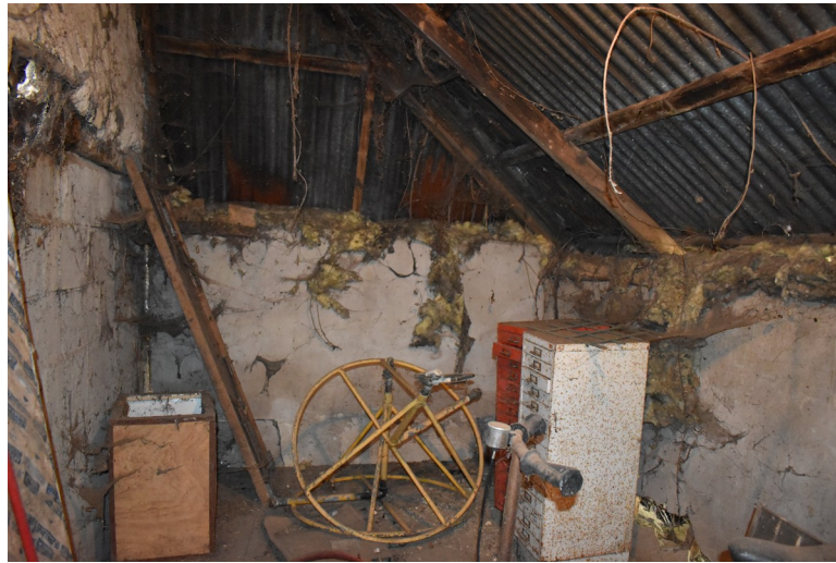
Photograph 6 Interior of bay 1. Photograph taken facing north-west.
