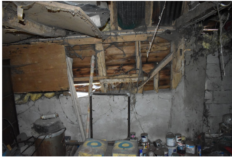
Photograph 8 Interior of bay 2, with entrance into bay 1 visible to right, including empty mortices on wall-plate. Photograph taken facing south-west.
