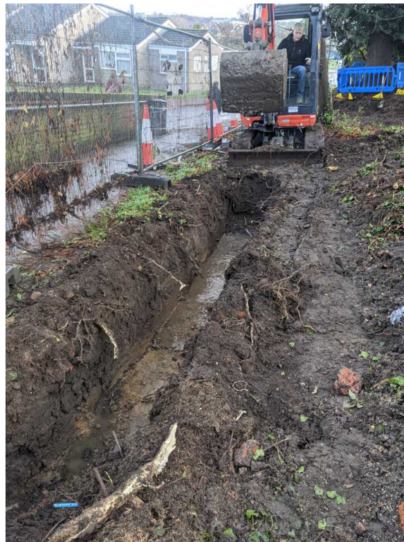
Photograph 1 Digger working shot
