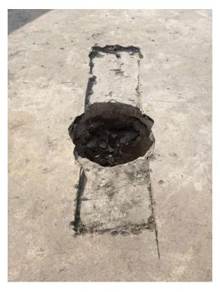
**Photograph 13** Martello Tower external view, second-floor. Detail of damage to floor, possibly due to removal of 20th-century water tank. Photograph taken facing south-east.
