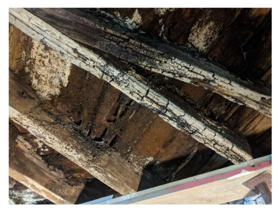
**Photograph 11** Martello Tower internal view, ground-floor. Detail of damage to floor above.
