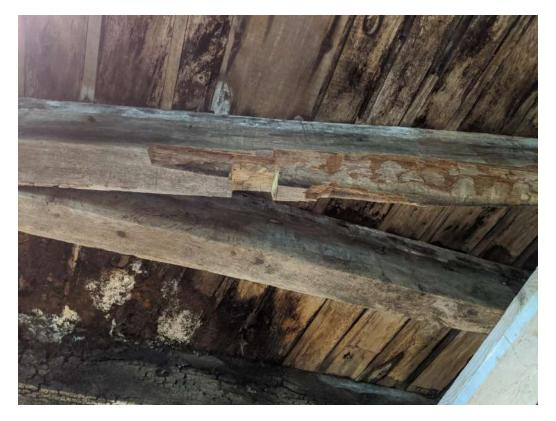
**Photograph 15** Martello Tower internal view, ground-floor. Detail of altered beam from floor above.
