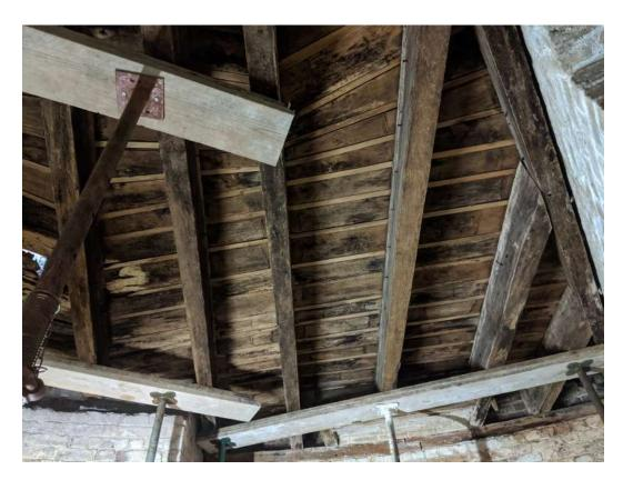
**Photograph 14** Martello Tower internal view, ground-floor. Detail of floor construction. Photograph taken facing north-east.
