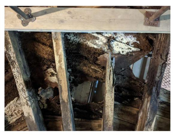
**Photograph 12** Martello Tower internal view, ground-floor. Detail of damage to floor above.
