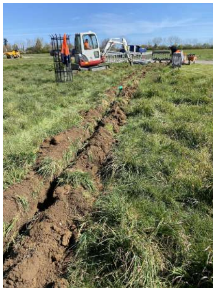
Photograph 1 Cable trenching – looking northeast
