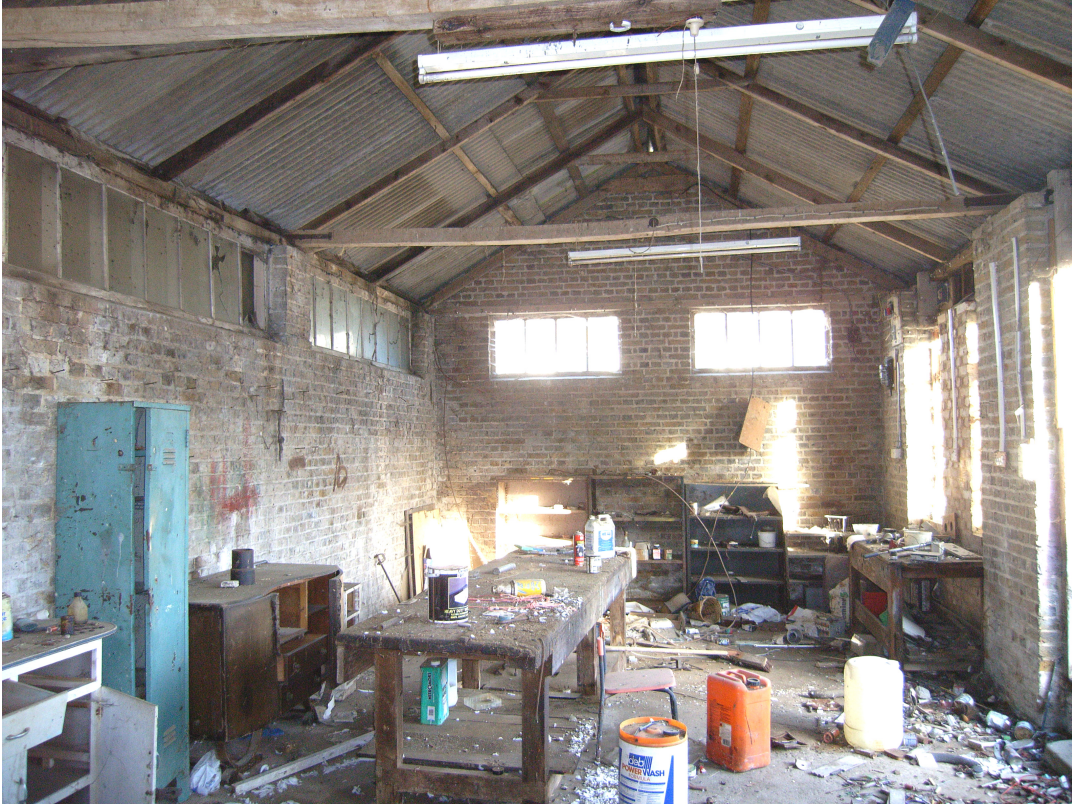
A2.9 Workshop. Interior from west, showing entrance to right.
