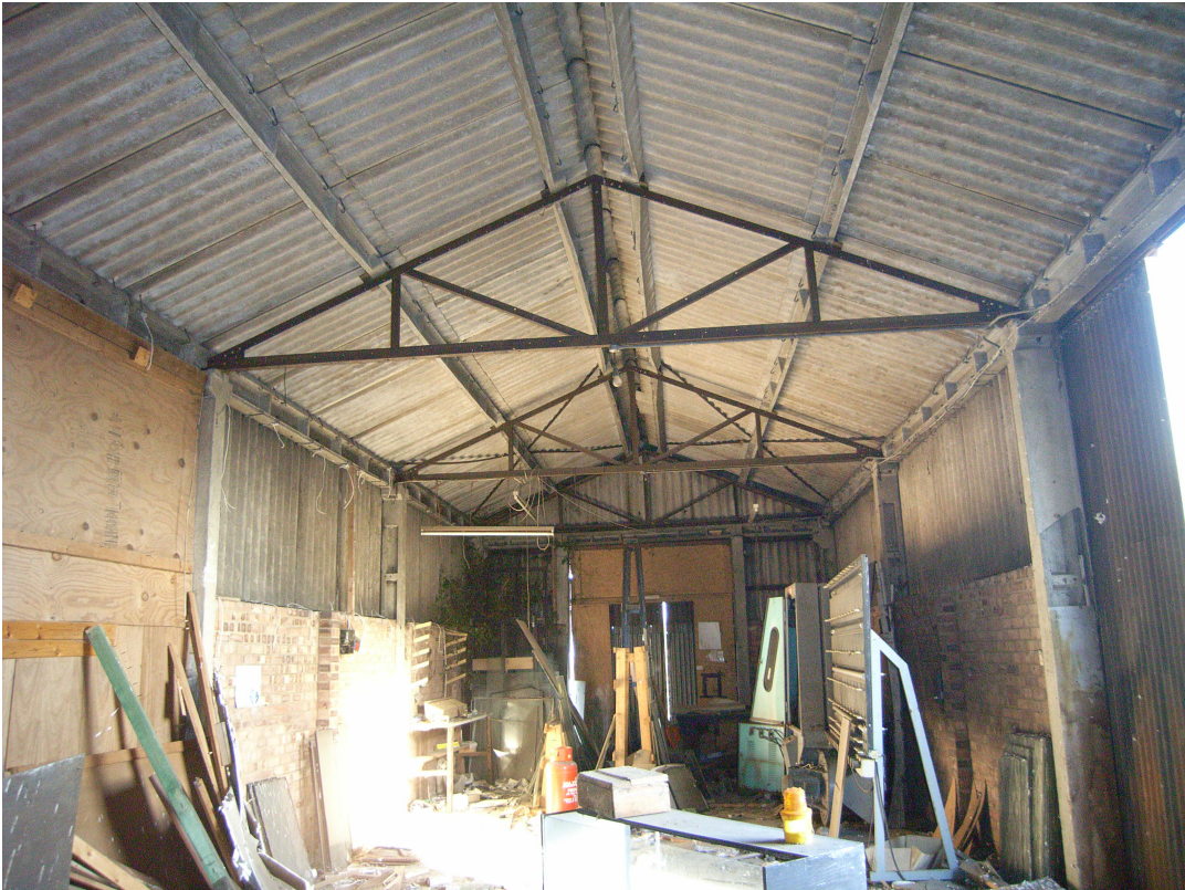
A2.11 Barn. Interior from west, showing mid 20th-century construction.
