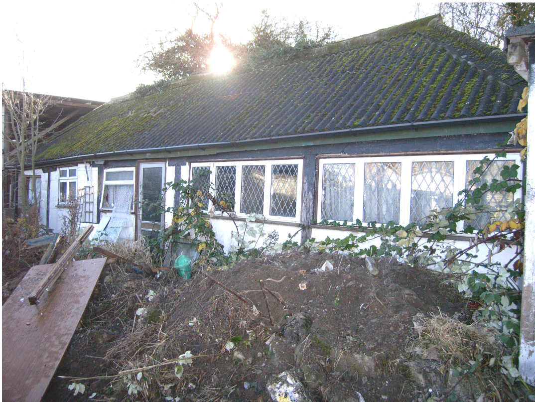
A2.6 Shelter shed. Exterior, showing former open arcade of eastern elevation.
