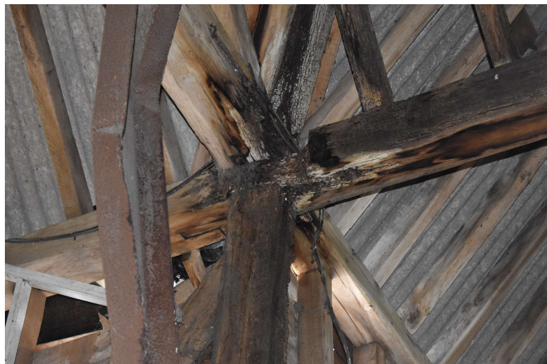
HSCF21_Photograph_060Rotting scarf joint on southern wall-plate between ba...
