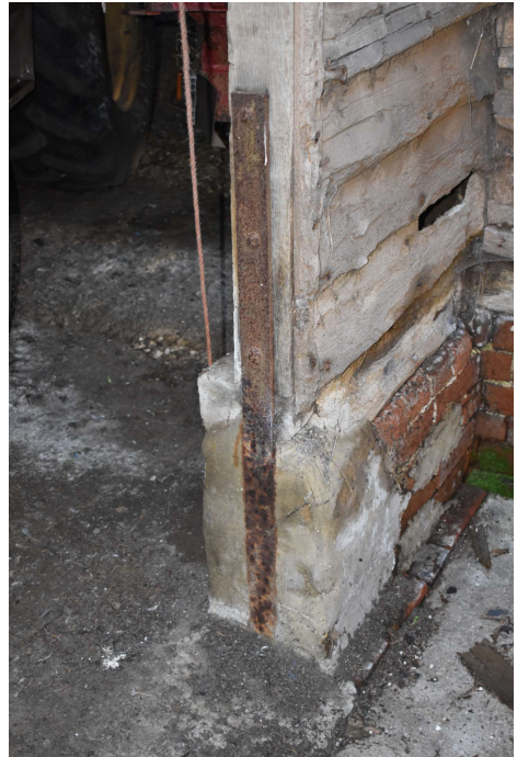
HSCF21_Photograph_069Detail of concrete and cut sill-beam in doorway on ea... HSCF21_Photograph_070Detail of concrete, cut sill-beam and metal brace in d...
