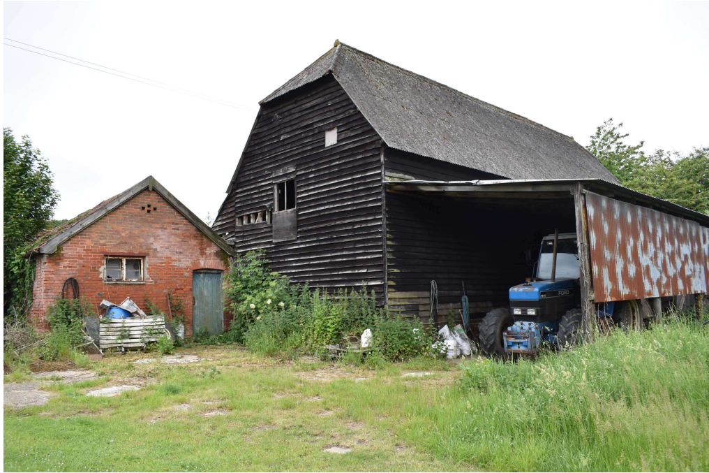
Photograph 4 Eastern elevation of threshing barn. Photograph taken facing south-west.
