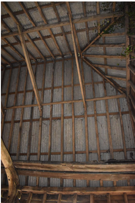
HSCF21_Phograph_036Interior southern elevation of bay 1 showing roof pitc...
