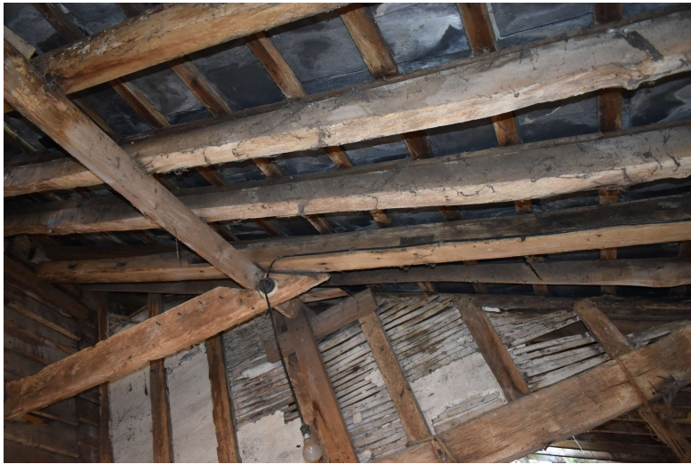
HSCF21_Phograph_079Detail of re-used timber in roof of lean-to. Photograp...
