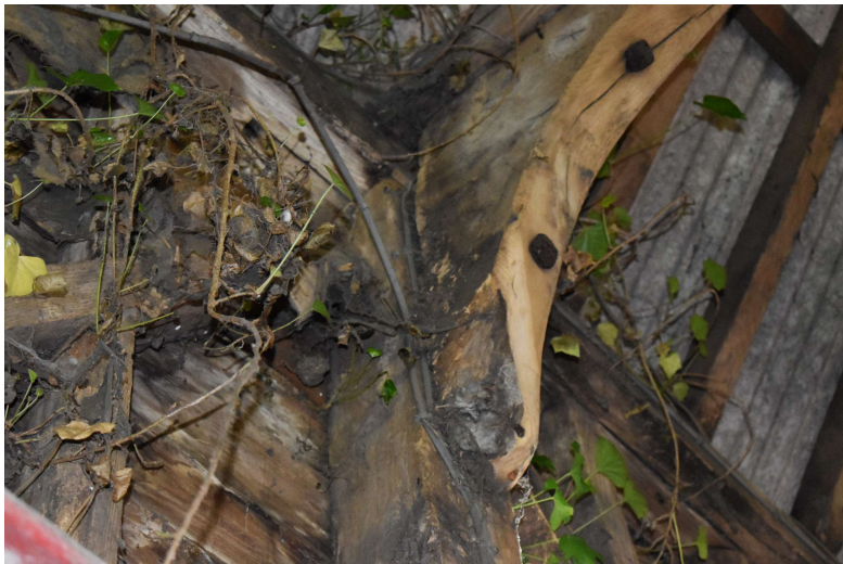
HSCF21_Photograph_057Detail of scarf joint on wall-plate on northern elevatio...
