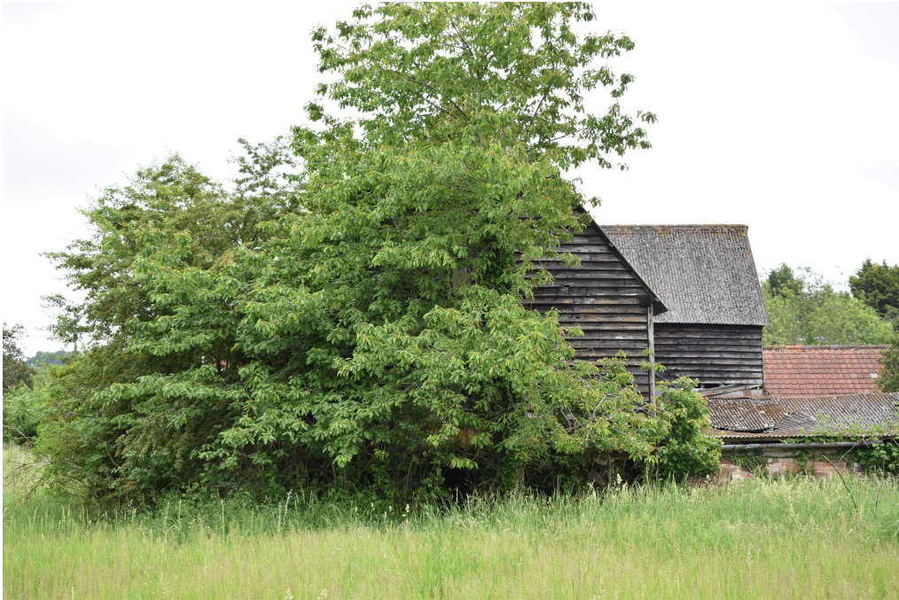
Photograph 6 Western elevation of threshing barn. Photograph taken facing east.
