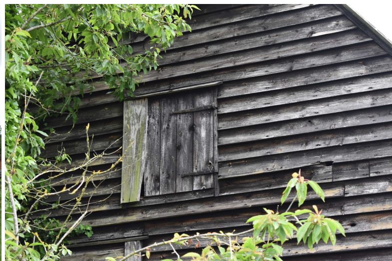
HSCF21_Photograph_012Pitching door on western elevation of threshing barn....
