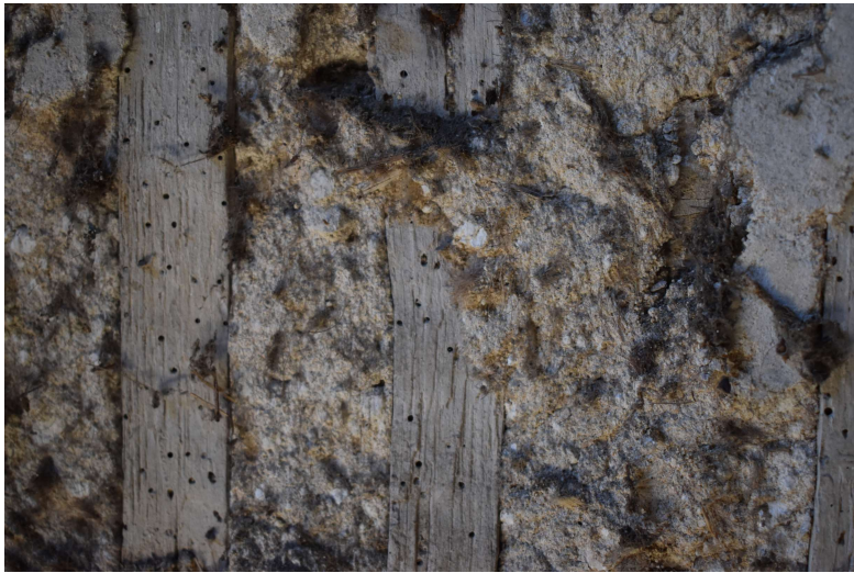
HSCF21_Photograph_085Detail of horse hair in lath and plaster in bay 5 south...
