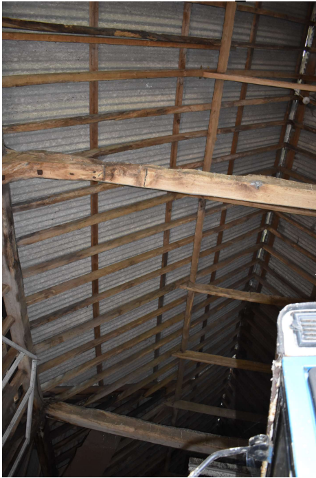
HSCF21_Phograph_031Interior southern elevation of bay 4 showing roof pitc...
