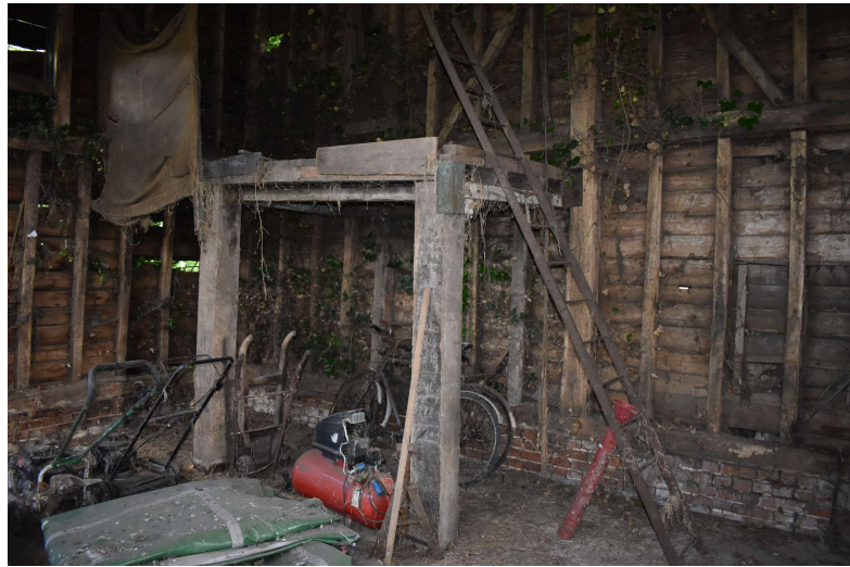
HSCF21_Photograph_056Detail of modern mezzanine level in bay 1. Photogra...
