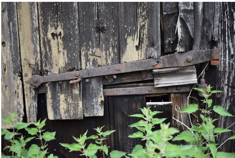
HSCF21_Photograph_017Detail of door hinges on midstory doors on southern ...
