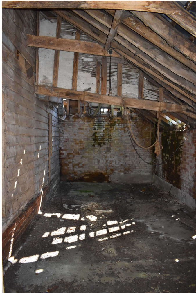
Photograph 19 Interior of lean-to. Photograph taken facing west.
