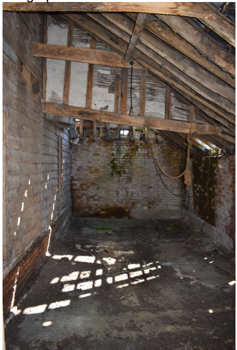
HSCF21_Phograph_080Interior of lean-to. Photograph taken facing west.
