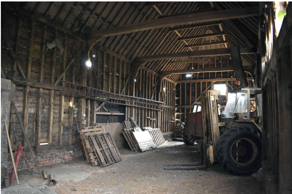
Photograph 7 Interior of threshing barn. Photograph taken facing north-east.
