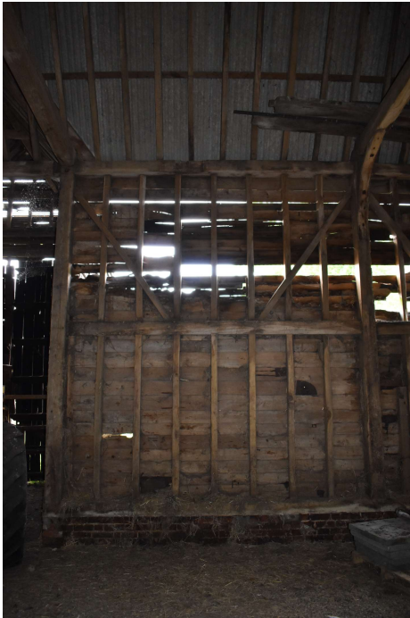
HSCF21_Phograph_033Interior southern elevation of bay 2. Photograph take...
