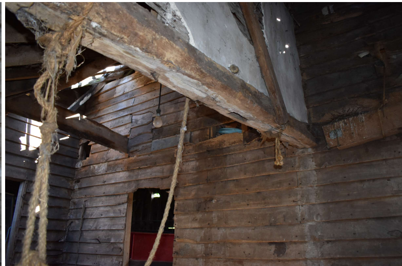
HSCF21_Photograph_076Re-use timber in lean-to. Photograph taken facing no...
