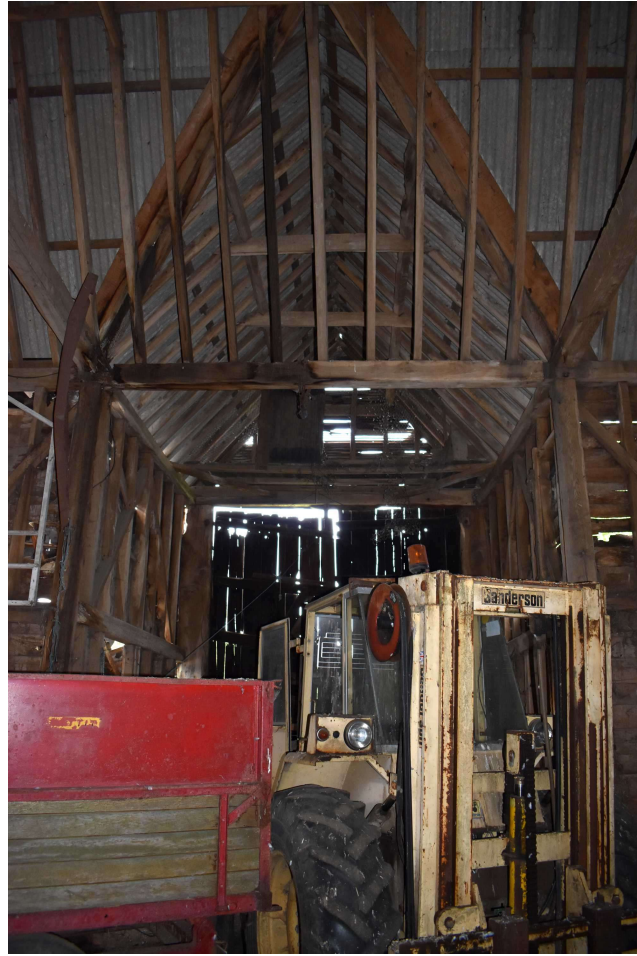
Photograph 8 Interior southern elevation of bay 3. Photograph taken facing south.
