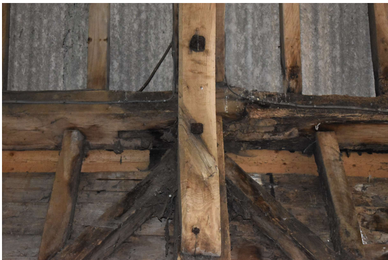
HSCF21_Photograph_059Scarf joint on northern wall-plate between bays 3 and...
