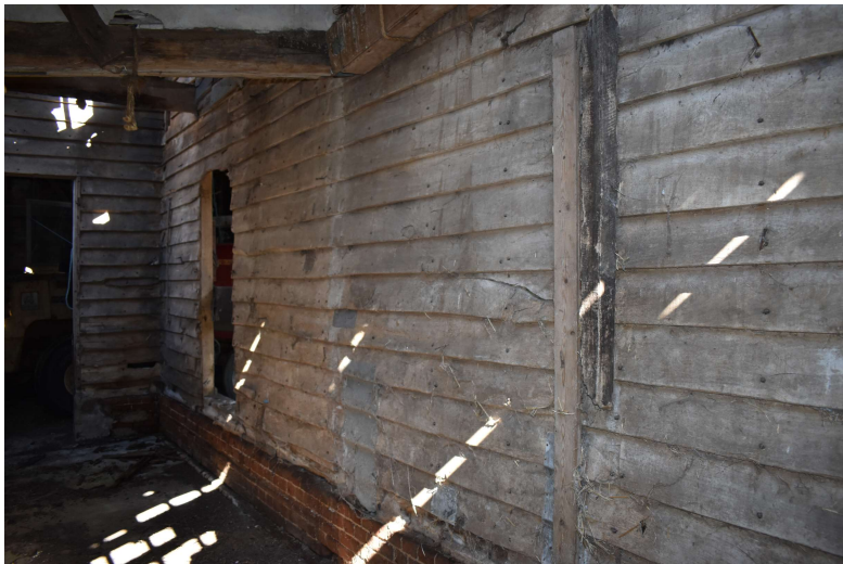
HSCF21_Photograph_075Original wetherboarding in lean-to on southern elevat...
