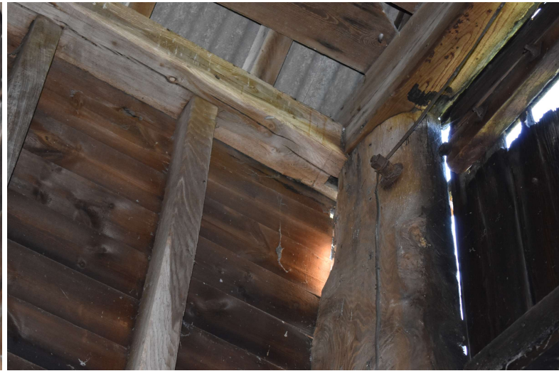
HSCF21_Photograph_074Mortise detail on east side of midstray door. Photogr...
