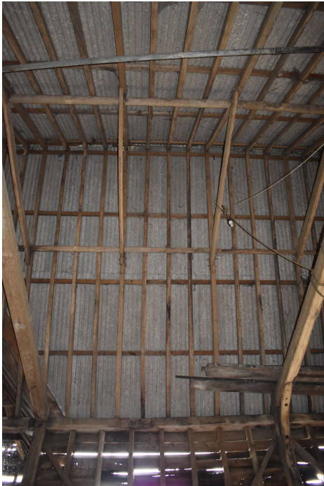
HSCF21_Phograph_034Interior southern elevation of bay 2 showing roof pitc...
