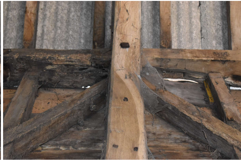
HSCF21_Photograph_062Northern wall-plate scarf joint between bays 4 and 5. ...
