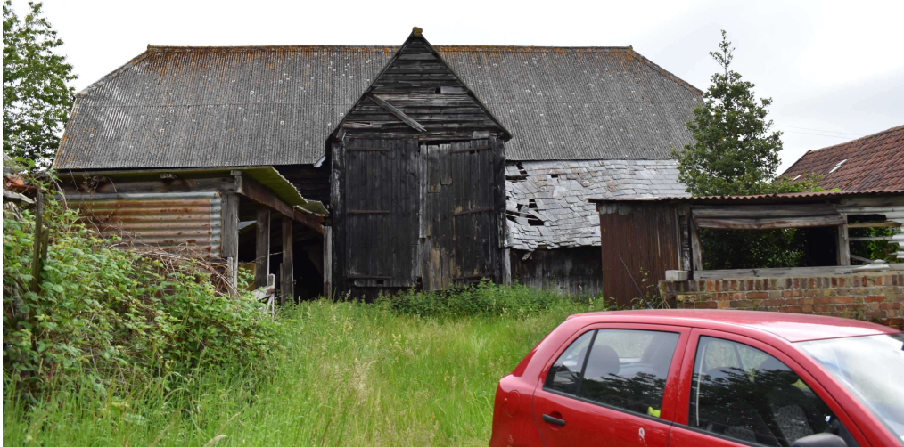
Photograph 2 Southern elevation of threshing barn. Photograph taken facing north.
