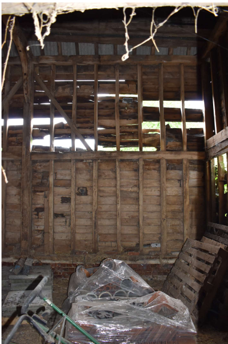
HSCF21_Phograph_035Interior southern elevation of bay 1. Photograph take...
