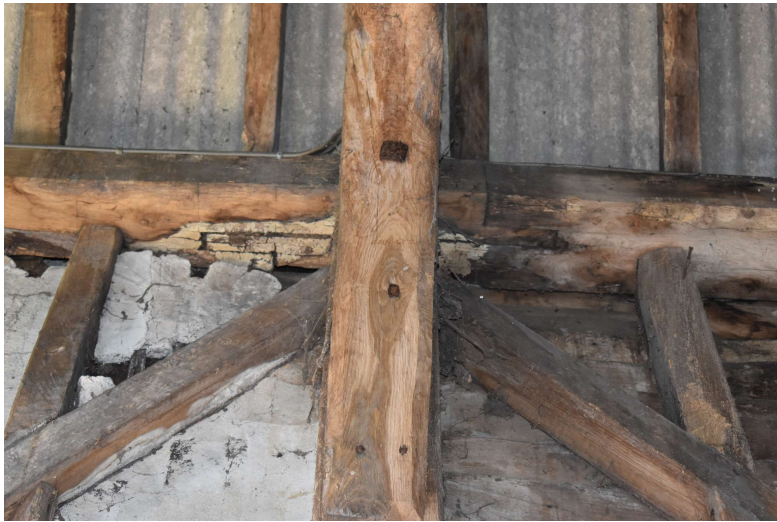
HSCF21_Photograph_061Southern wall-plate scarf joint between bays 4 and 5...
