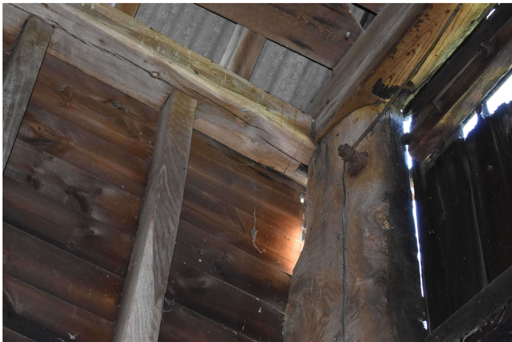
Photograph 16 Mortise detail on east side of midstrey door. Photograph taken facing south-east.
