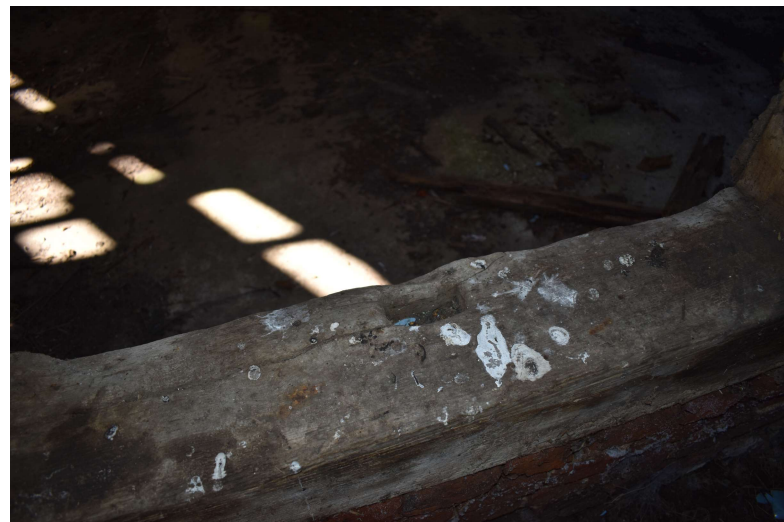
HSCF21_Photograph_066Empty mortice in sill-beam of southern elevation of b...
