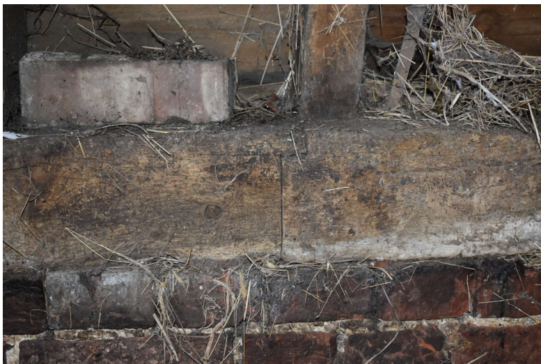
HSCF21_Photograph_053Detail on scarf joint on sill-beam in western elevation...
