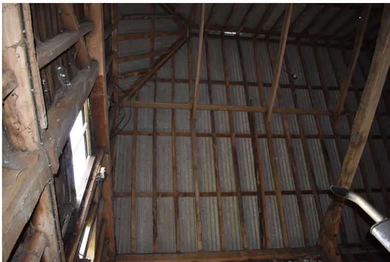
HSCF21_Phograph_029Interior southern elevation of bay 5 showing roof pitc...
