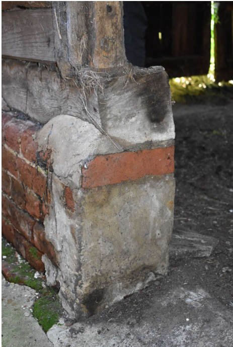
HSCF21_Photograph_069Detail of concrete and cut sill-beam in doorway on ea... HSCF21_Photograph_070Detail of concrete, cut sill-beam and metal brace in d...
