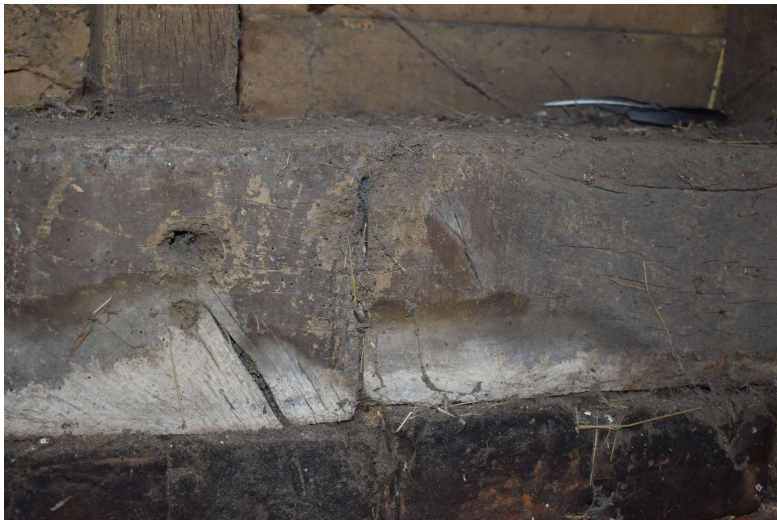
HSCF21_Photograph_063Northern sill-beam scarf joint in bay 5. Photograph ta...
