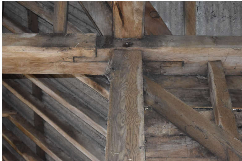
HSCF21_Photograph_058Scarf joint in southern wall-plate between bays 2 and...
