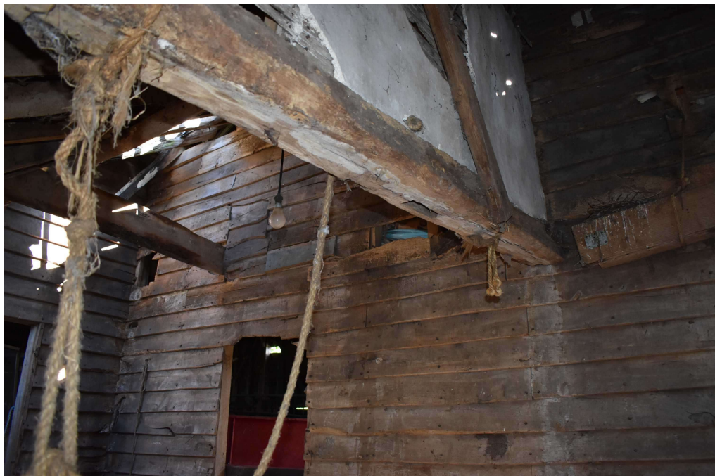
Photograph 18 Re-used timber in lean-to. Photograph taken facing north-west.
