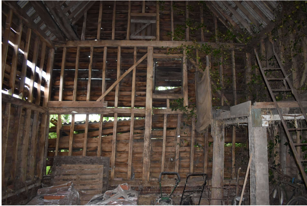
Photograph 12 Interior western elevation of bay 1. Photograph taken facing west.
