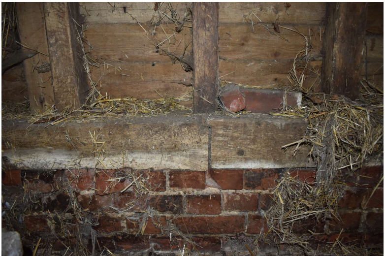
HSCF21_Photograph_052Detail of scarf joint on sill-beam in southern elevation...
