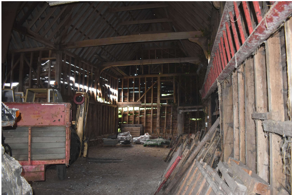
Photograph 9 Interior of threshing barn. Photograph taken facing south-west.
