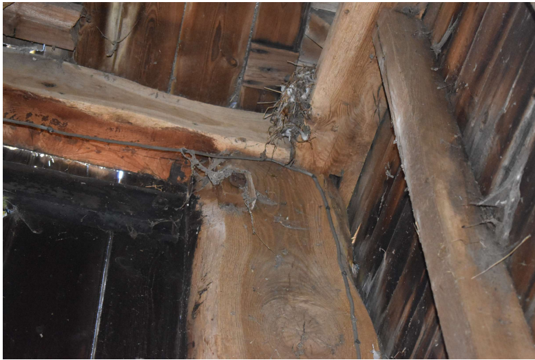
HSCF21_Photograph_073Mortise detail on west side of midstray door. Photogr...
