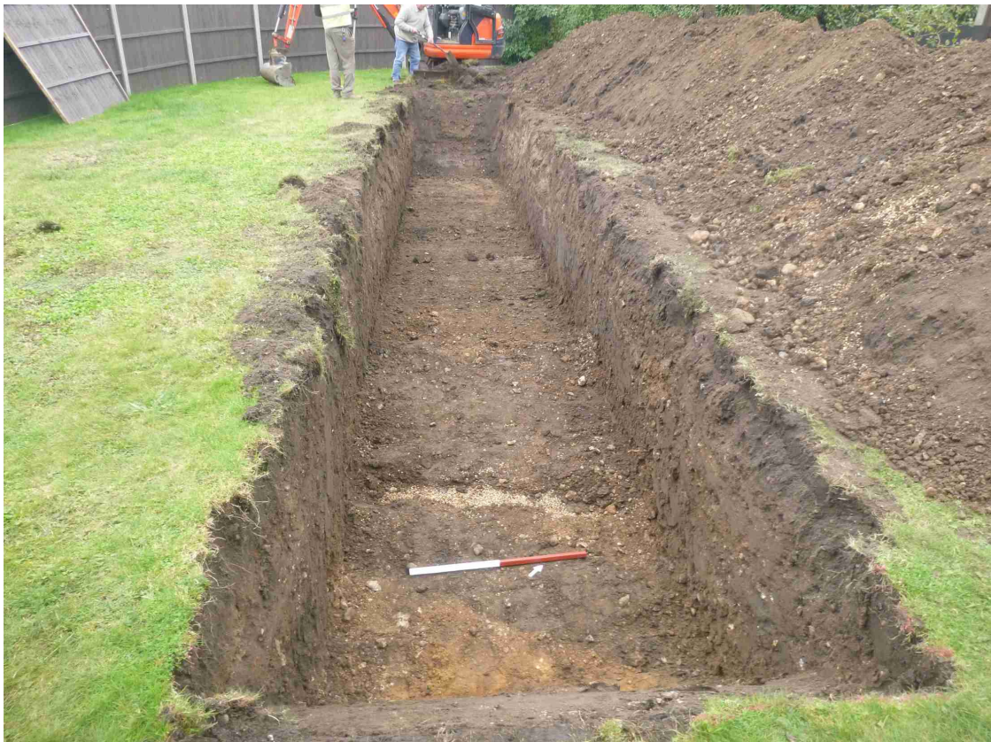
Photograph 1 Trench 1 (showing modern service trenches in foreground), looking west-northwest
