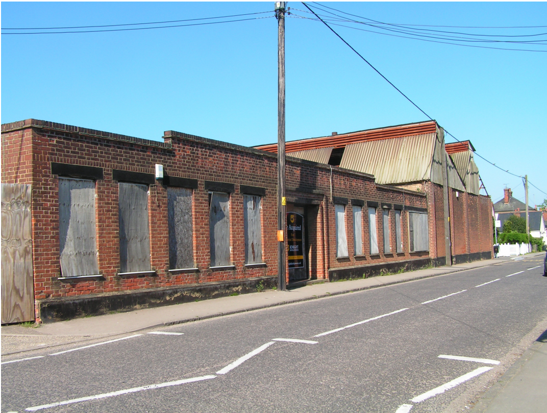
A1.1 Rayne Foundry frontage showing main offices, view north-east, from The Street.
