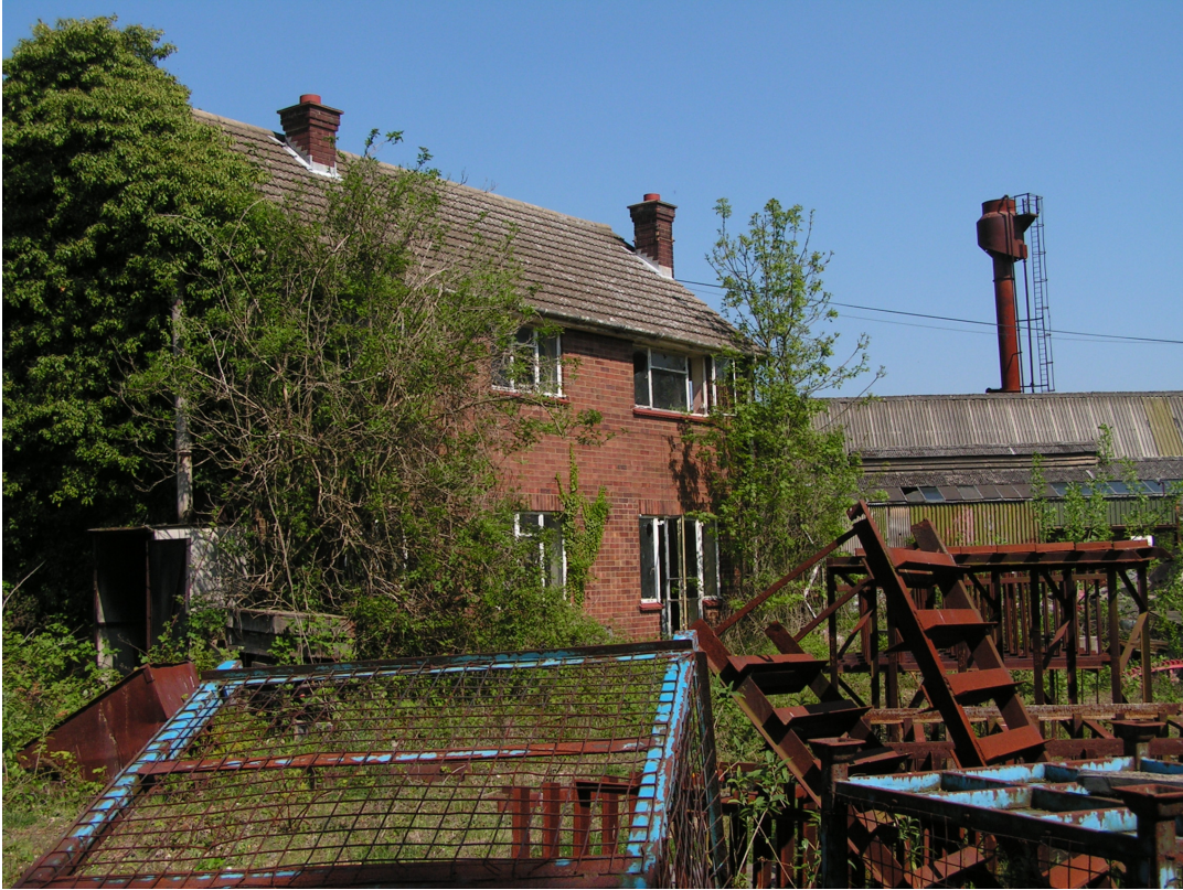
A1.23 Building 7: the former foundry manager's house with the main foundry complex and cupola chimney in the background, view east.
