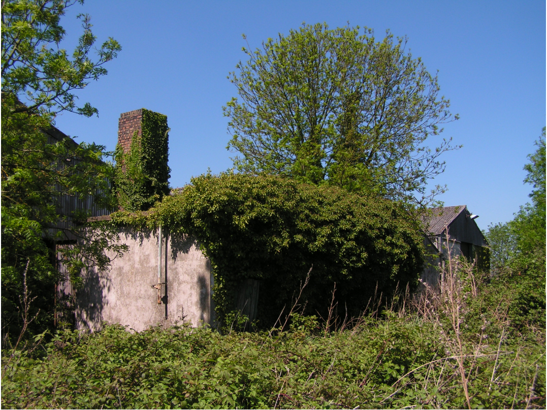
A1.25 Building 15: possible boiler room, view north-west.
