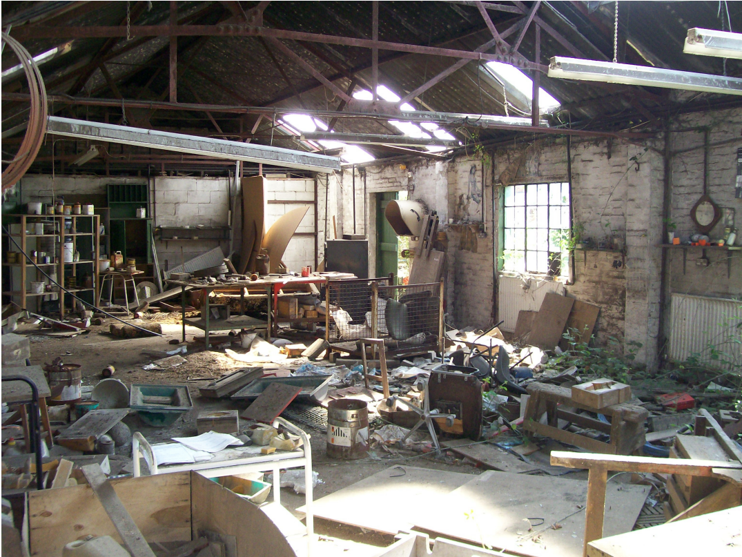
A1.4 Interior of the pattern shop, view south-west.
