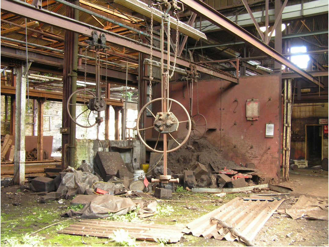
A1.16 The overhead monorail metal-handling system with ladle hoists, view north-east.
