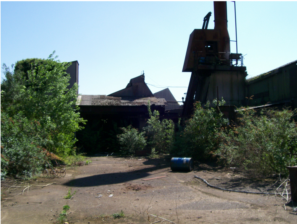
A1.14 Roper cupola chimney showing the automatic lift to the charge door, view south.
