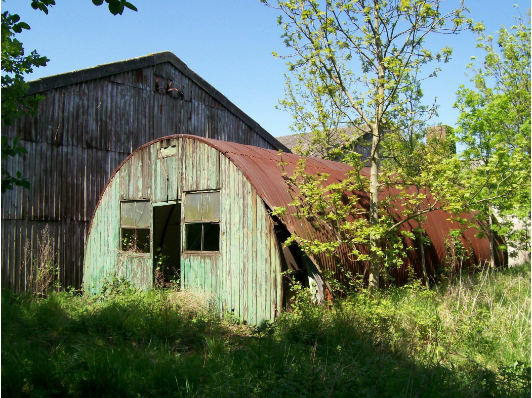
A1.26 Building 16: Nissen hut, view north-west.
