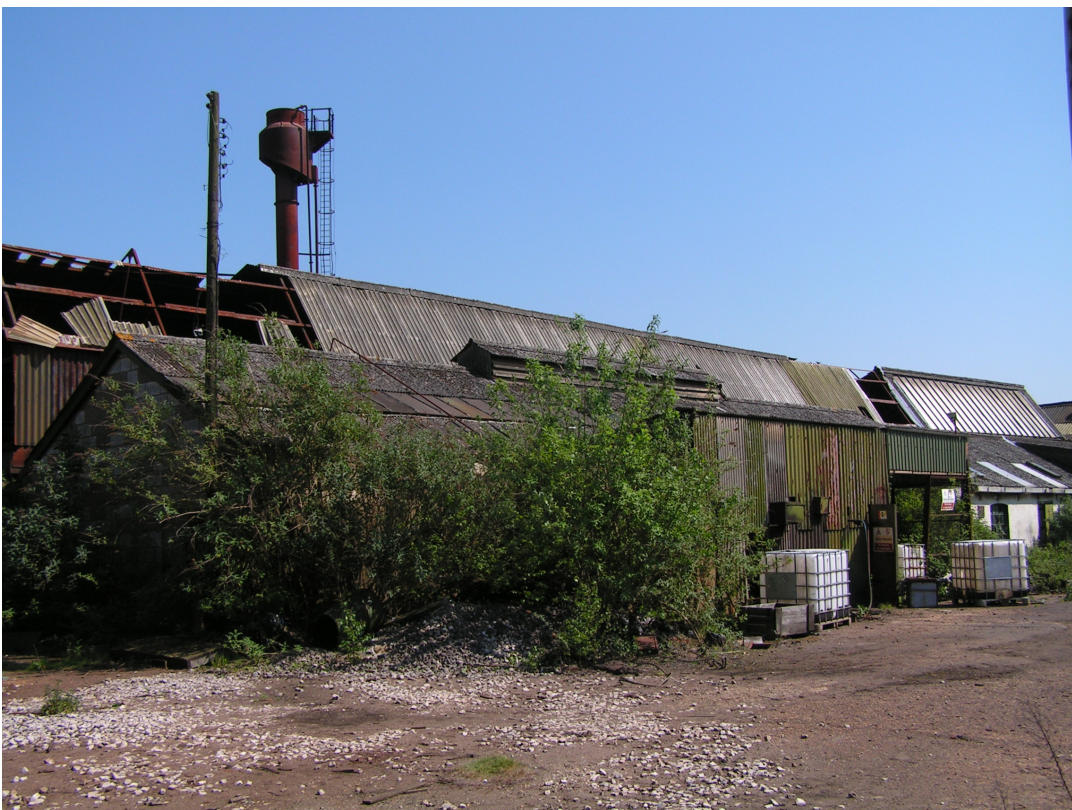
A1.2 General shot of the main foundry complex, view south-east.
