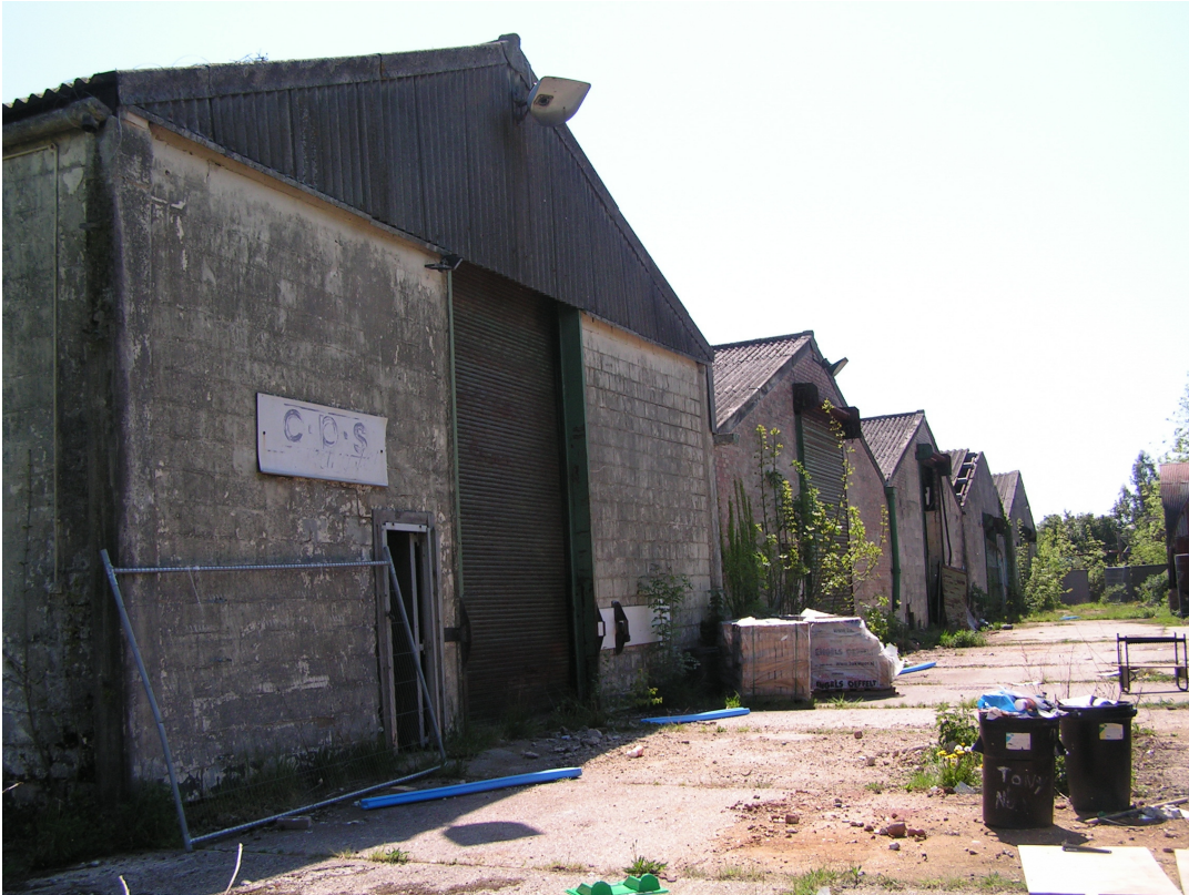
A1.24 Buildings 12-14: exterior, view south-east.
