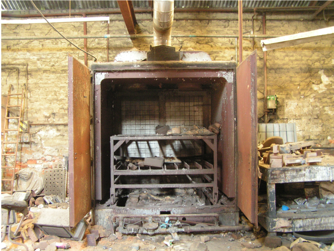
A1.9 Core baking oven, view east.
