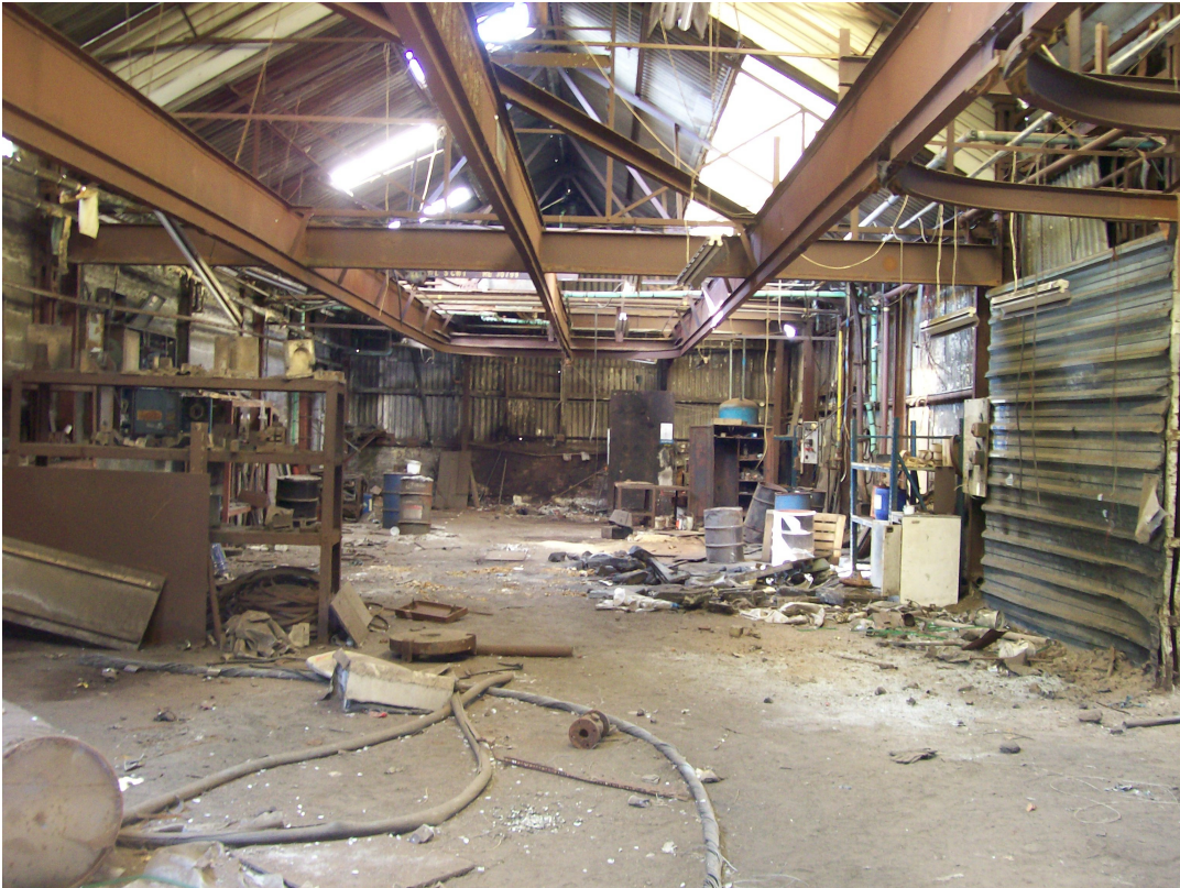
A1.20 Aluminium foundry with overhead monorail metal-handling system, view south-west.
