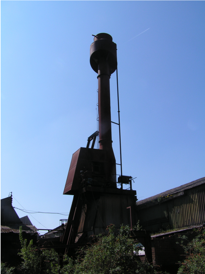
A1.13 Roper cupola chimney, view south-west.
