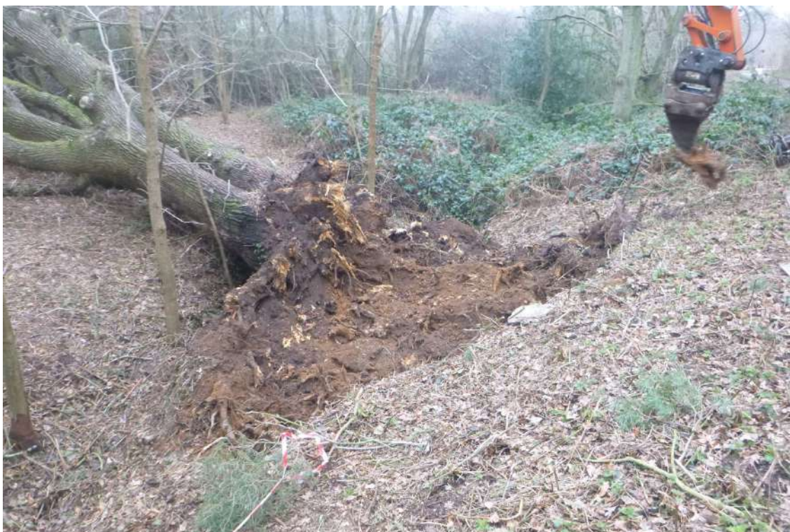
Photograph 3 Breaking up the tree roots, looking south-east
