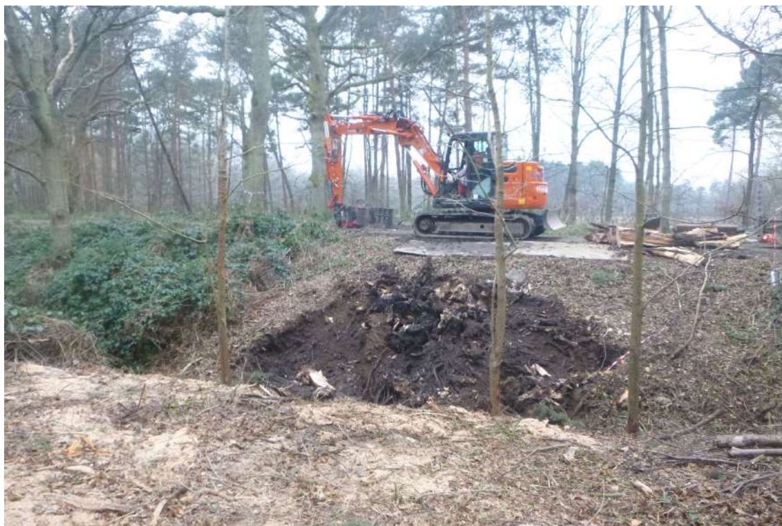
Photograph 6 Tree removed and tree throw backfilled, looking west
