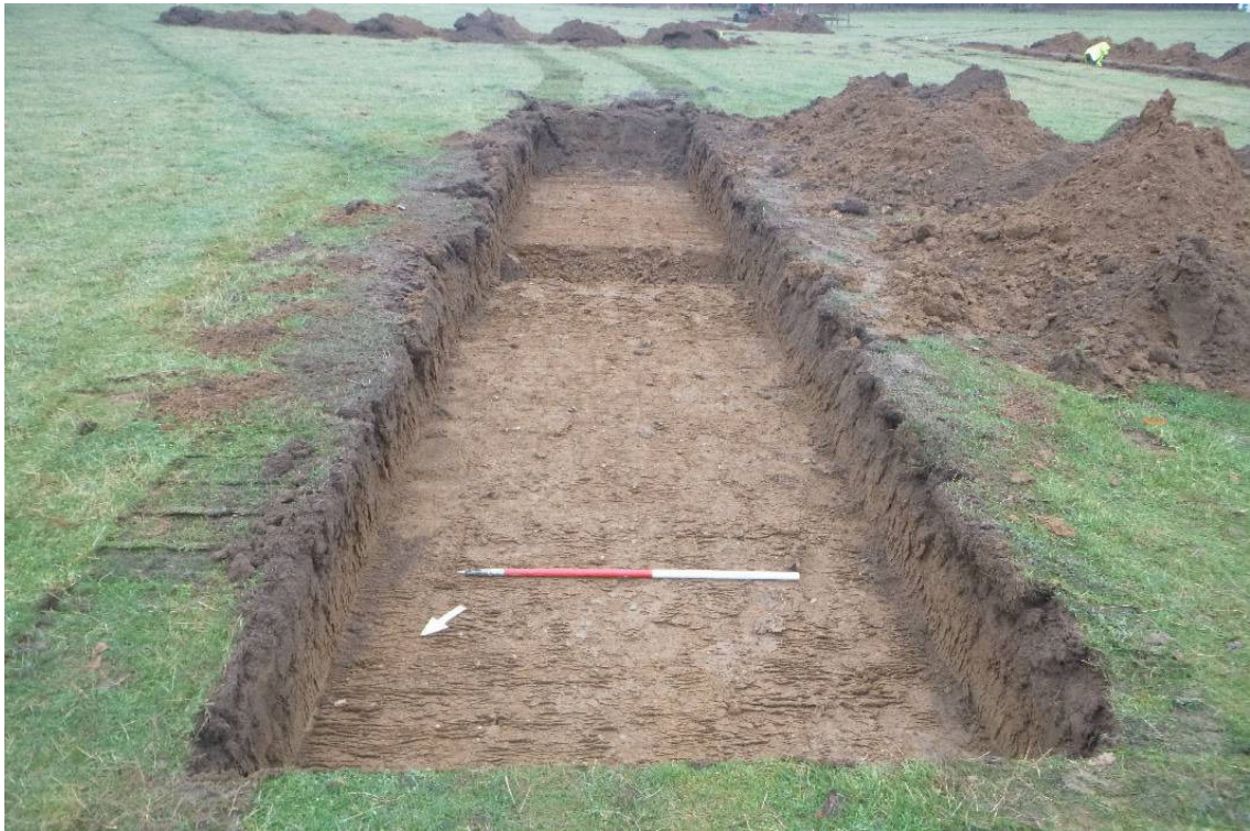
Photograph 3 T2 trench shot, looking southeast.
