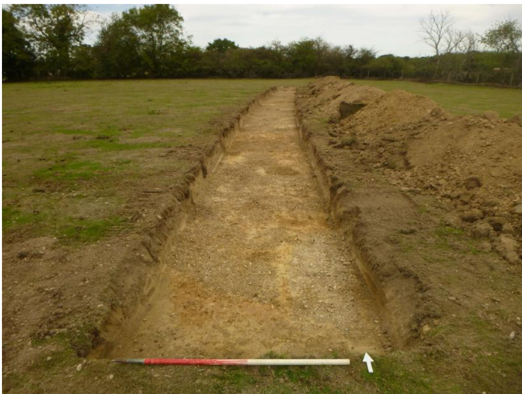
Photograph 5 T54 trench shot, looking north.
