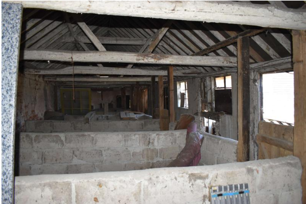
Photograph 20 Interior of store 5. Photograph taken facing north-west.
