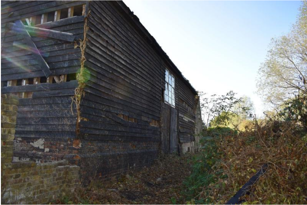
Photograph 4 Western elevation of barn. Photograph taken facing south
