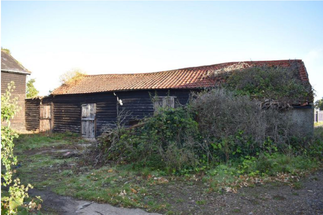
Photograph 6 Southern elevation of interior courtyard. Photograph taken facing north.
