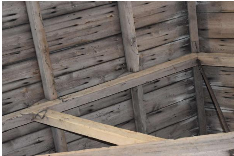
CFTF22_Photograph_119Detail of lower scarf-joint in purlin in western ... CFTF22_Photograph_120Detail of barn roof truss. Photograph taken f...
