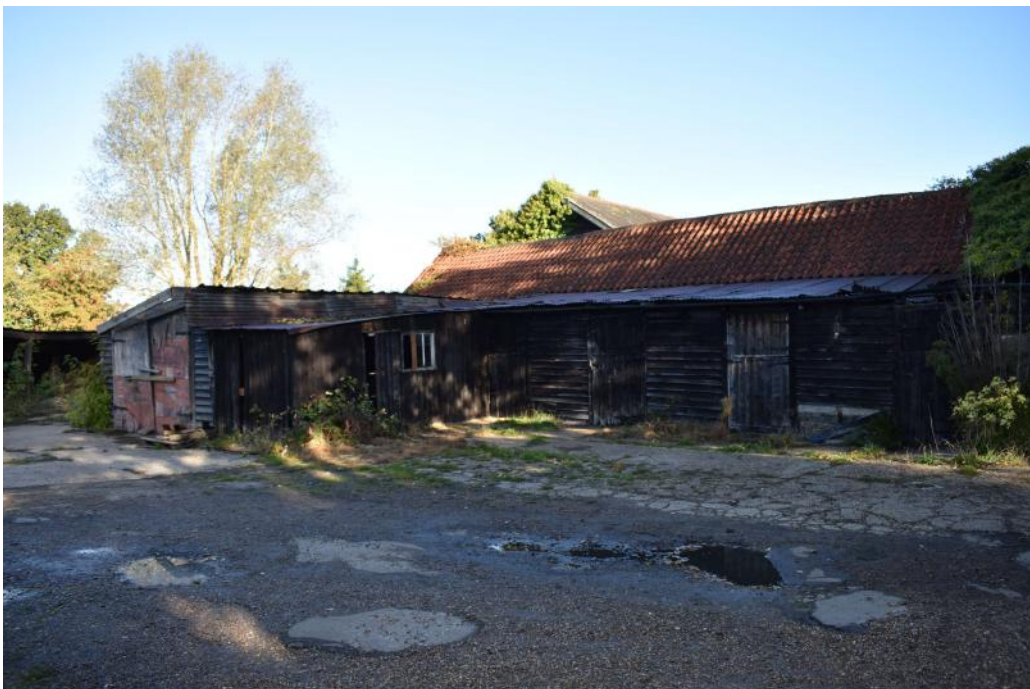
Photograph 5 Eastern and southern elevations of stores 1, 2 and 4. Photograph taken facing north.
