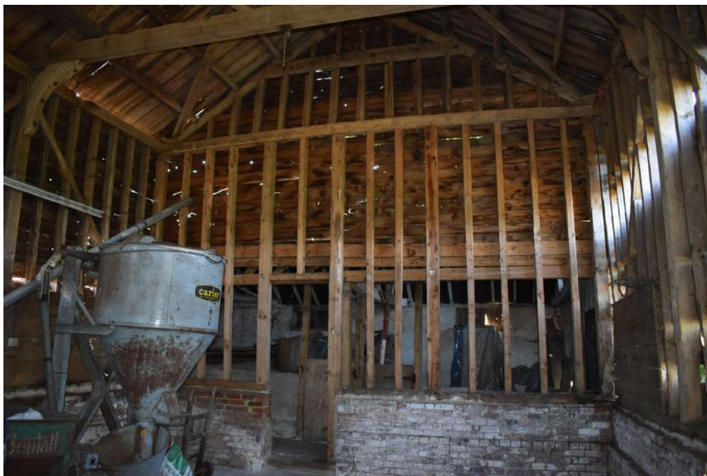
Photograph 12 Southern wall of barn. Photograph taken facing south.
