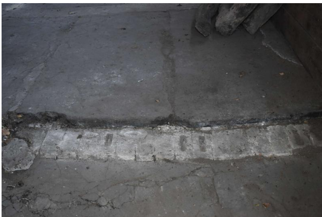
Photograph 11 Detail of shallow-frogged bricks in floor of bay 3 of barn. Photograph taken facing south.
