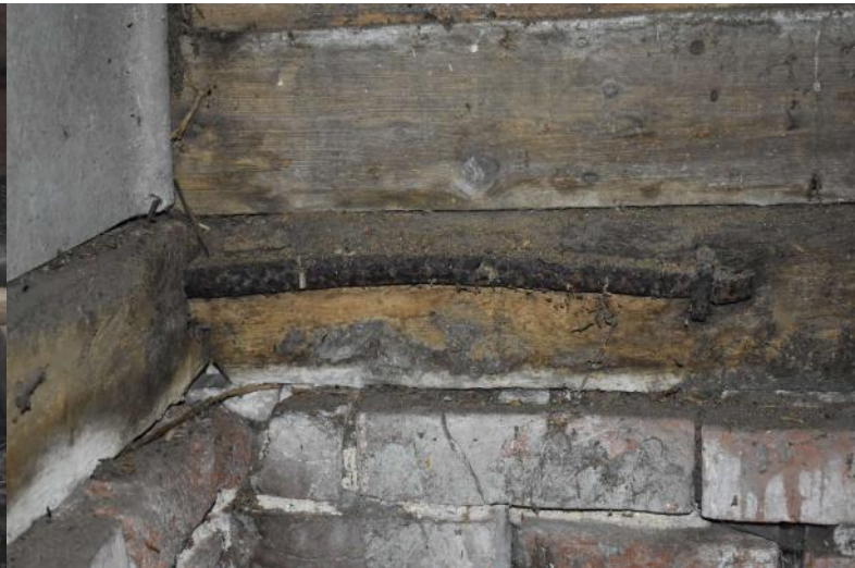
CFTF22_PhotoGraph_125Detail of iron strap on sill-beam of northern ... CFTF22_PhotoGraph_126Detail of scarf joint on sill-beam in eastern w...
