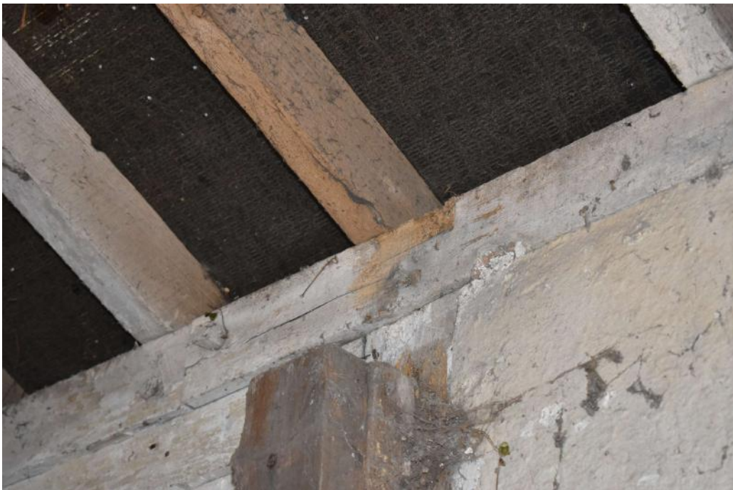
Photograph 24 Detail of removed tie-beam in store 9. Photograph taken facing north.
