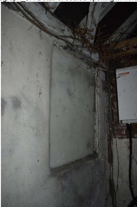
CFTF22_PhotoGraph_077Detail of sealed opening in northern wall of s... CFTF22_PhotoGraph_078Detail of cut bricks in inserted doorway betw...
