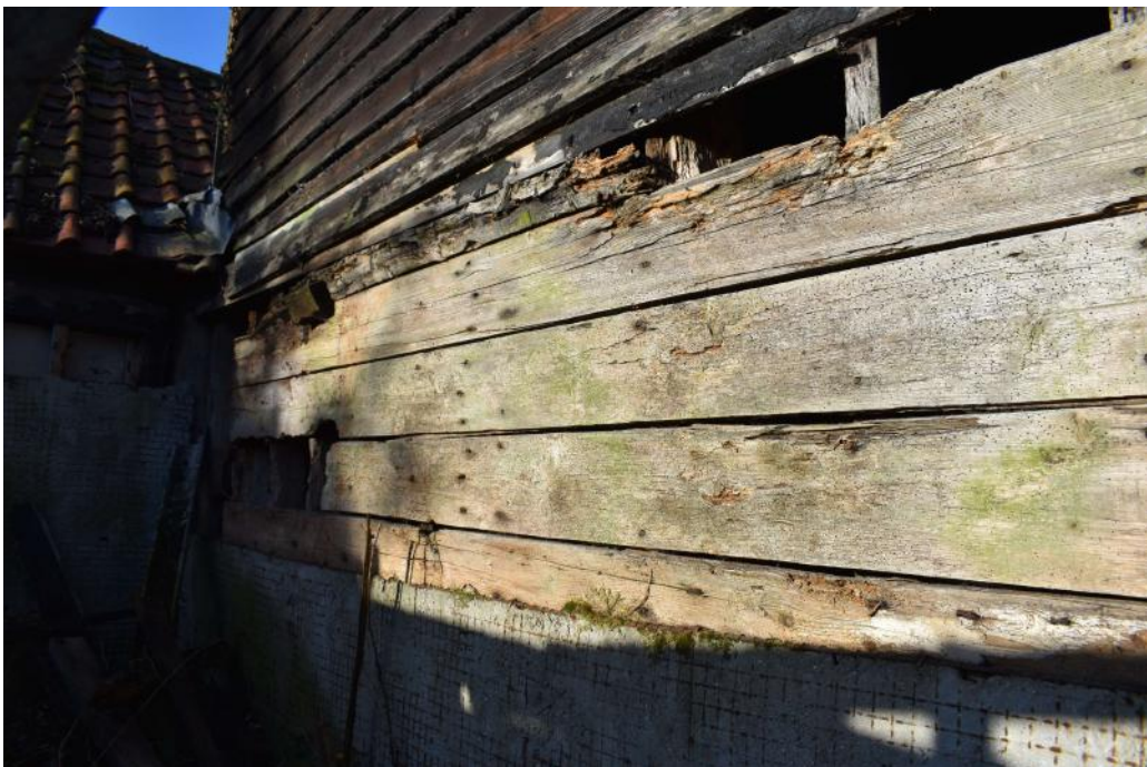
Photograph 2 Possible original weather-boarding on eastern elevation of barn (in store 6). Photograph taken facing south-west.
