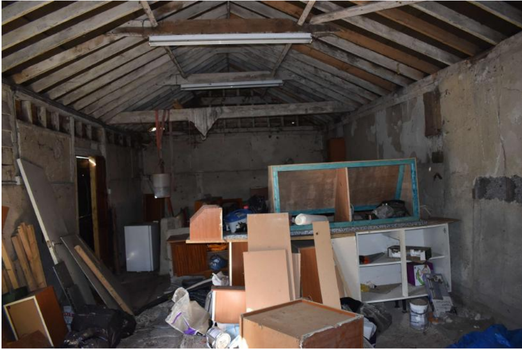
Photograph 23 Interior of store 9. Photograph taken facing north-west.
