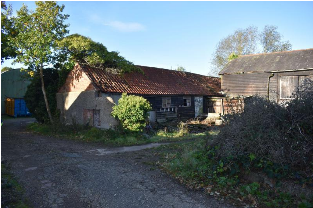
Photograph 7 Northern elevation of the interior courtyard. Photograph taken facing west.
