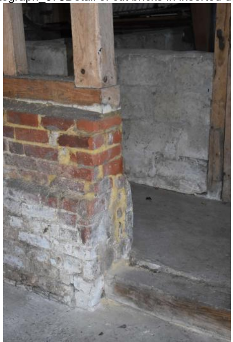
CFTF22_PhotoGraph_077Detail of sealed opening in northern wall of s... CFTF22_PhotoGraph_078Detail of cut bricks in inserted doorway betw...
