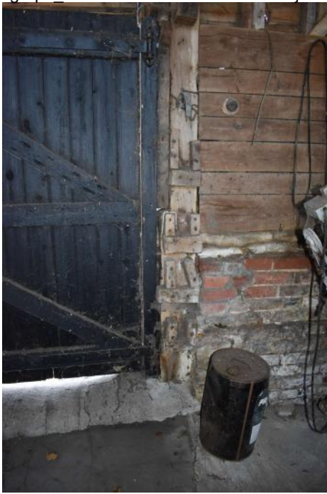
CFTF22_Photograph_117Detail of wooden blocks adjacent to barn do... CFTF22_Photograph_118Detail of upper scarf-joint in purlin in western...
