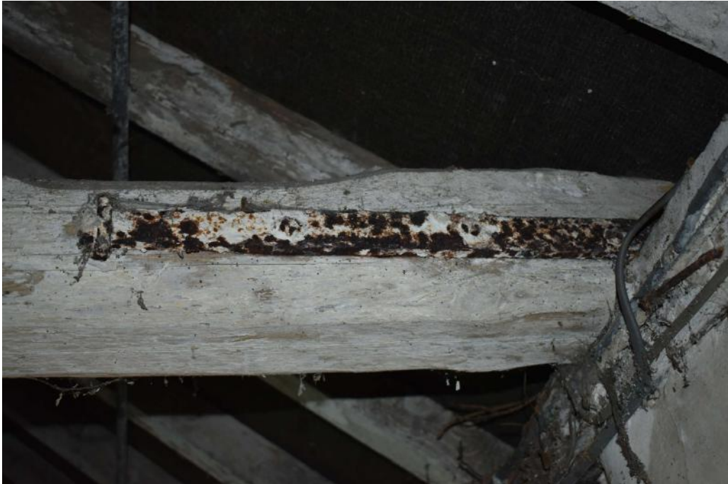
Photograph 22 Detail of iron-strap on tie-beam of store 5. Photograph taken facing north-west.
