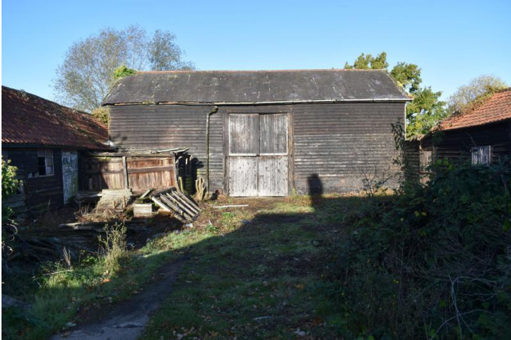
Photograph 1 Eastern elevation of barn. Photograph taken facing west north-west.
