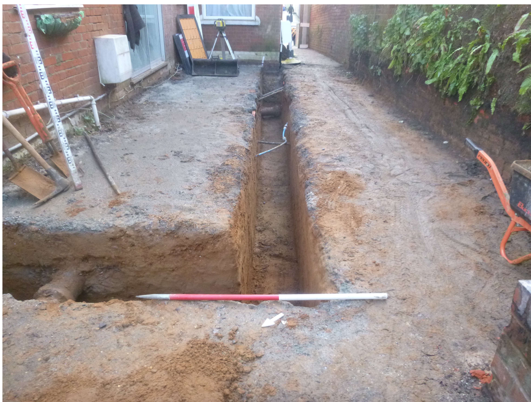
Photograph 3 Foundation trench, view south-east.
