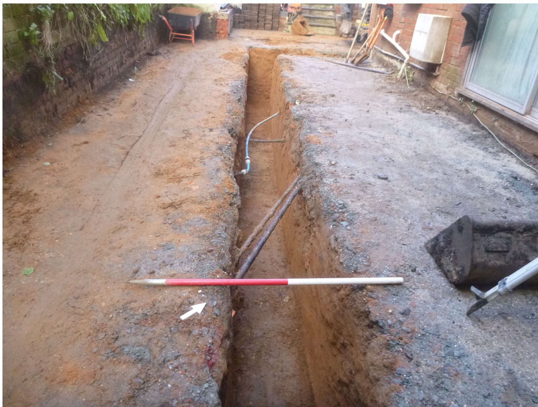
Photograph 4 Foundation trench, view north-west.
