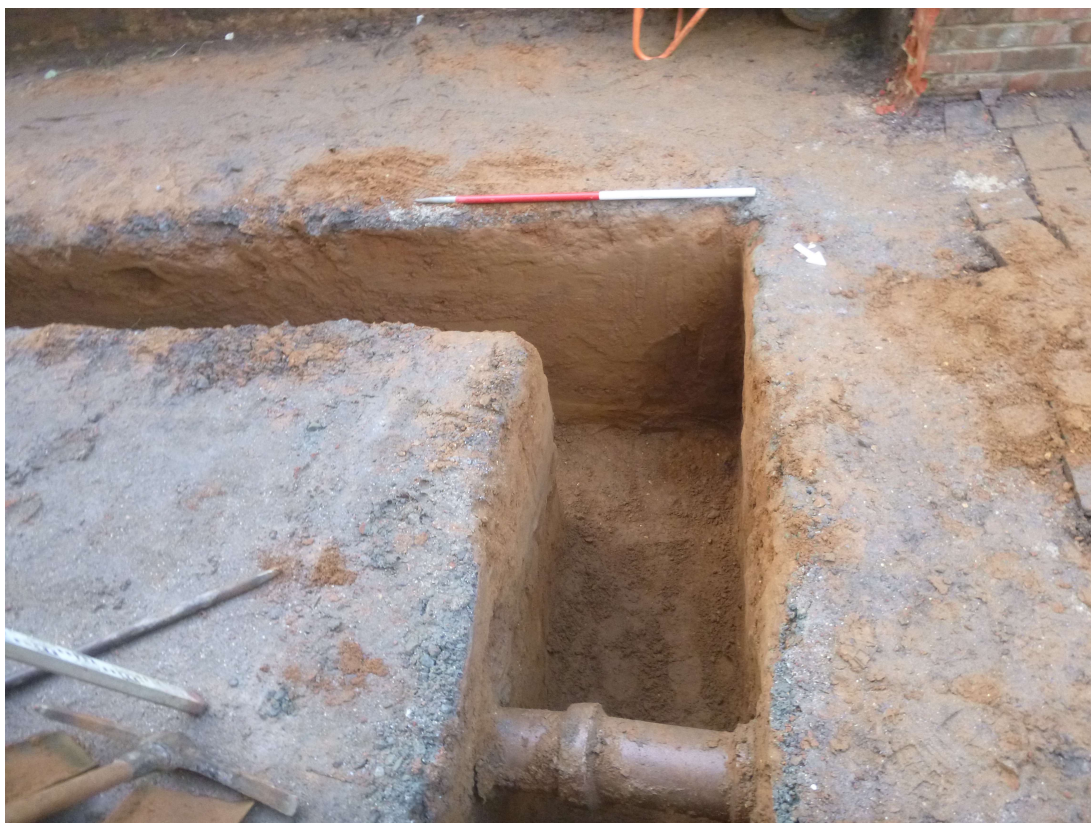
Photograph 2 Foundation trench, view south-west.
