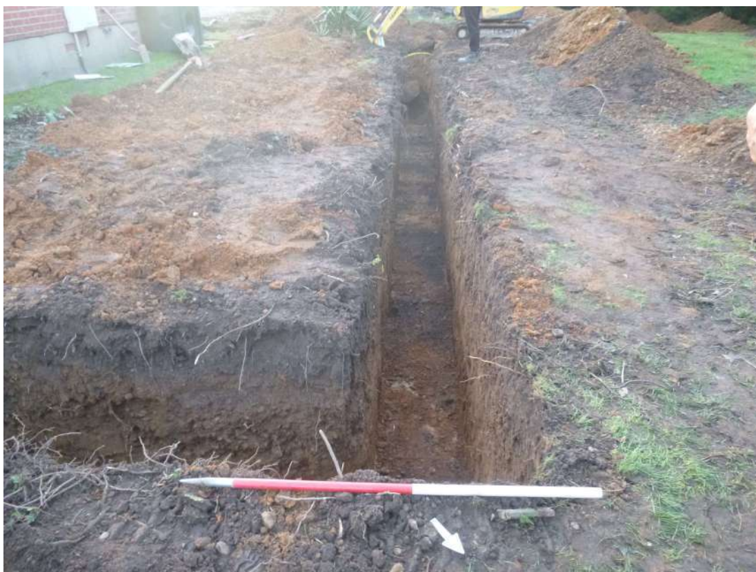
Photograph 3 Foundation trench for the northern extension, view south-west.
