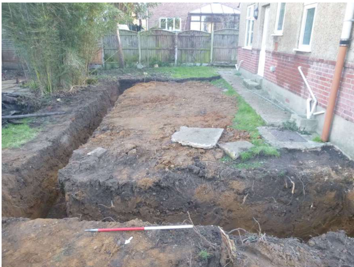
Photograph 2 Foundation trench for the eastern extension, view south-east.
