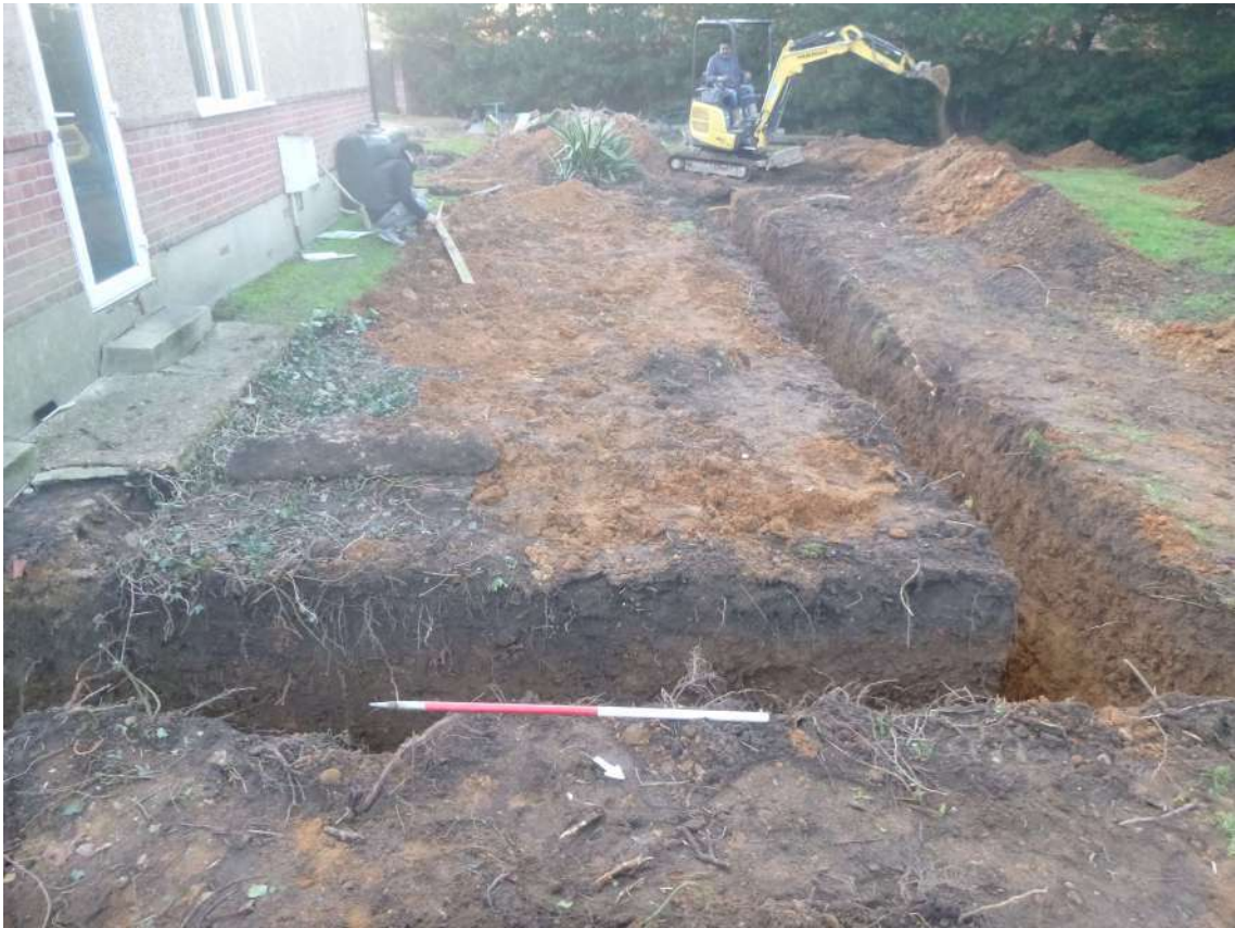
Photograph 4 Foundation trench for the northern extension, view south-west.
