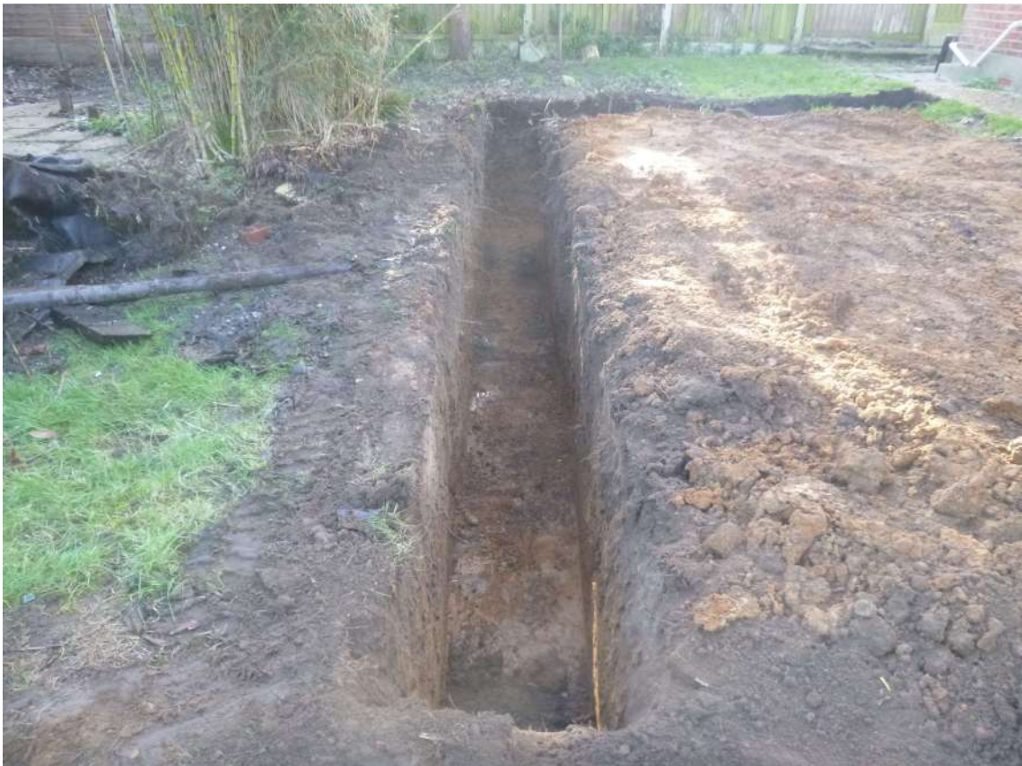
Photograph 1 Foundation trench for the eastern extension, view south-east.
