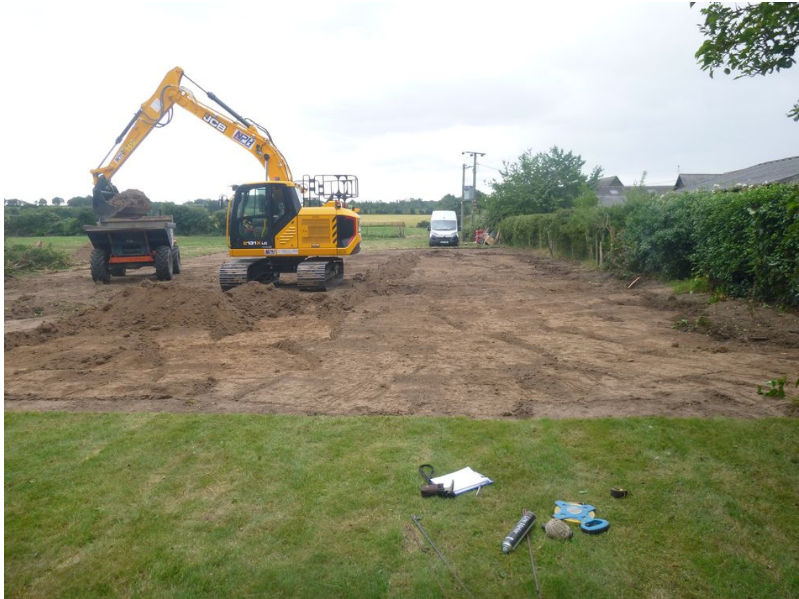
Photograph 1 Area strip/level reduction, view south.
