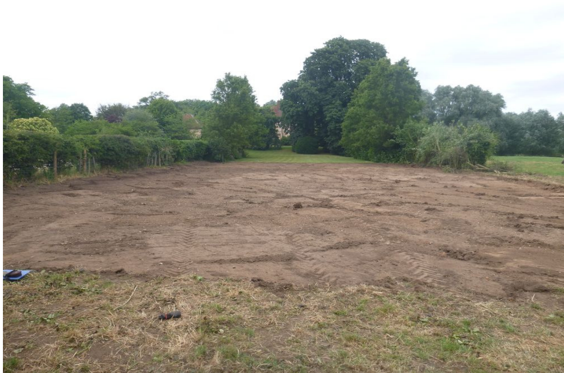
Photograph 2 Completed area strip/reduction, view north.
