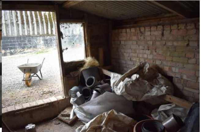
GEAGE23_PhotoGraph_058.JPG Internal view of extension 1. Photograph taken facing north.
