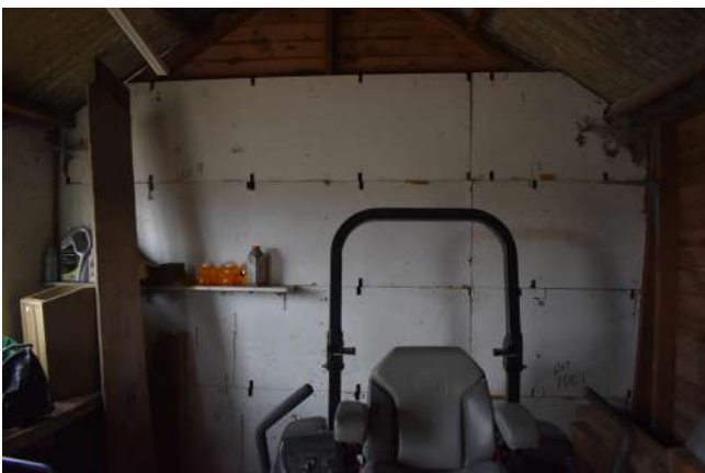
GEAGE23_PhotoGraph_051.JPG Detail of interior wall cladding in sectional timber hut. Photograph taken facing north-w est.
