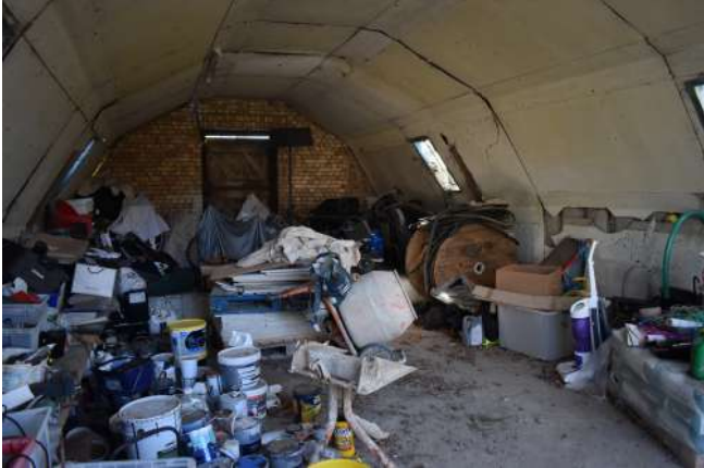
GEAGE23_PhotoGraph_017.JPG Internal view of the handcraft hut. Photograph taken facing north-east.
