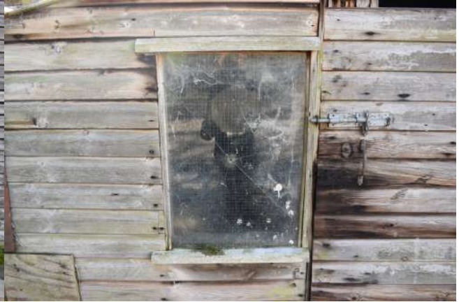
GEAGE23_PhotoGraph_038.JPG Detail of window on northern elevation of modern extension of sectional timber hut. Photograph taken facing south-east.
