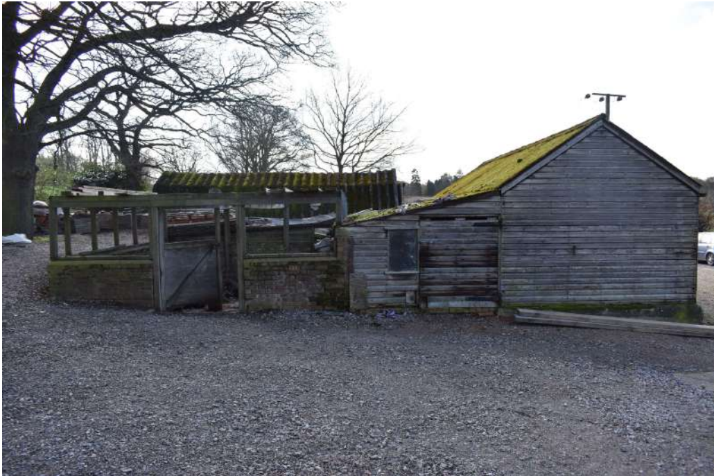
Photograph 11 Northern elevation of sectional timber hut. Photograph taken facing south-east.
