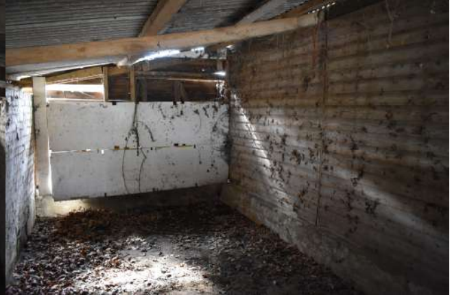
GEAGE23_PhotoGraph_054.JPG Internal view of extension 1. Photograph taken facing south-east.
