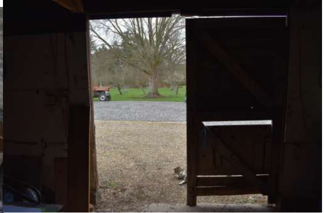
GEAGE23_PhotoGraph_050.JPG Detail of exterior doorway in western wall of sectional timber hut. Photograph taken facing south-w est.
