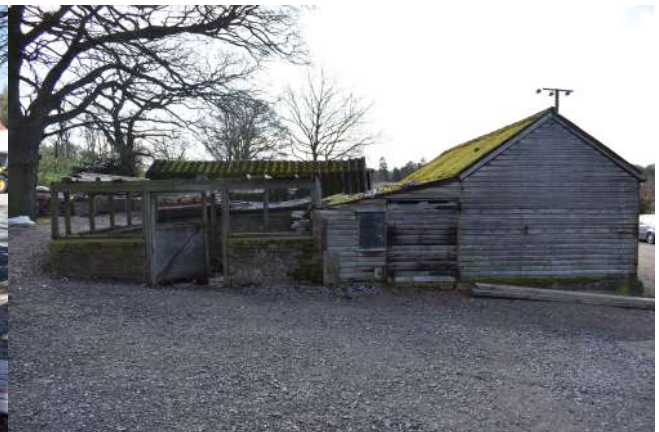
GEAGE23_Phograph_036.JPG Northern elevation of sectional timber hut. Photograph taken facing south-east.
