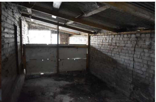
GEAGE23_PhotoGraph_052.JPG Internal view of extension 1. Photograph taken facing north.
