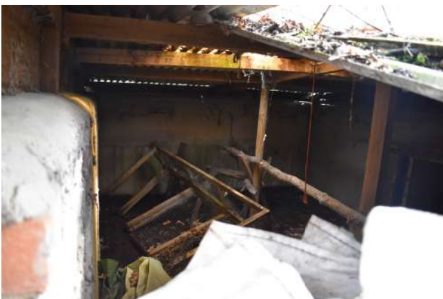
GEAGE23_PhotoGraph_067.JPG Internal view of extension 2. Photograph taken facing east.
