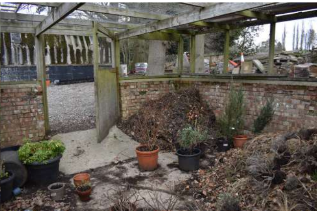
GEAGE23_PhotoGraph_064.JPG Internal view of extension 3. Photograph taken facing north-west.
