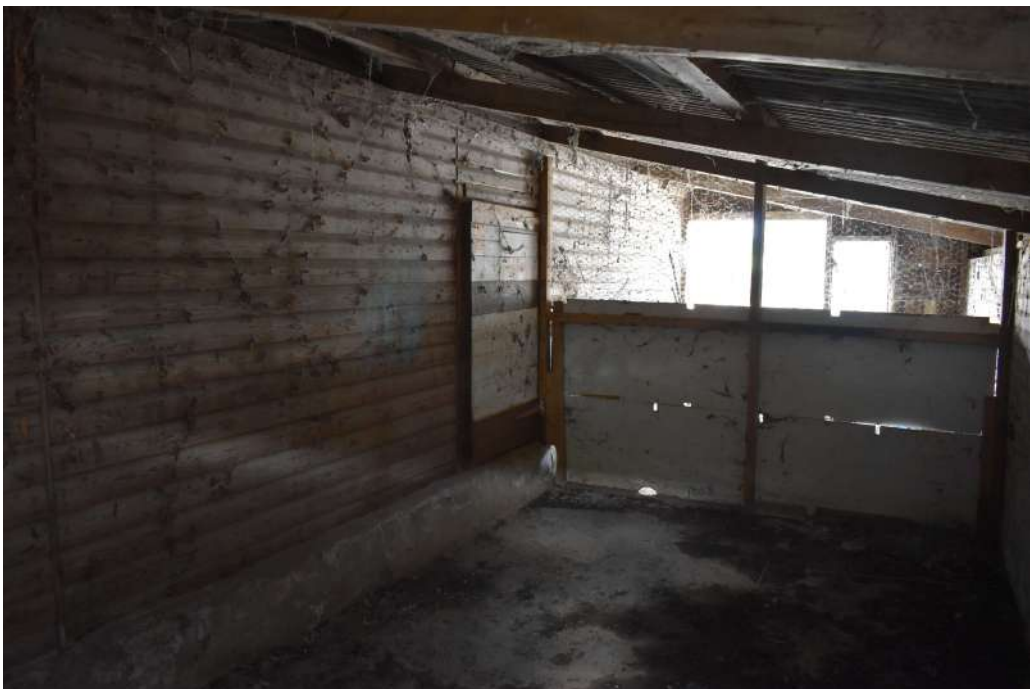
Photograph 15 Internal view of extension 1. Photo taken facing north-west.
