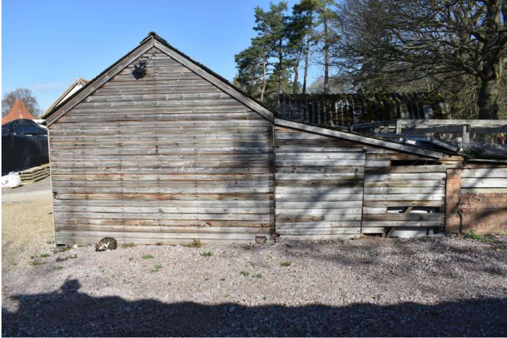
Photograph 12 Southern elevation of the sectional timber hut. Photograph taken facing north-west.
