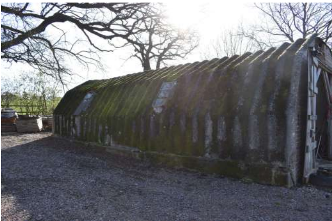
GEAGE23_PhotoGraph_003.JPG Northern elevation of the handcraft hut. Photograph taken facing east.
