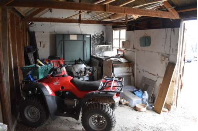
GEAGE23_PhotoGraph_042.JPG Internal view of sectional timber hut. Photograph taken facing south.
