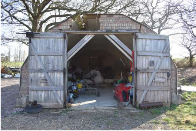
GEAGE23_PhotoGraph_001.JPG Western elevation of the handcraft hut. Photograph taken facing north-east.
