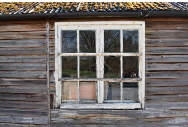
GEAGE23_Photograph_031.JPG Detail of window on western elevation of the sectional timber hut. Photograph taken facing north-east.
