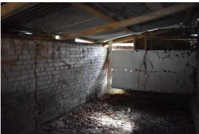
GEAGE23_PhotoGraph_055.JPG Internal view of extension 1. Photograph taken facing south-east.
