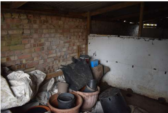
GEAGE23_PhotoGraph_059.JPG Internal view of extension 1. Photograph taken facing east.
