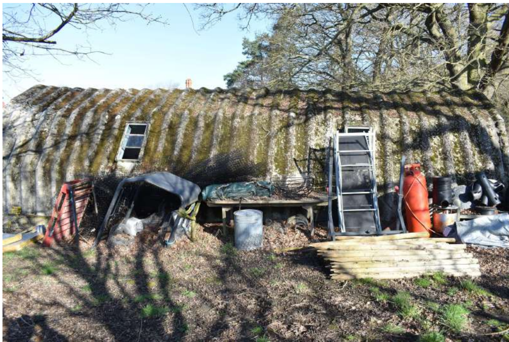
Photograph 5 Southern elevation of the handcraft hut. Photograph taken facing north-west.
