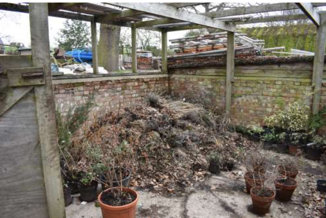
GEAGE23_PhotoGraph_063.JPG Internal view of extension 3. Photograph taken facing south.
