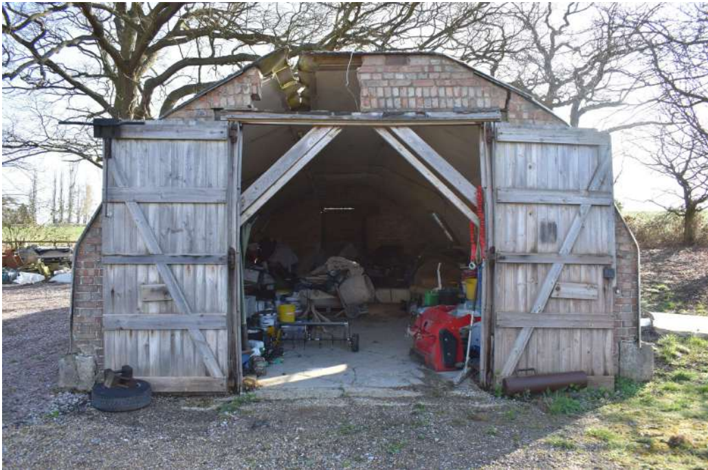
Photograph 4 Western elevation of the handcraft hut. Photograph taken facing north-east.
