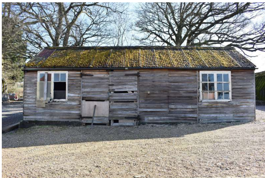
Photograph 10 Western elevation of the sectional timber hut. Photograph taken facing north-east.
