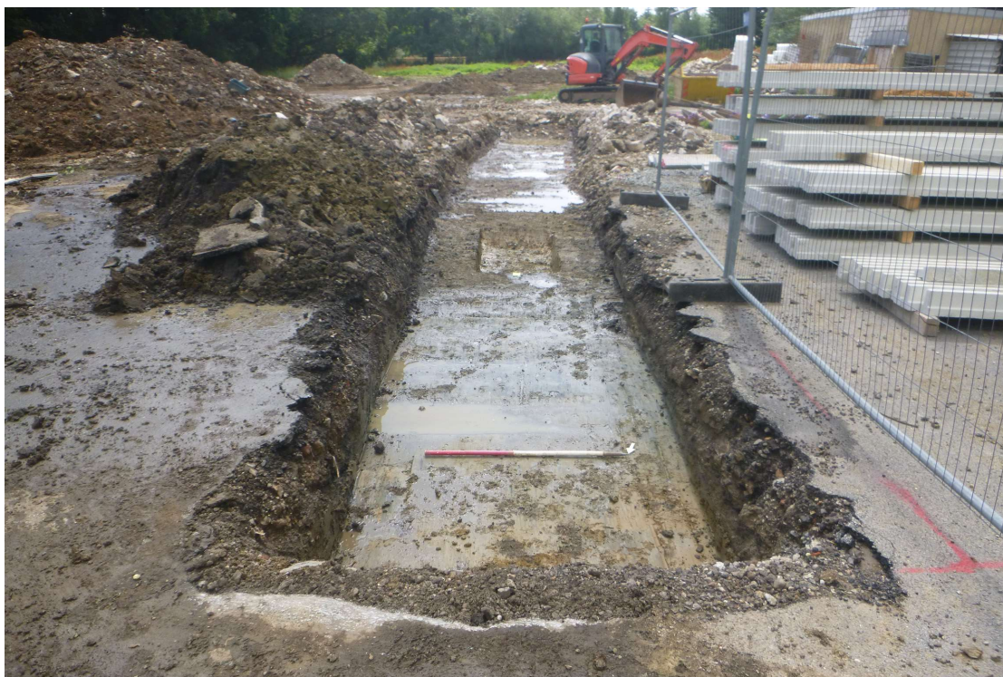
Photograph 2 Trench 2, looking south-south-east.
