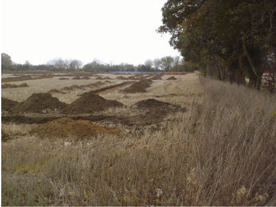
Plate 2: Field A. Trench 1 centre, with Trench 2 behind (view west).
