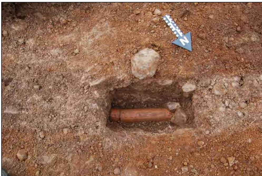
Plate 5: feature 1, showing drainage pipe
