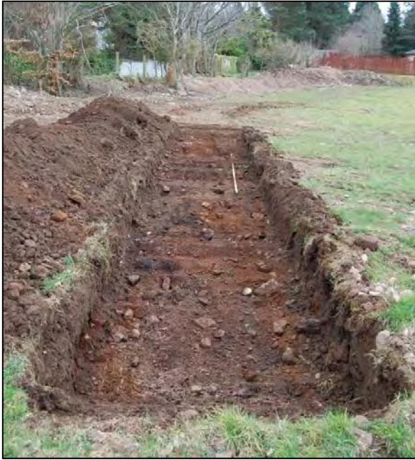
Plate 3 Trench 3 from NW
