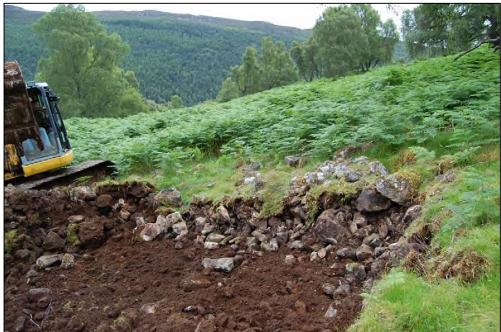
Plate 5 Feature 25 during excavation showing rough NW facing section.
