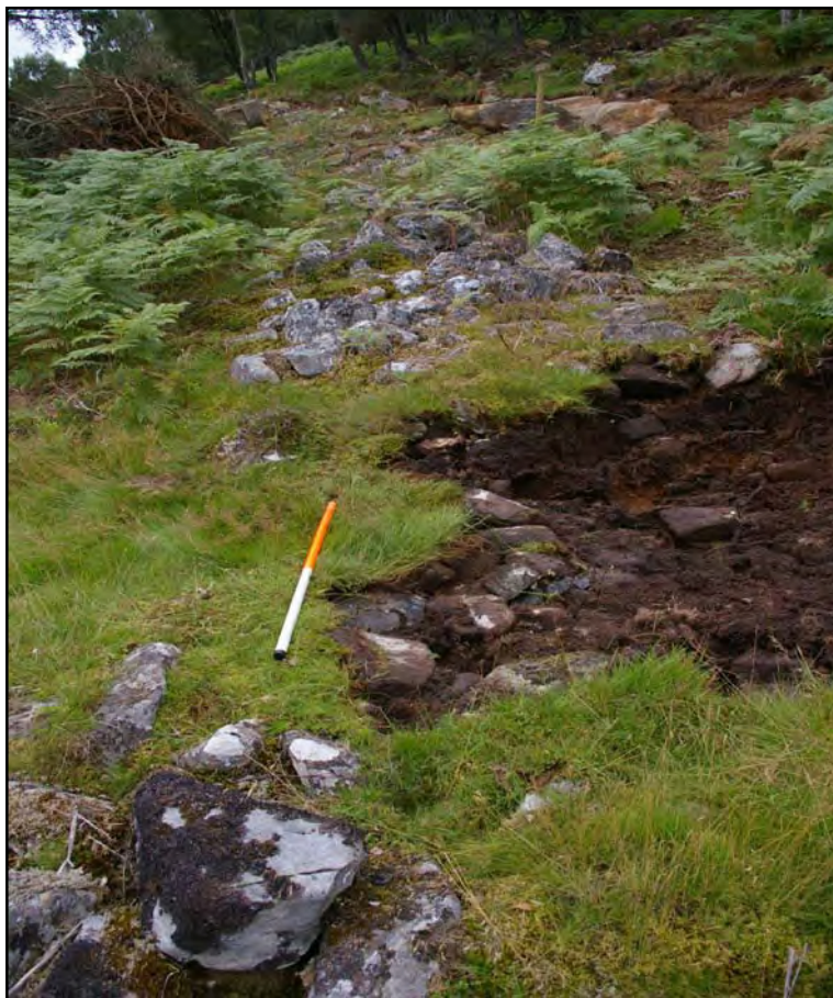
Plate 1 Stripping between F9 and F10 shows the gap to be superficial
