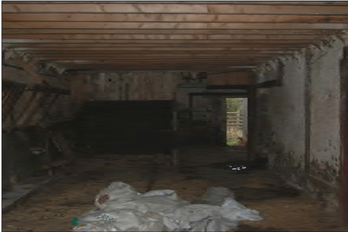
Plate 13 House 6: internal partition
