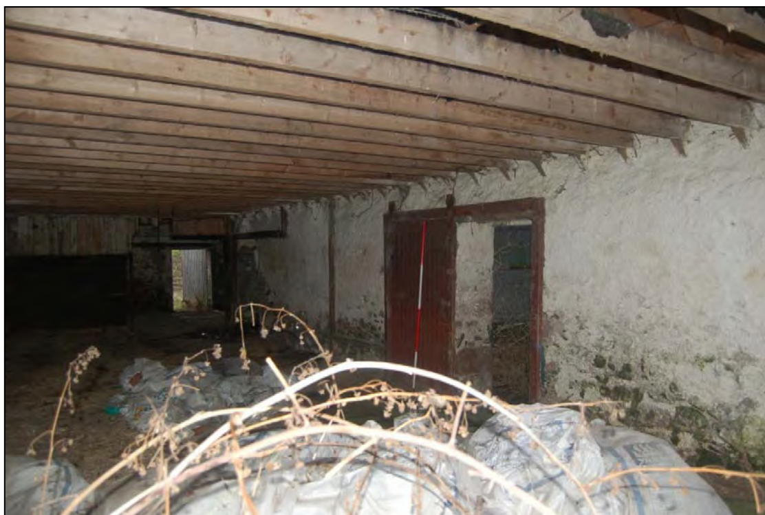
Plate 15 House 6: timber runners on doorway
