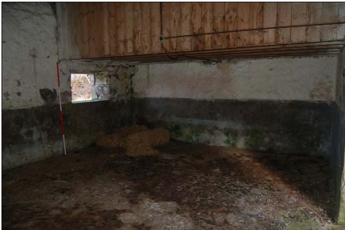
Plate 23 House 9, N room floor joists and upper timber partition forming 1 st floor room
