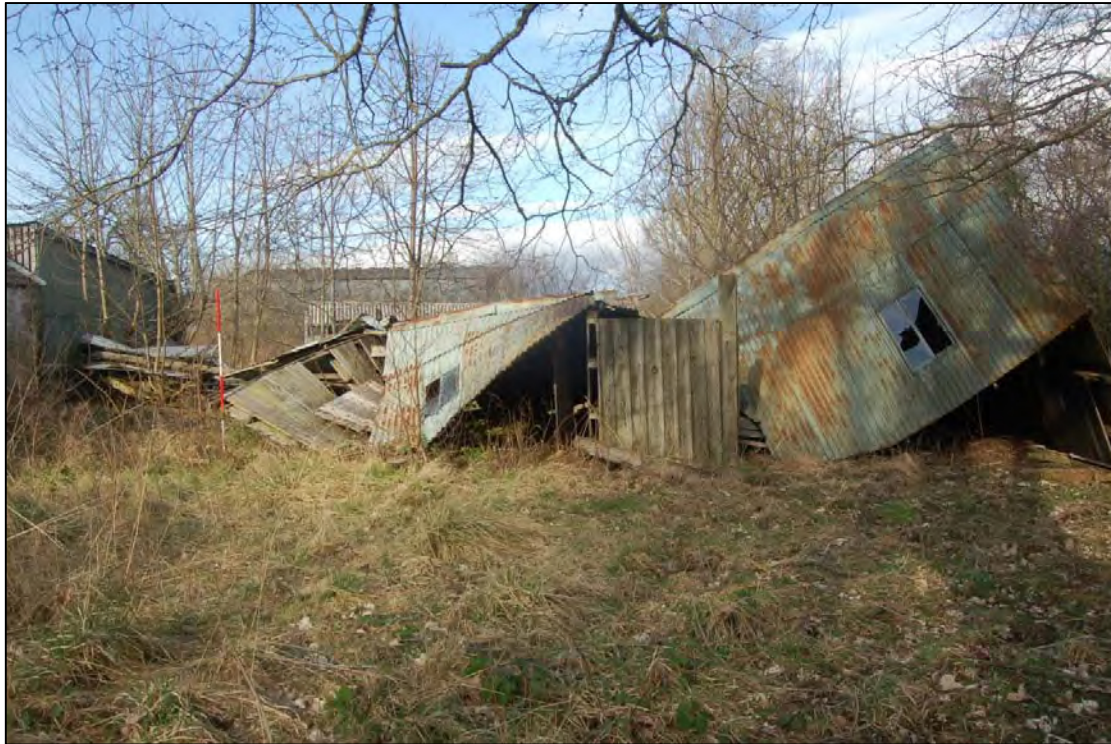
Plate 8 Shed 2 from S
