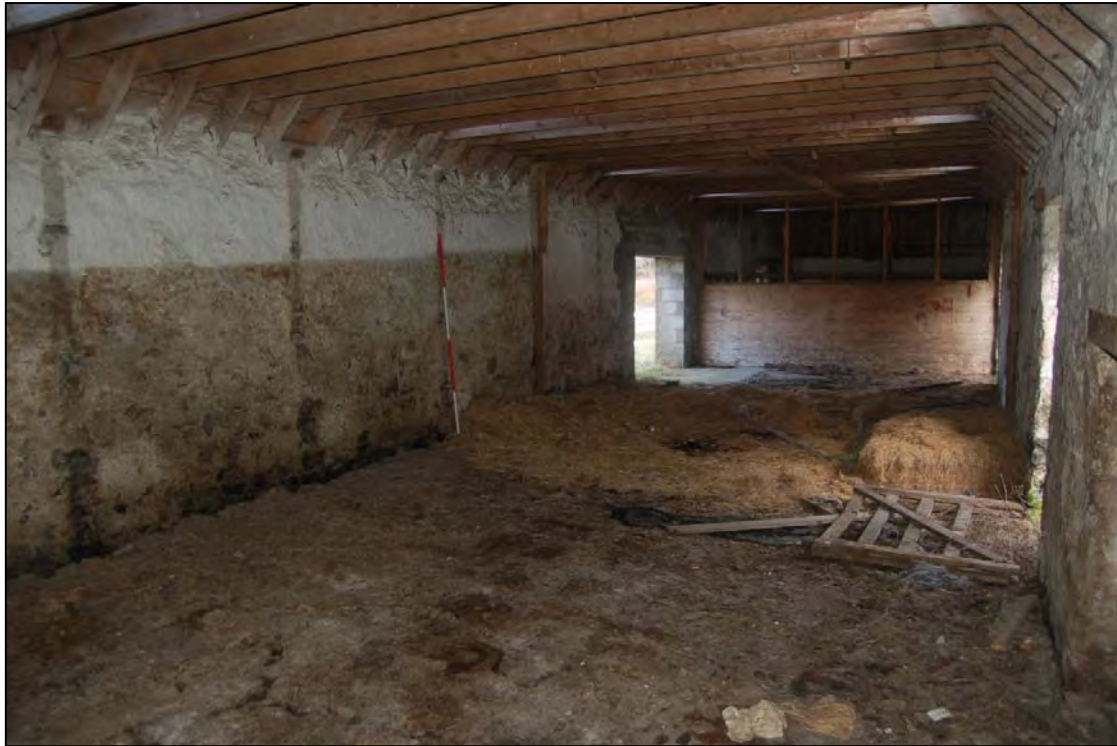
Plate 22 House 9, internal timber partition
