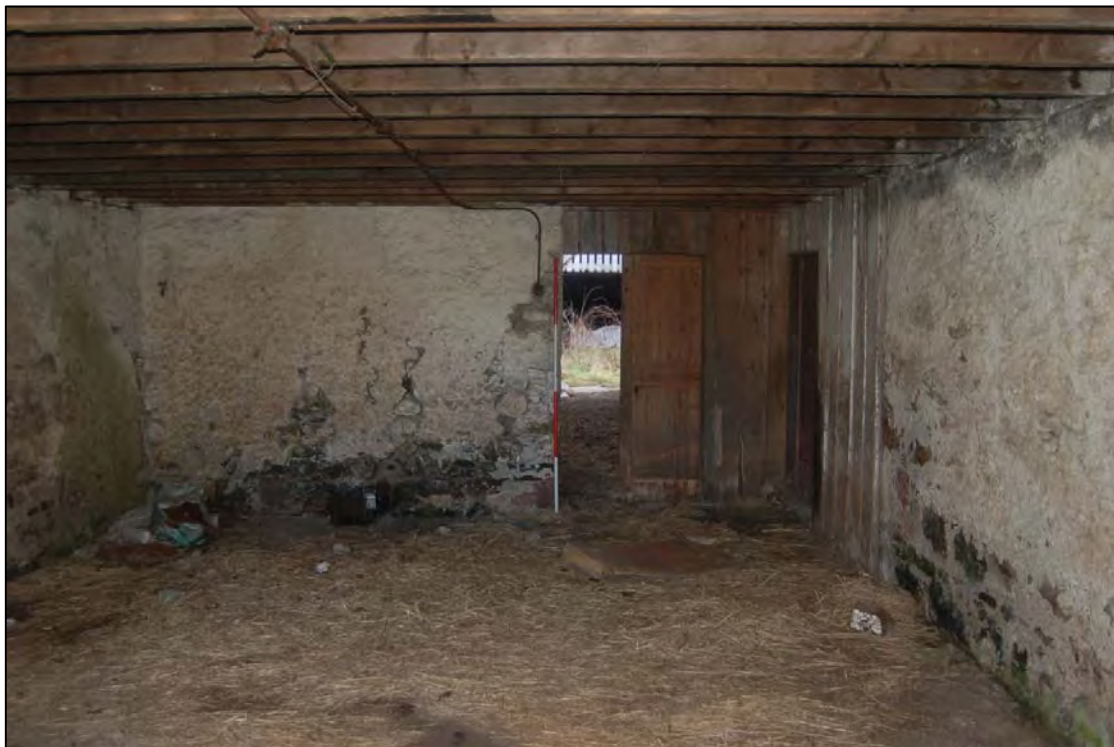
Plate 19 House 8, internal timber partitions and floor joists above
