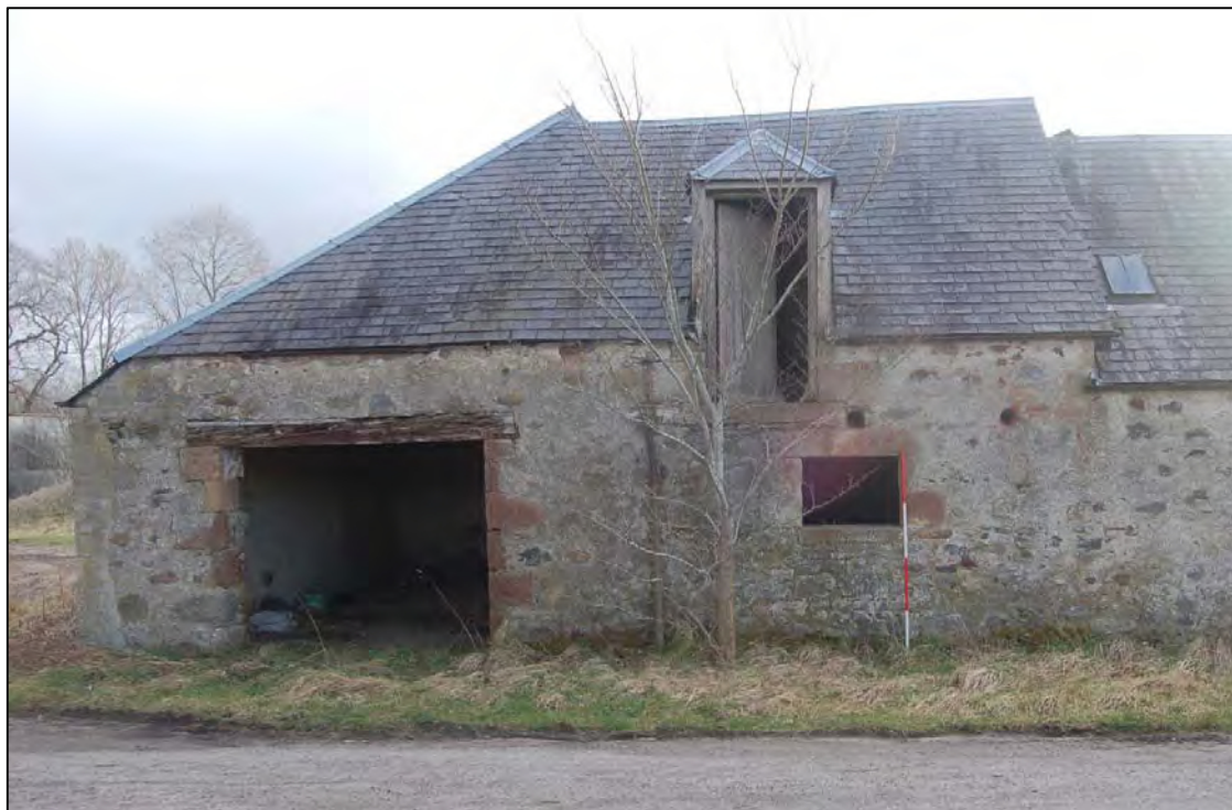
Plate 21 House 9, W elevation showing dormer doorway to upper floor loft
