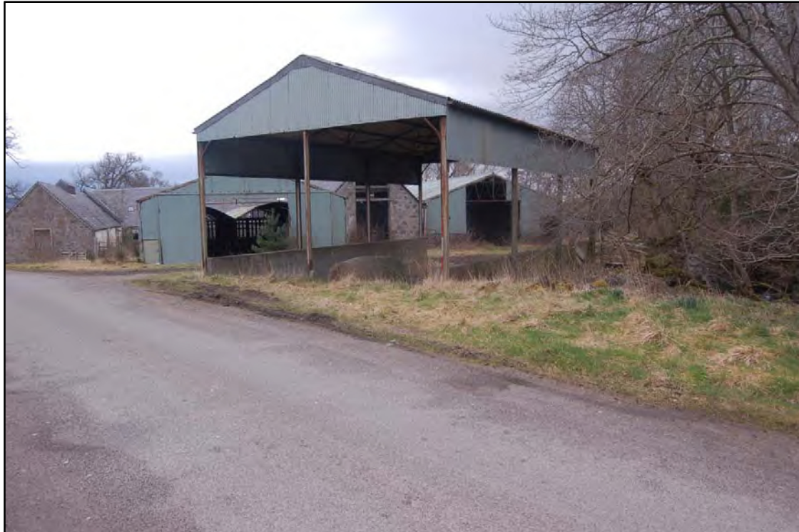
Plate 5 Barn 3 from SSW
