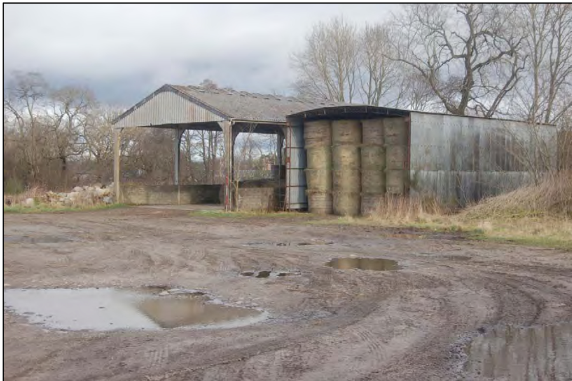
Plate 6 Barn 4 and Shed 4 from SW
