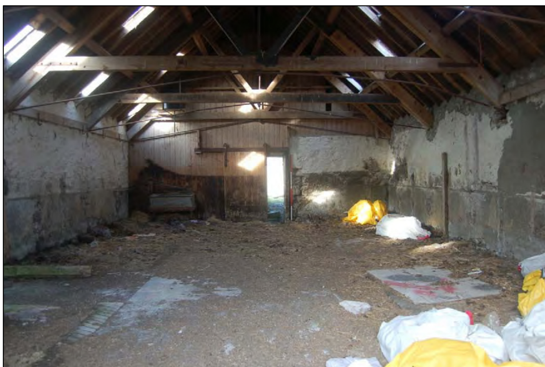
Plate 20 House 8, internal partition extended to roof, forming first floor loft
