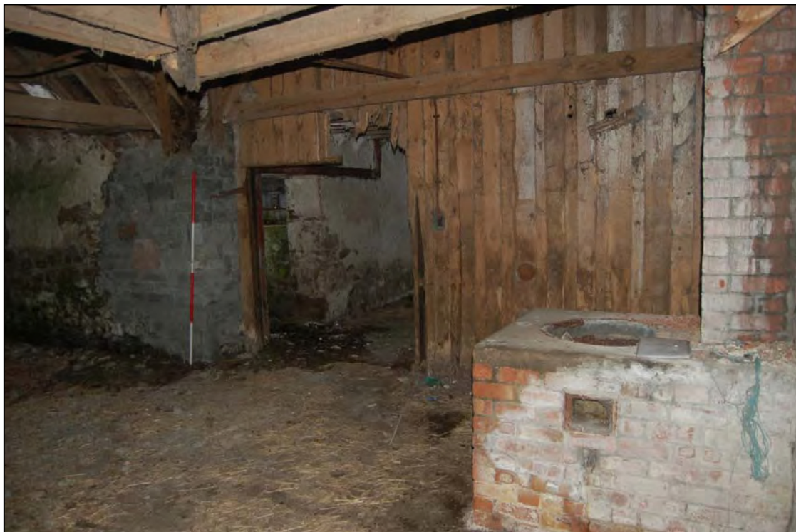
Plate 14 House 6: modern block work repair and wash boiler
