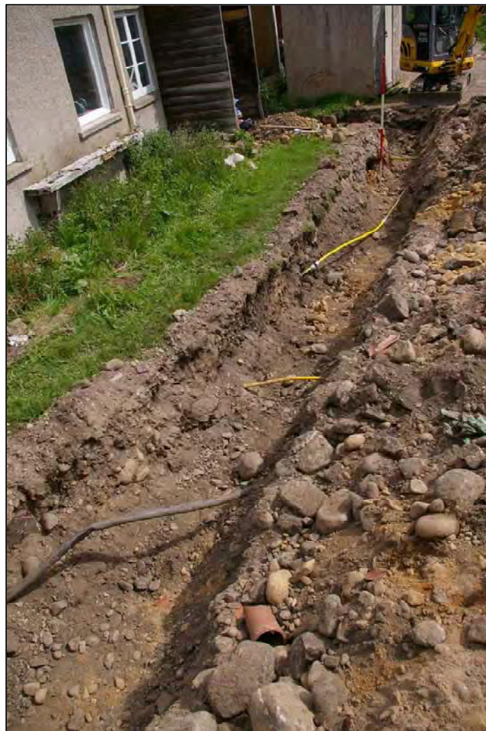
Plate 3 Connection trench, view ENE, showing services and disturbed ground
