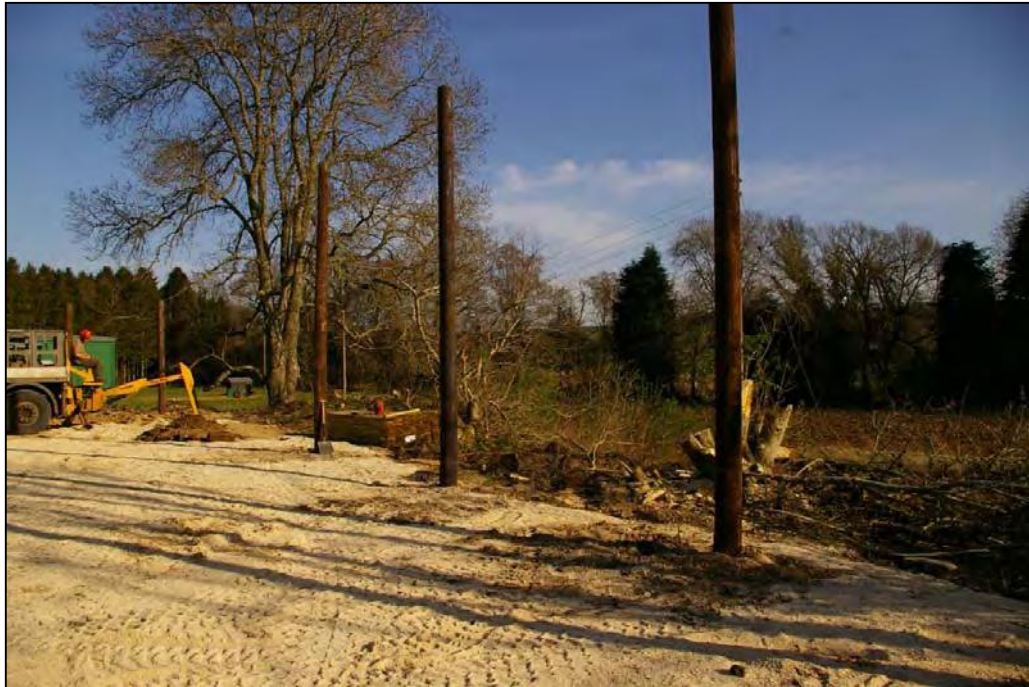
Plate 4 Construction of fuel store
