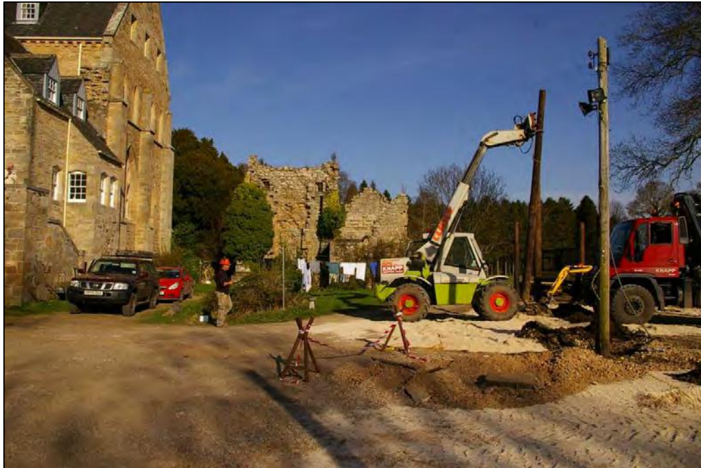
Plate 1 View east, 2012: erection of fuel store poles Compare with Figure 8 above
