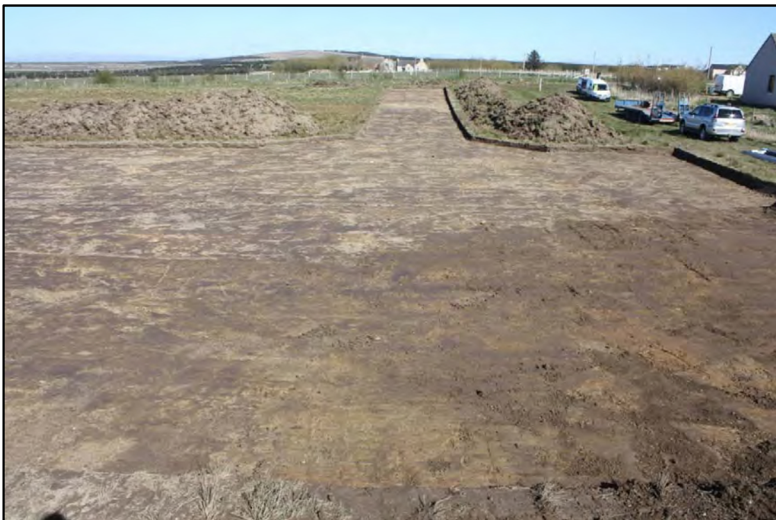
Photo 16 – Stripped area looking E
