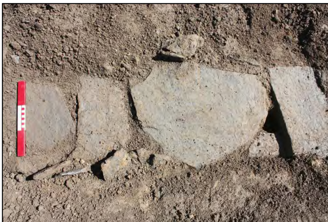
Photo 8 – Phase 1 land drain – detail of capping stones
