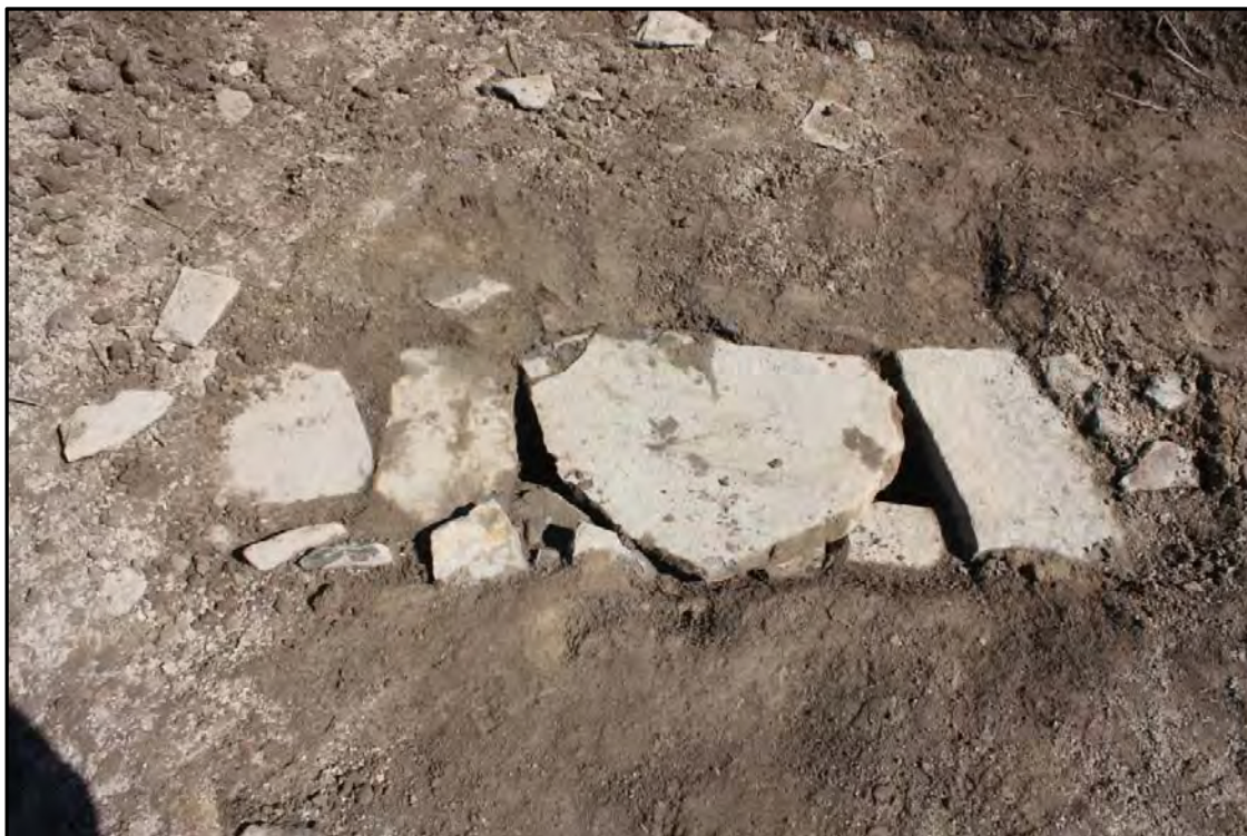
Photo 10 – Phase 1 land drain re-instated
