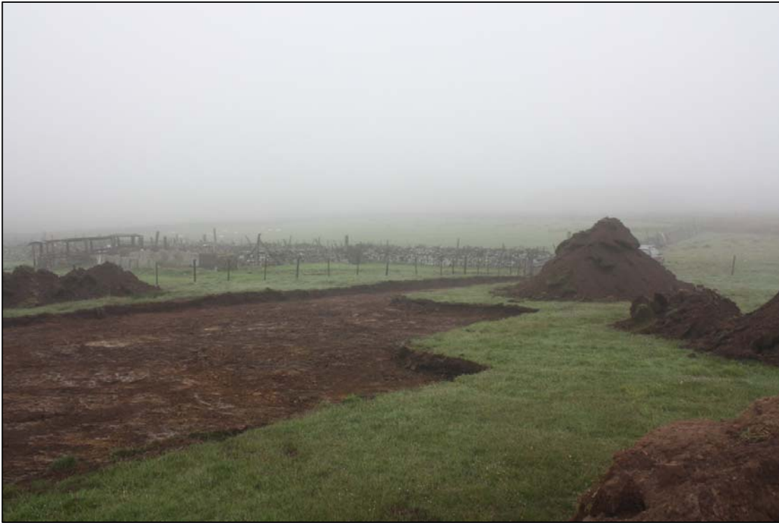
Photo 9 Stripped area looking NW
