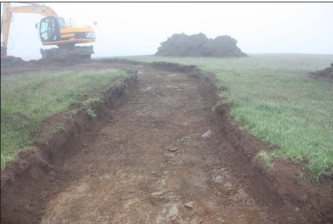
Photo 6 Foul water drain track cleared, looking N
