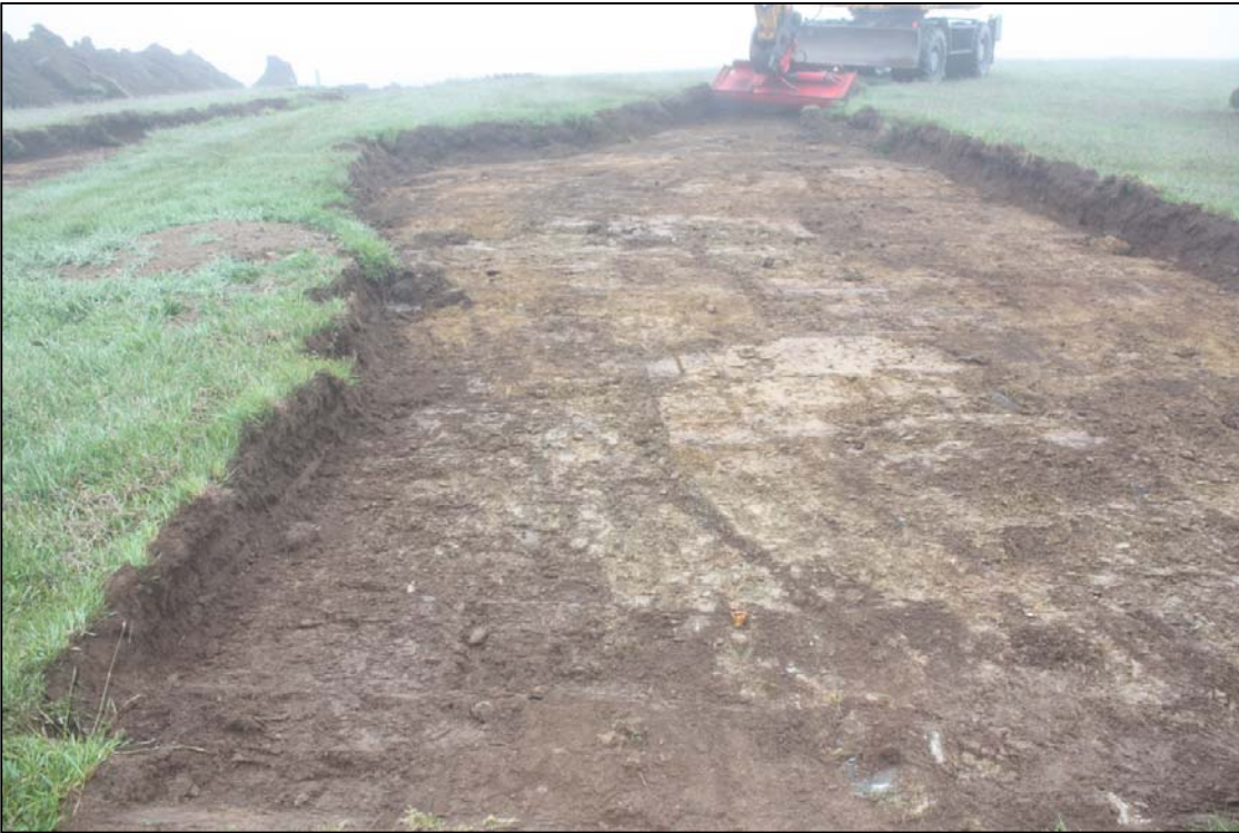
Photo 5 Septic tank and soak-away area cleared looking N
