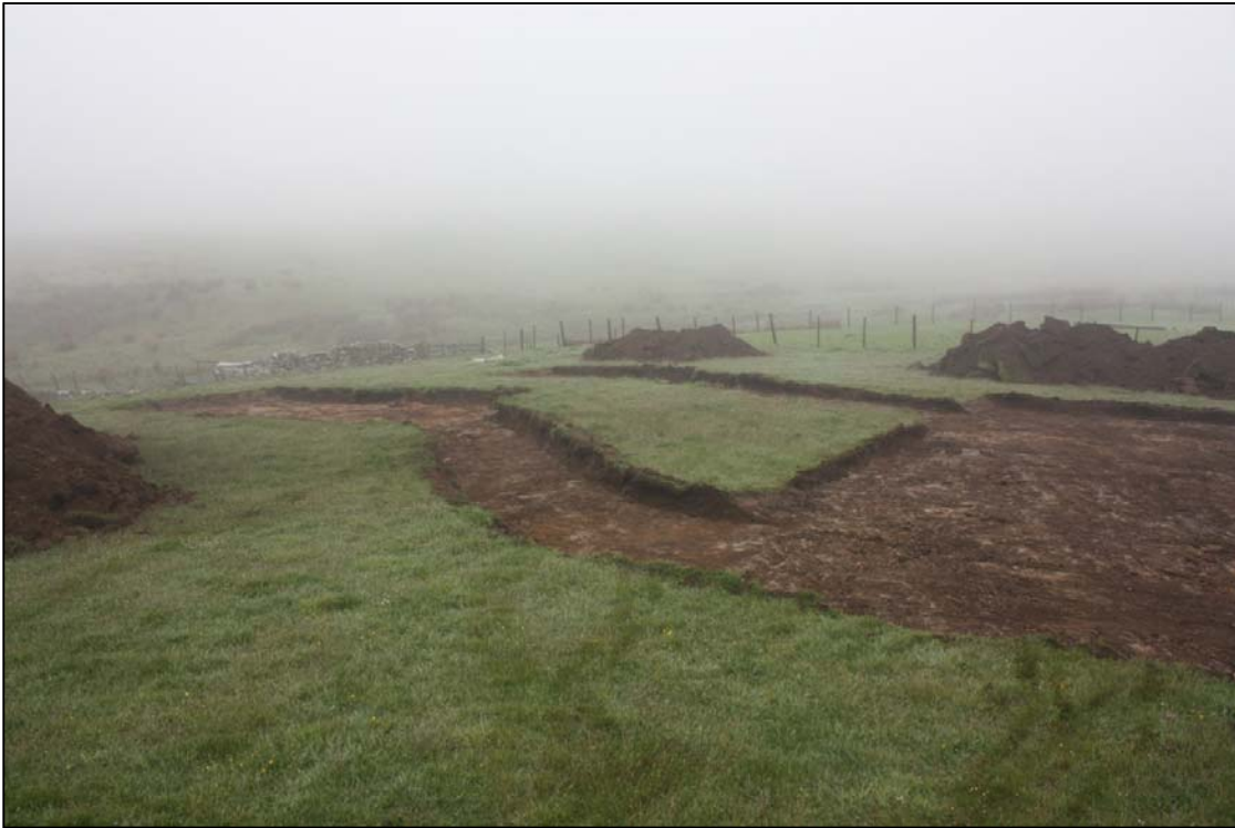
Photo 7 Stripped area looking SW
