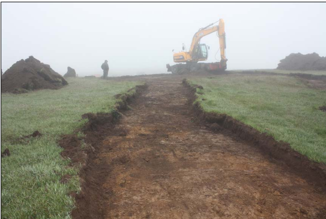
Photo 4 Rain water drain track cleared, looking N
