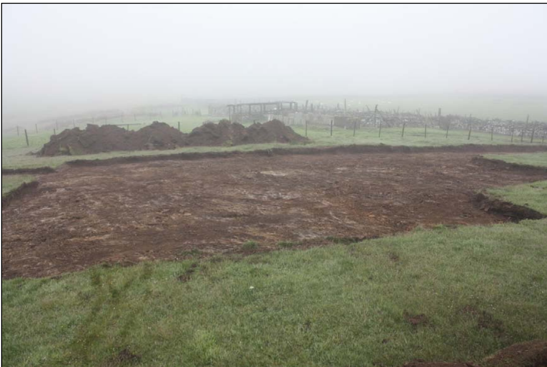
Photo 8 Stripped area looking W
