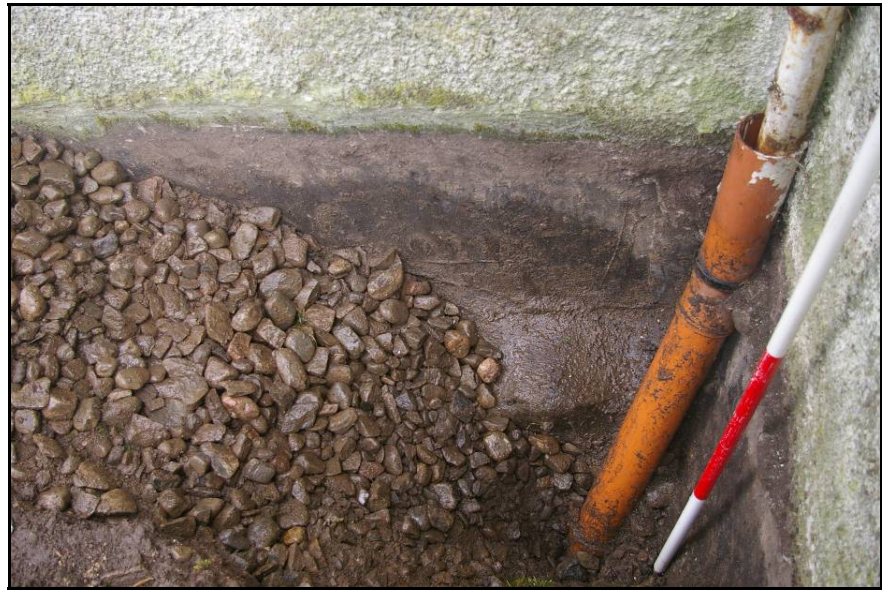
Figure 3 Trench A: excavated to c.1m below present ground level only
