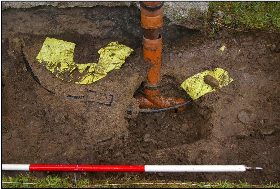
Figure 5 Trench B: downpipe running into perforated pipe and electricity cable
