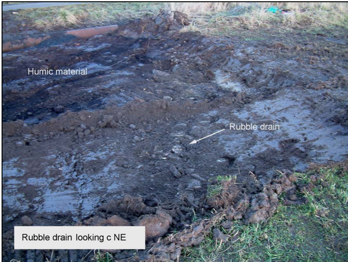
Figure 10 Rubble drain looking NE (Image 7)
