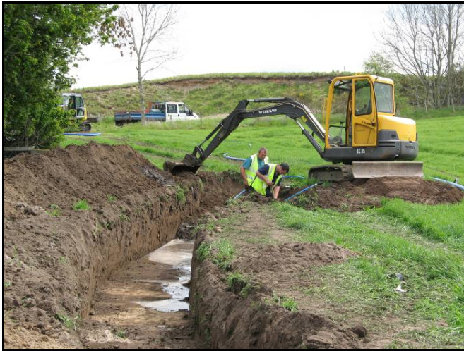
Figure 5 Excavation of watching brief trench - repairing water main
