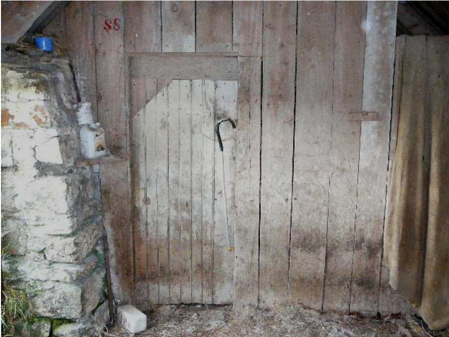
**Figure 18** Interior partition and reused door
