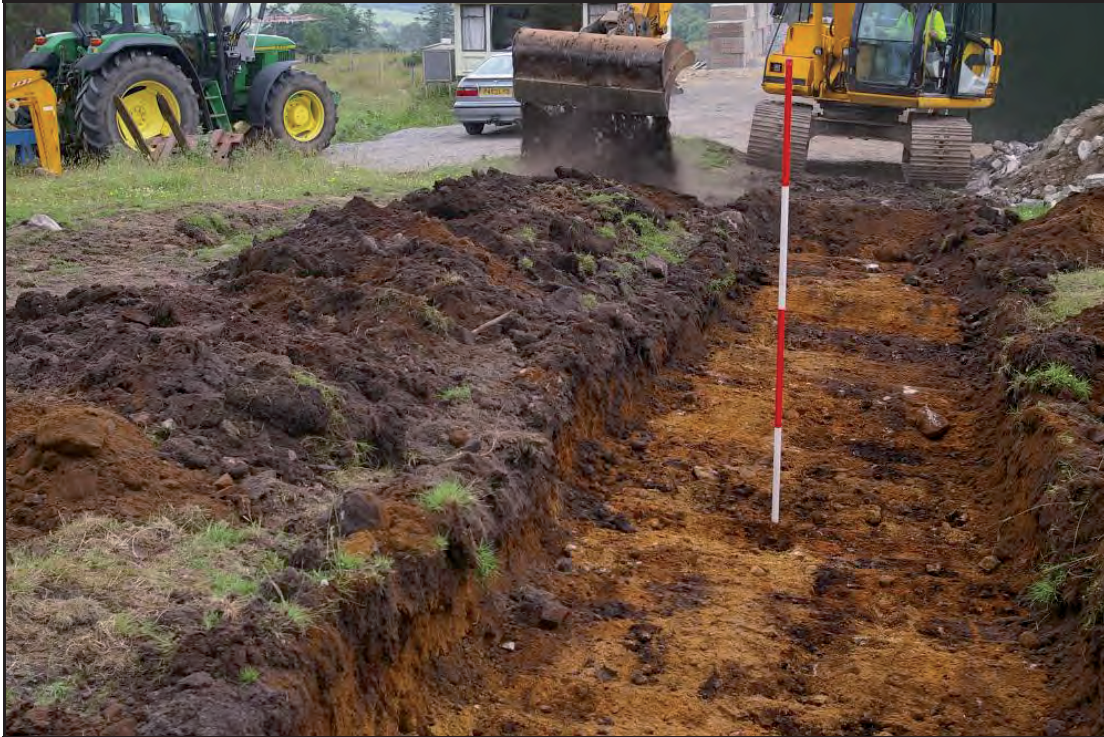
Plate 5 Trench 1 under excavation, July 2008
