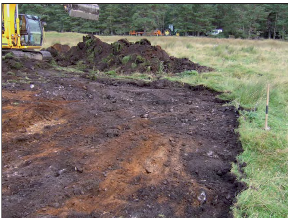
Plate 3 Clearing the house site - showing ground conditions.
