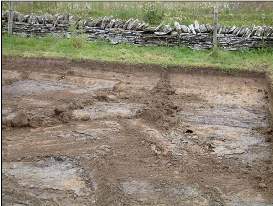
6: Bedrock appearing approx. 40 cm below surface (Photo 2) Location and direction shown as No. 2 on site plan above
