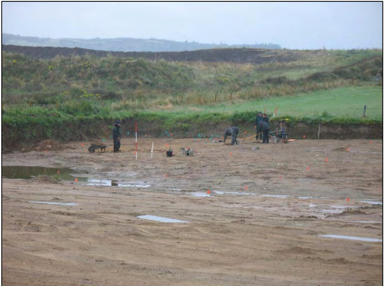
Plate 1 Wet weather made conditions difficult and large areas of the site flooded.
