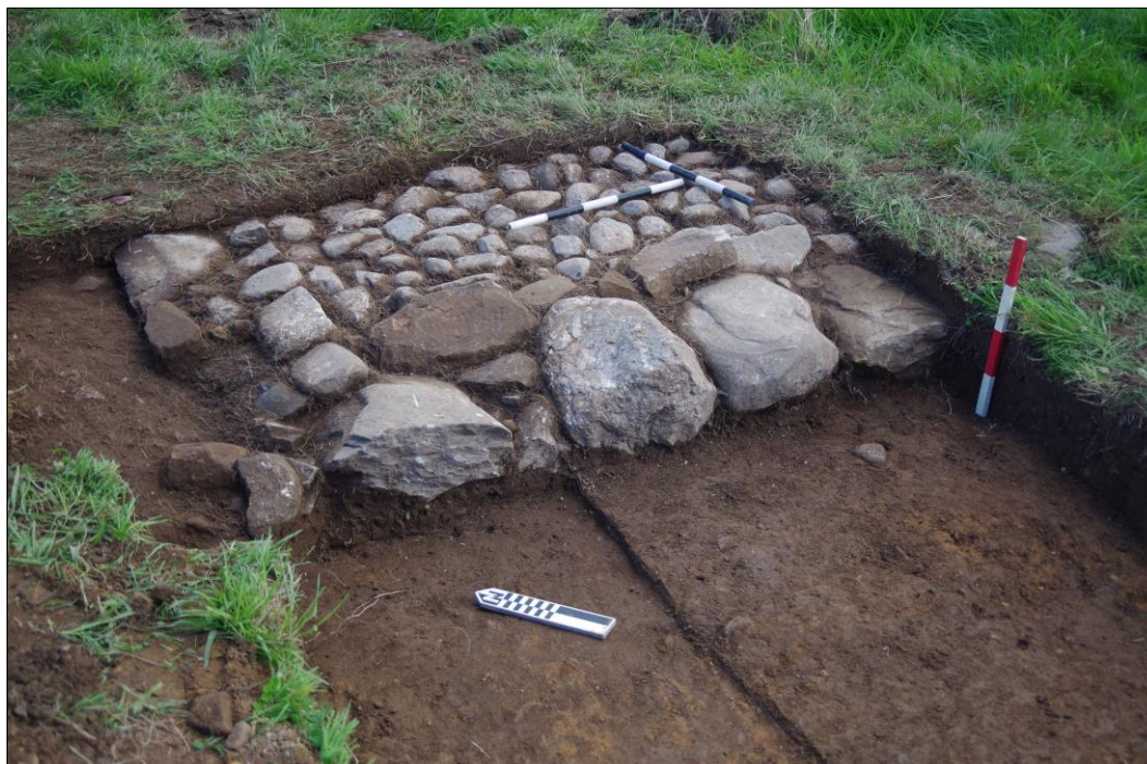
Figure 23 - Wall foundations 1308 and 1309 and cobbled floor 1310, after cleaning. Facing NE. Scales 500mm and 400mm.
