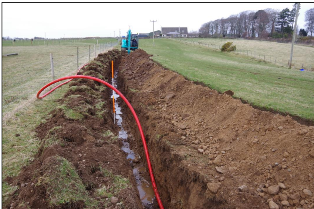
Figure 14: The cable trench as excavated. Facing NW. Scale 2m
