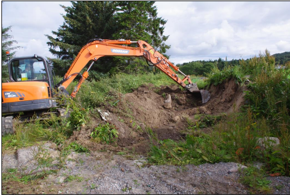
Figure 8 – Removal of modern spoil heaps in progress. Facing N
