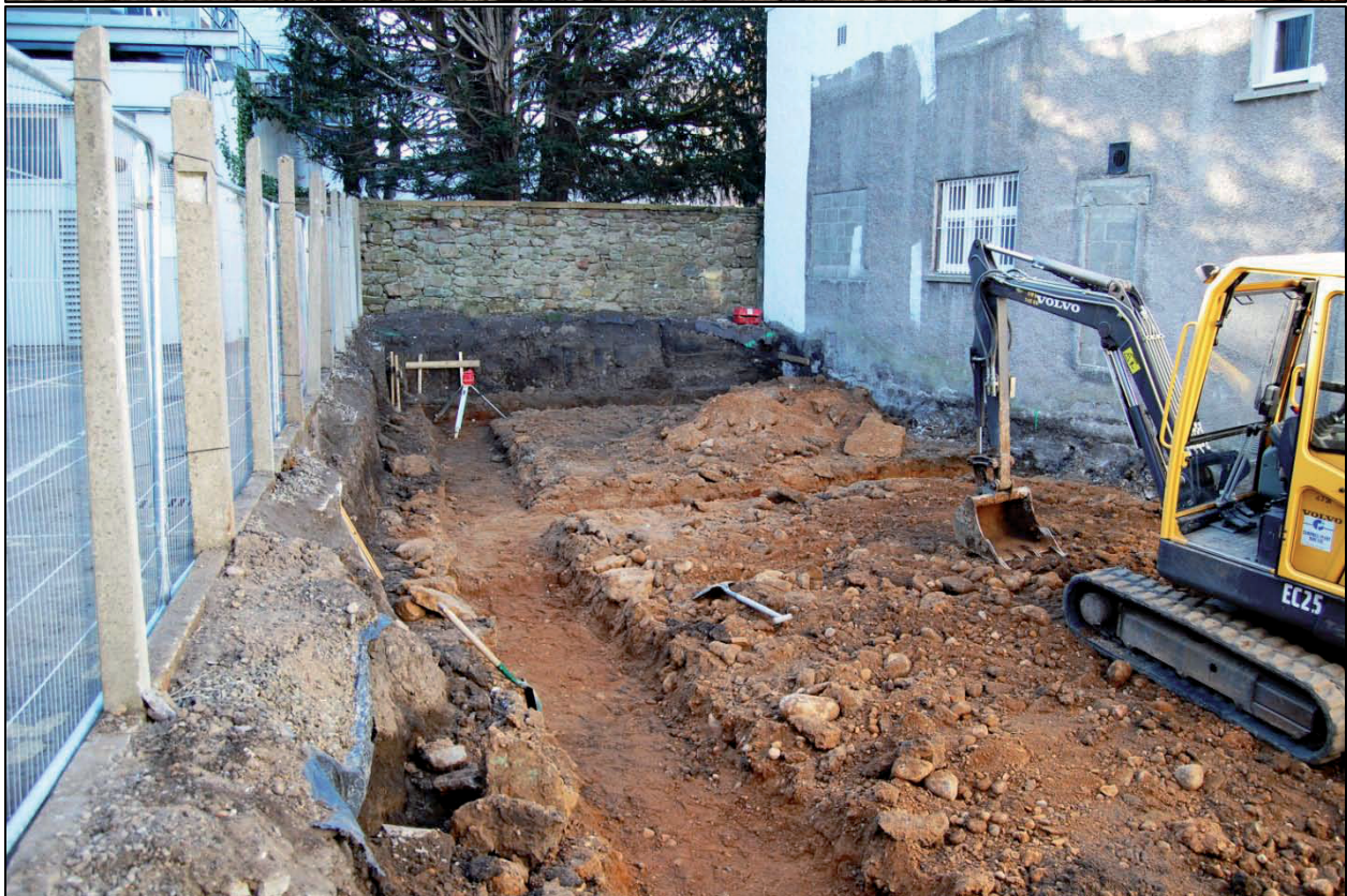
Plate 1 (Top) view NE, site cleared; (Bottom) View SE showing foundation trenches
