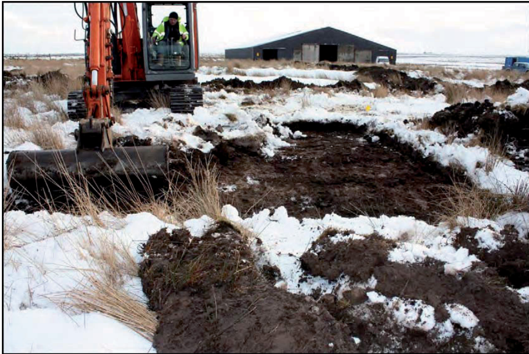
Plate 17 Trial trench T8 being stripped looking SE
