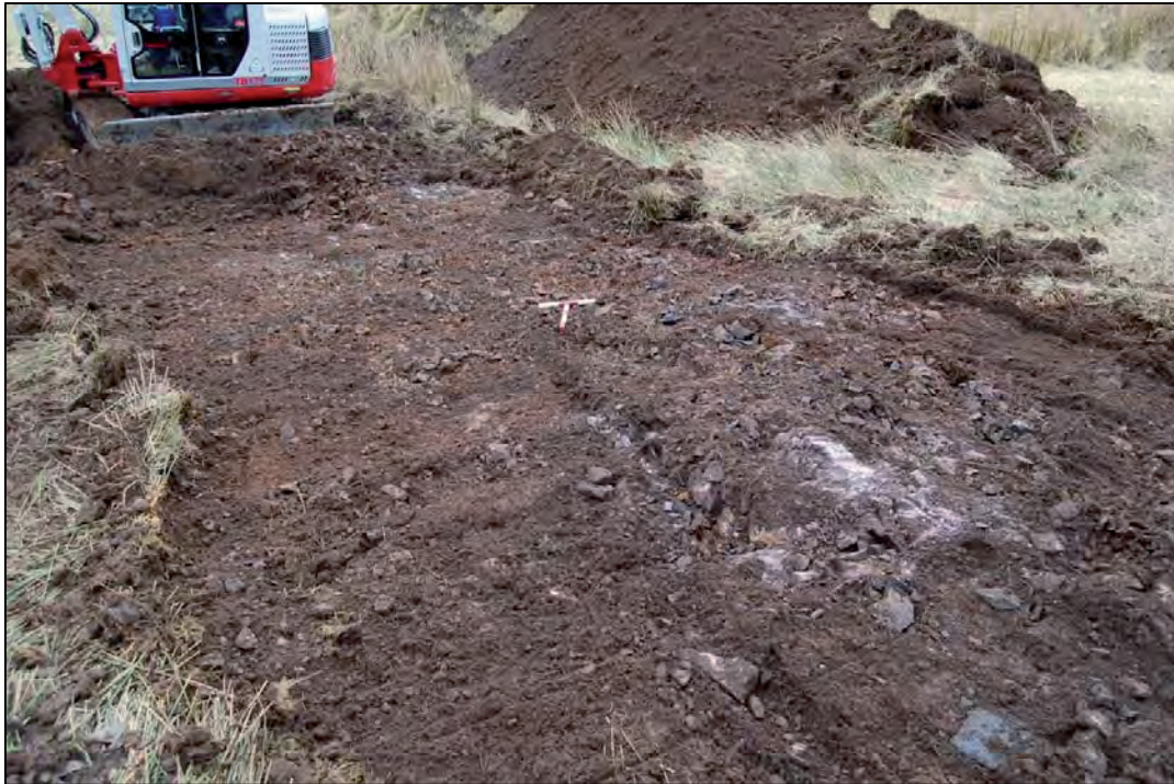
Plate 12 Driveway stripping in progress - bedrock close to surface.
