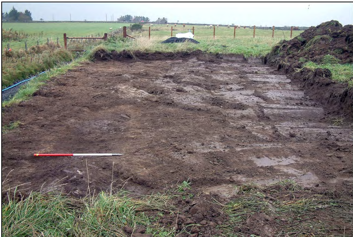
Photo 5 Phase 1 stripped area - looking northwest
