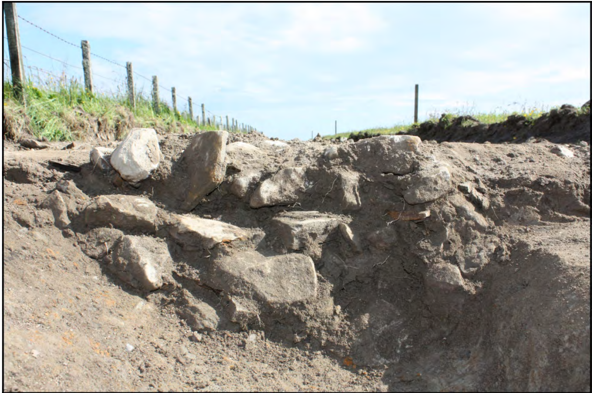
Plate 28 Rumbling drain section 'EE' (figure 7) close-up (scale in 0.5m divisions)
