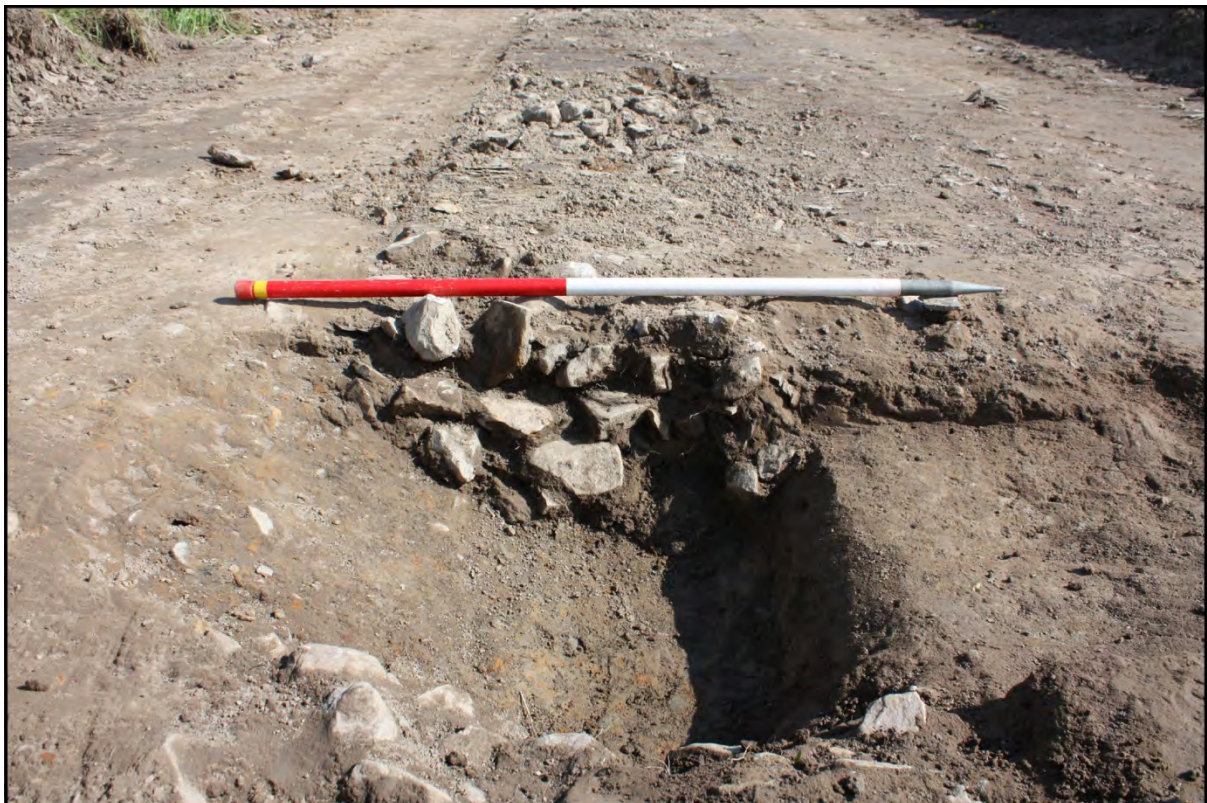
Plate 27 Rumbling drain section 'EE' (figure 7) (2m scale)
