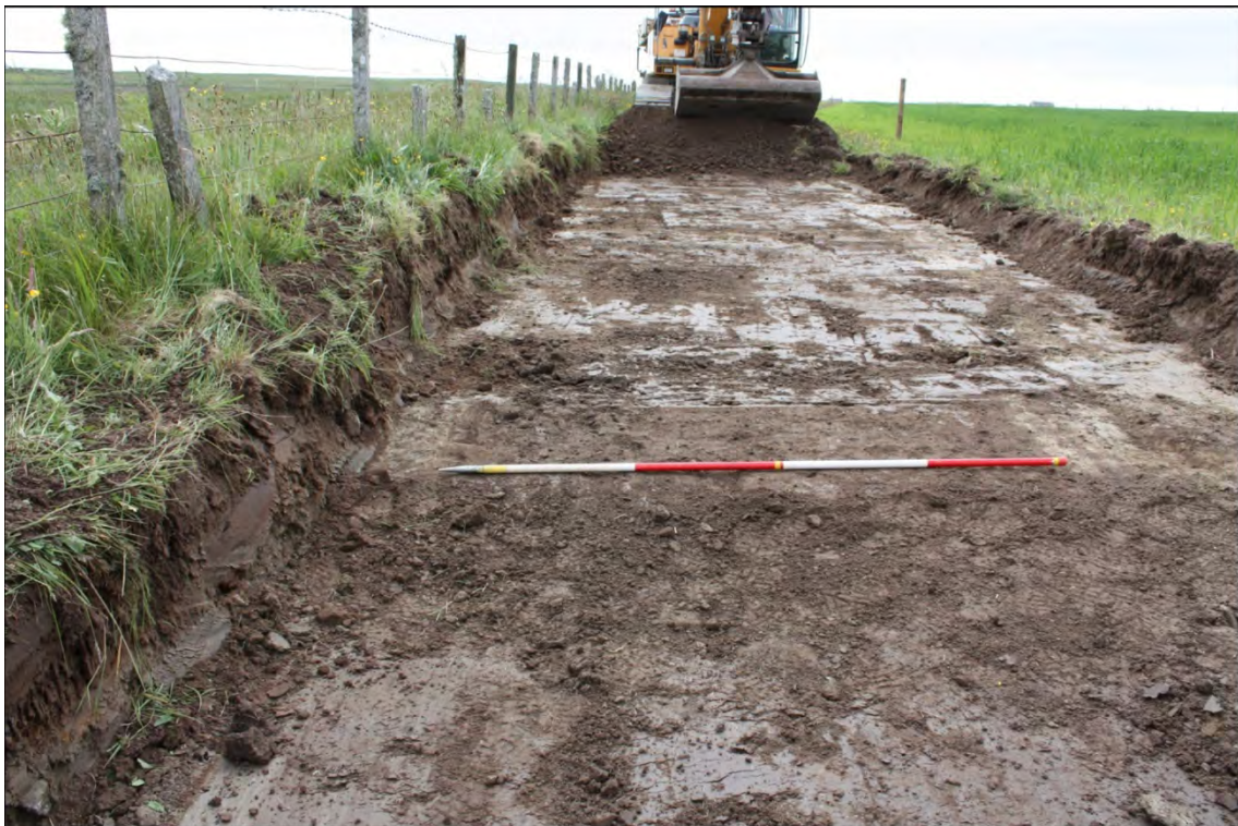
Plate 7 Drive looking south east – ditch cut (2m scale)
