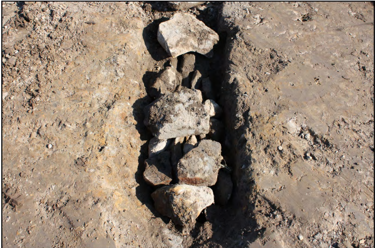
Plate 32 Field drain section 'FF' (figure 8) re-instated
