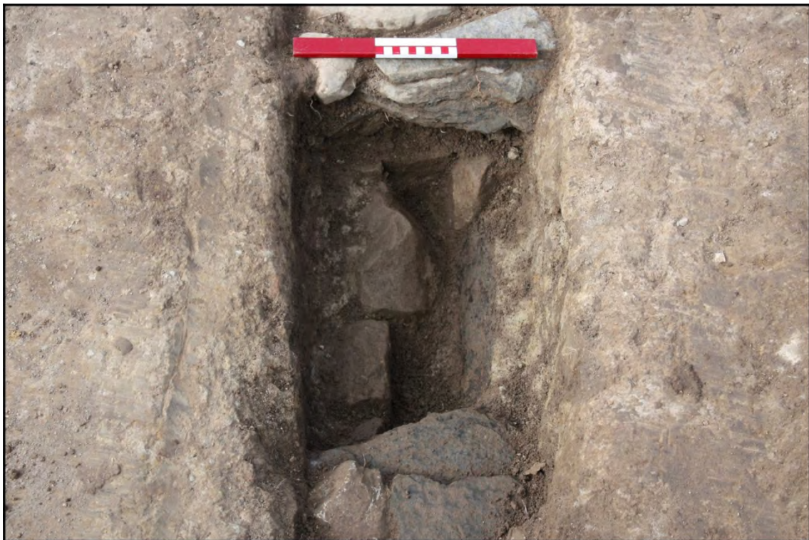
Plate 19 Field drain section 'BB' (figure 8) stage 2 (30cm scale)
