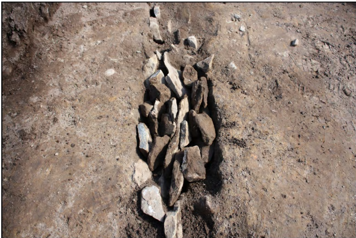
Plate 17 Field drain section 'AA' (Figure 8) re-instated
