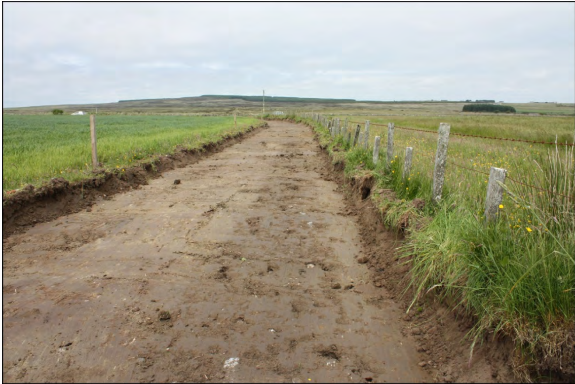
Plate 12 Stripped access drive showing rumbling drain cut
