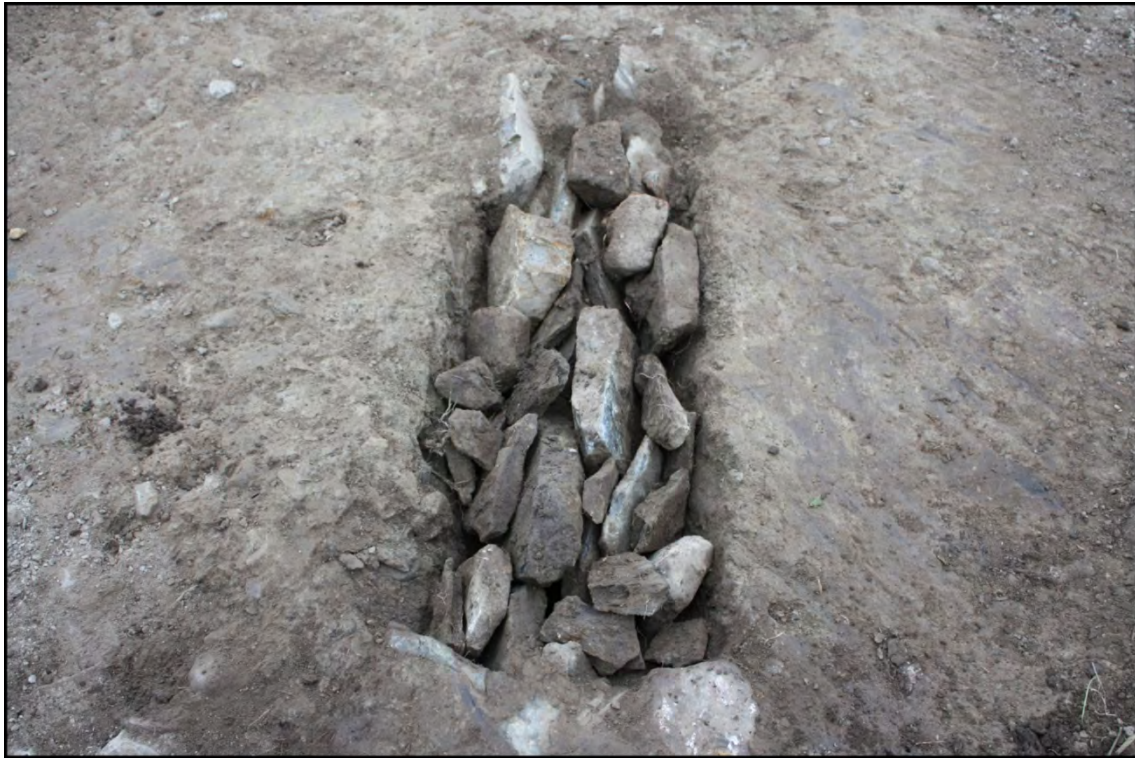
Plate 26 Field drain section 'DD' (figure 8) re-instated
