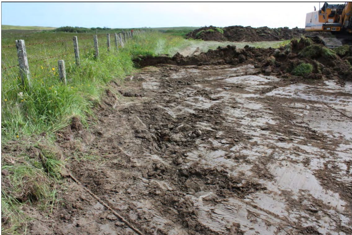
Plate 13 Rumbling drain continuation at hammer-head
