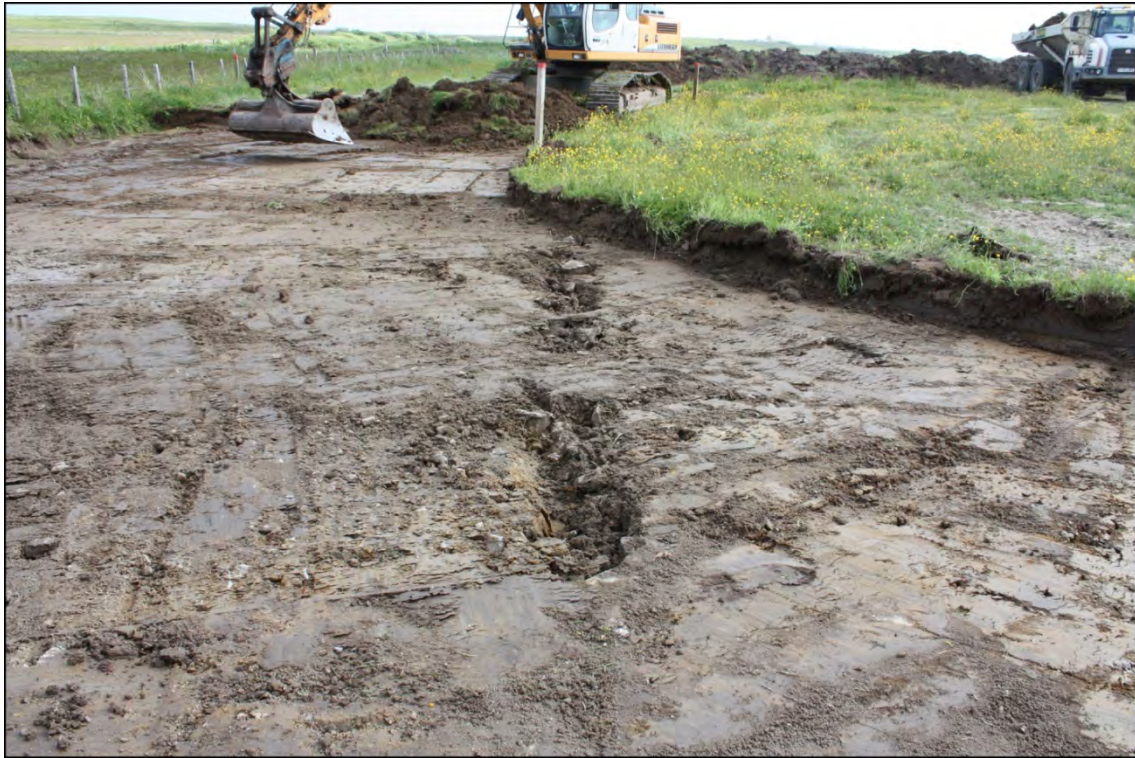
Plate 14 Field drain at hammer-head
