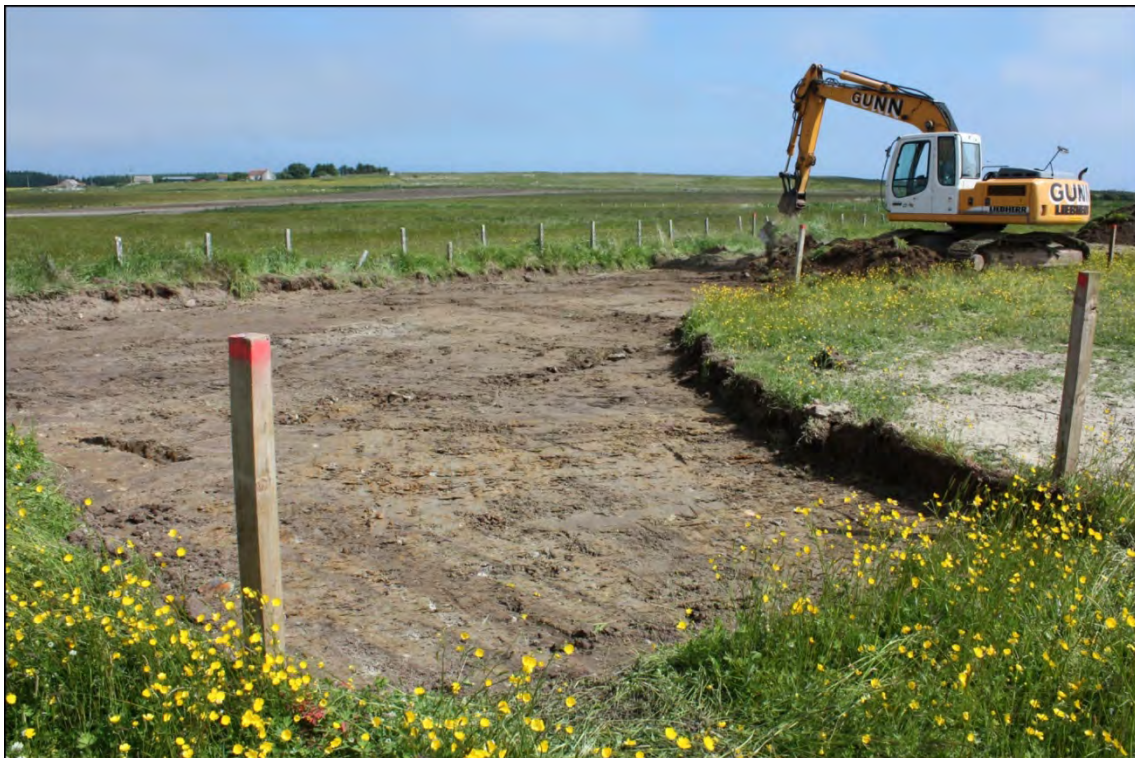
Plate 15 Stripped hammer-head looking east
