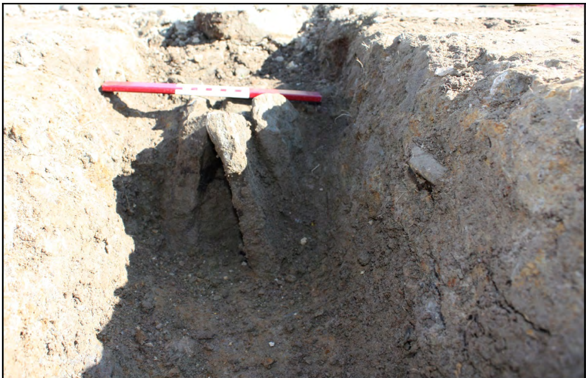
Plate 31 Field drain section 'FF' (figure 8) close-up
