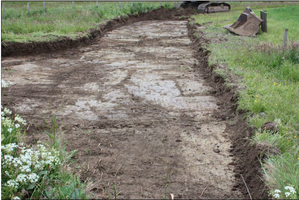
Plate 6 Stripped drive entrance looking east
