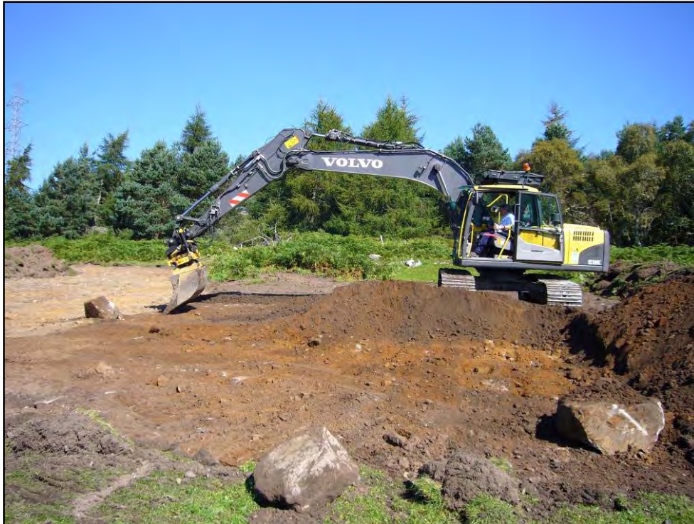
Plate 2 General site clearance showing some of the erratic boulders dislodged.
