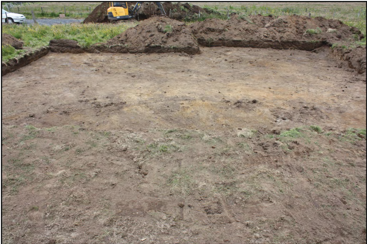
Photo 7 Stripped house-base looking east
