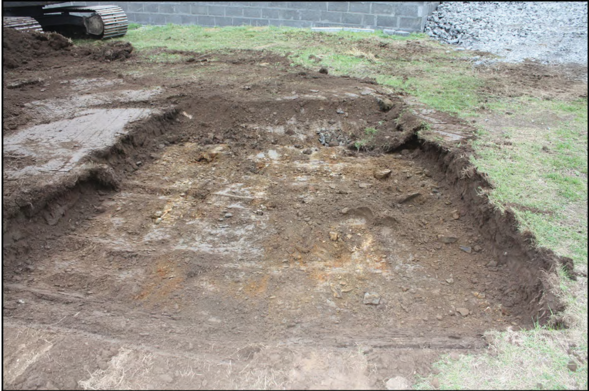
Photo 13 Stripped septic tank location looking northwest
