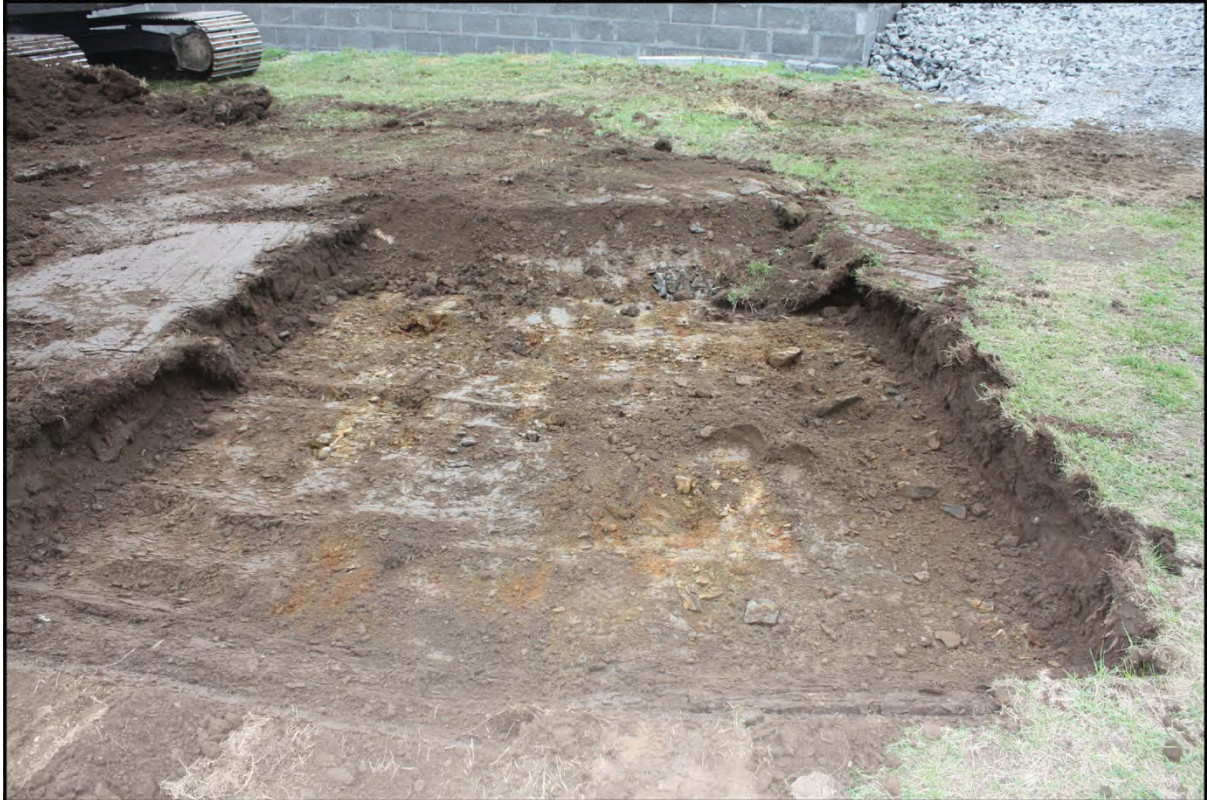
Photo 13 Stripped septic tank location looking northwest
